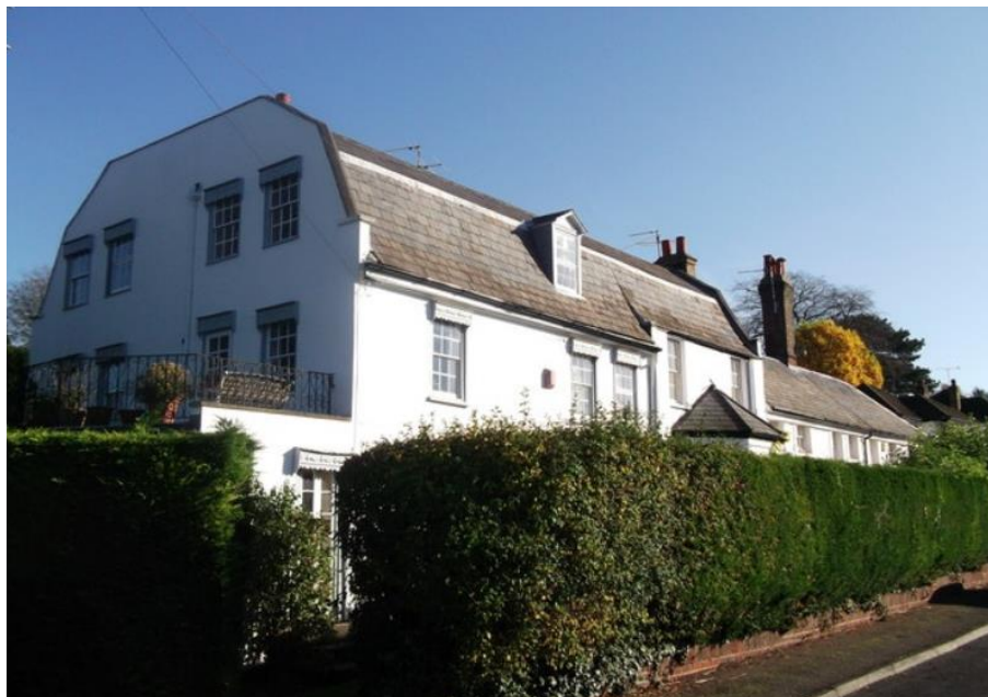
Plate 2: View looking ENE towards the S front of Purley Bury, a Grade II listed house
