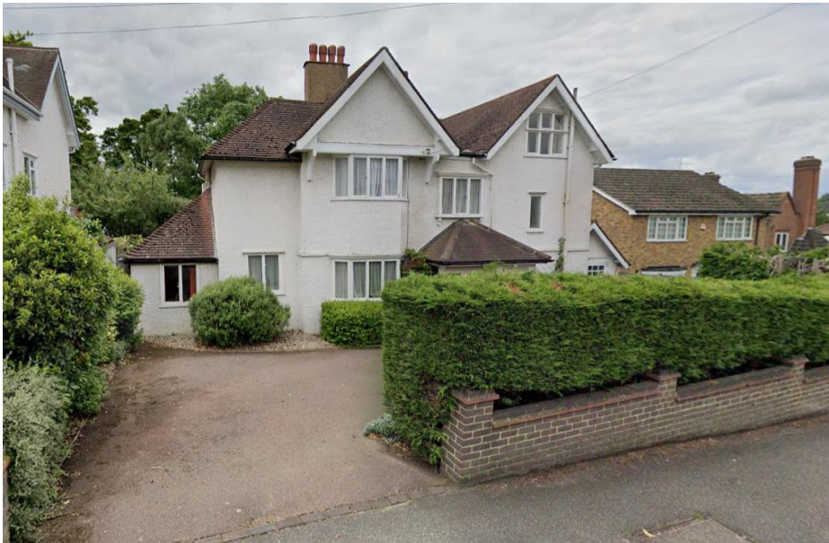
Plate 1: View looking SW showing front elevation of 84 Purley Downs Road
