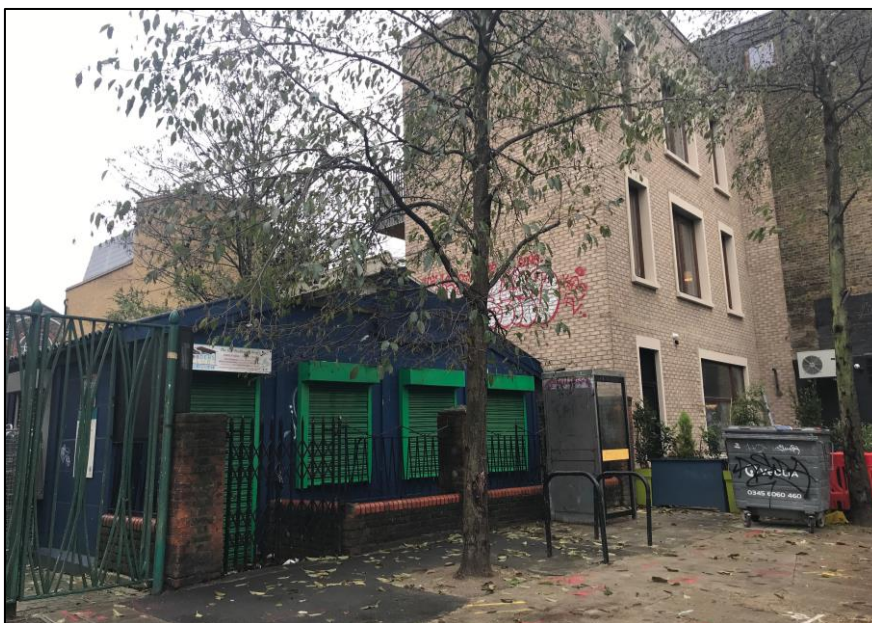
Plate 3: View looking ESE from Peckham Hill Street towards the front of the old library building
