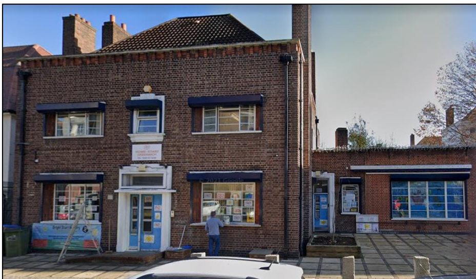
Plate 1: View looking E showing main elevation of Oak House and single storey extension to S
