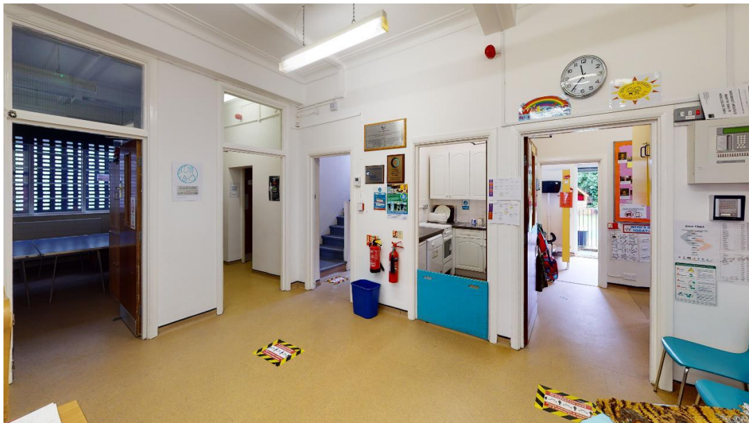
Plate 6: Internal view looking NW showing communal area on ground floor with doorway leading to stairs to first floor
