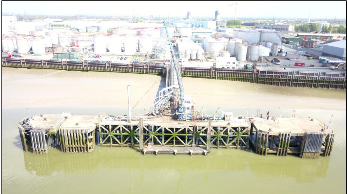
Plate 3: View looking N from river showing front elevation of Thunderer Jetty with oil storage facilities on landward side
