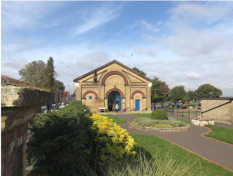
Plate 8: View looking W showing E gable end of workshop range to SW of main engine house at Crossness Pumping Station
