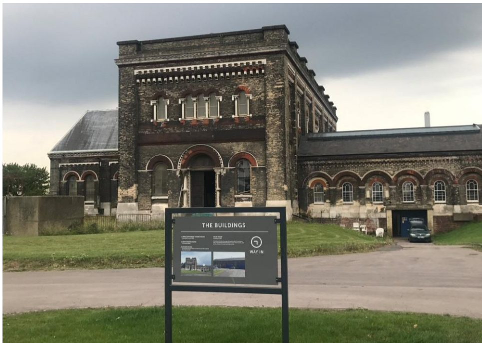
Plate 7: View looking ENE showing eastern elevation of engine house at Crossness Pumping Station
