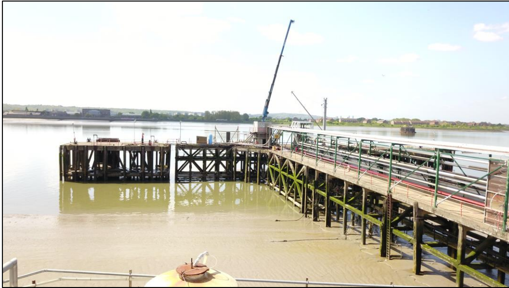
Plate 2: Oblique view looking SSW showing approach structure leading to head/platform at Thunderer Jetty
