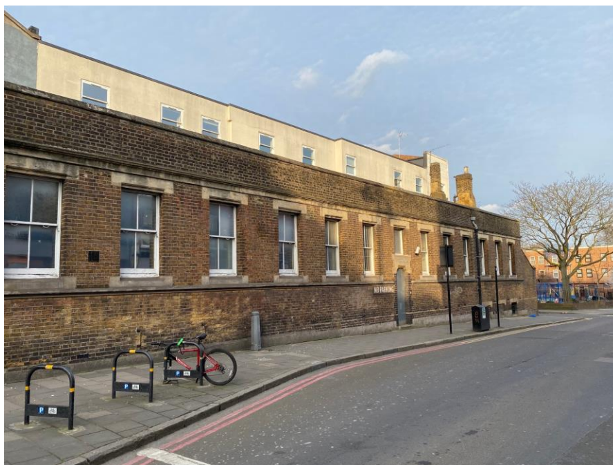
Plate 5: View looking ENE showing frontage of No. 138 Stoke Newington High Street running along Brooke Road
