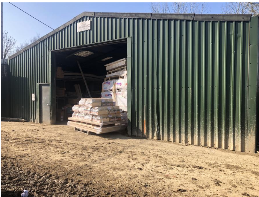
Plate 4: View WSW showing exterior of late 20 th century steel-framed shed (Building 1)
