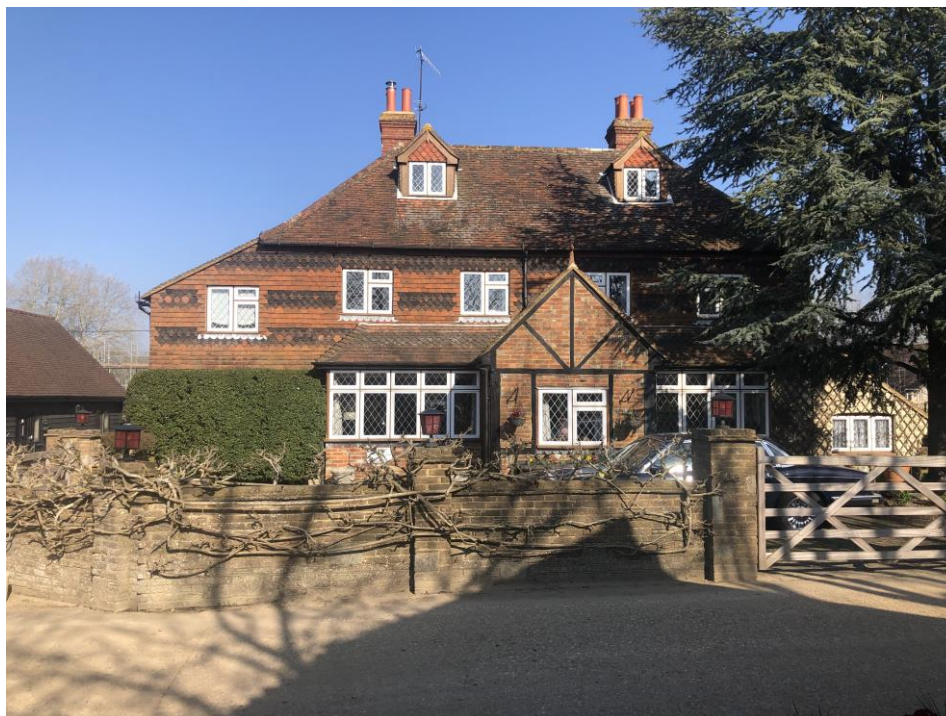
Plate 1: View N showing principal S-facing elevation of farmhouse at Nutley Dean Farm (to the S of the site)
