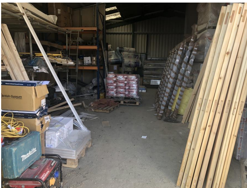
Plate 5: View looking W showing interior of late 20 th century steel-framed storage shed (Building 1)
