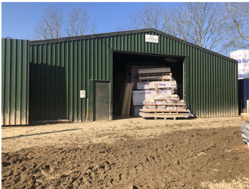
Plate 3: View WNW showing principal E-facing elevation of late 20 th century steel-framed storage shed (Building 1)
