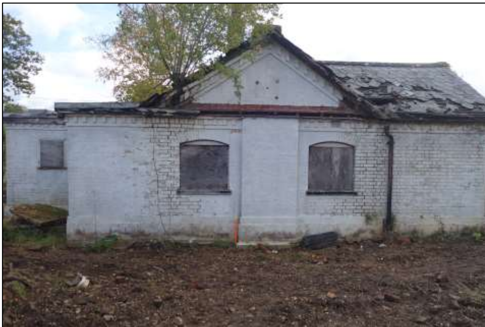
Plate 4: View looking SE showing NW-facing elevation of The Lodge
