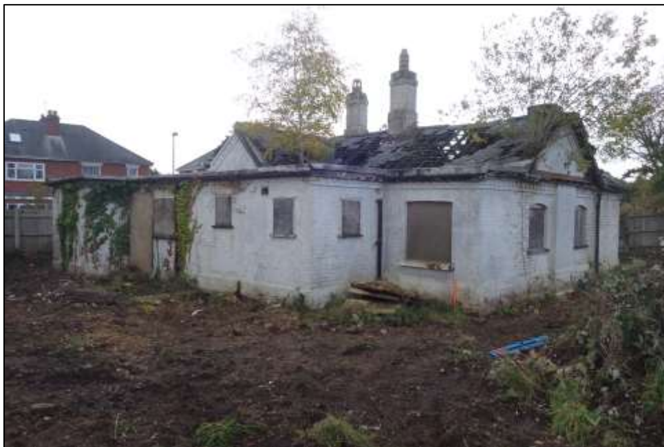
Plate 6: View looking S showing NE-facing elevation of The Lodge
