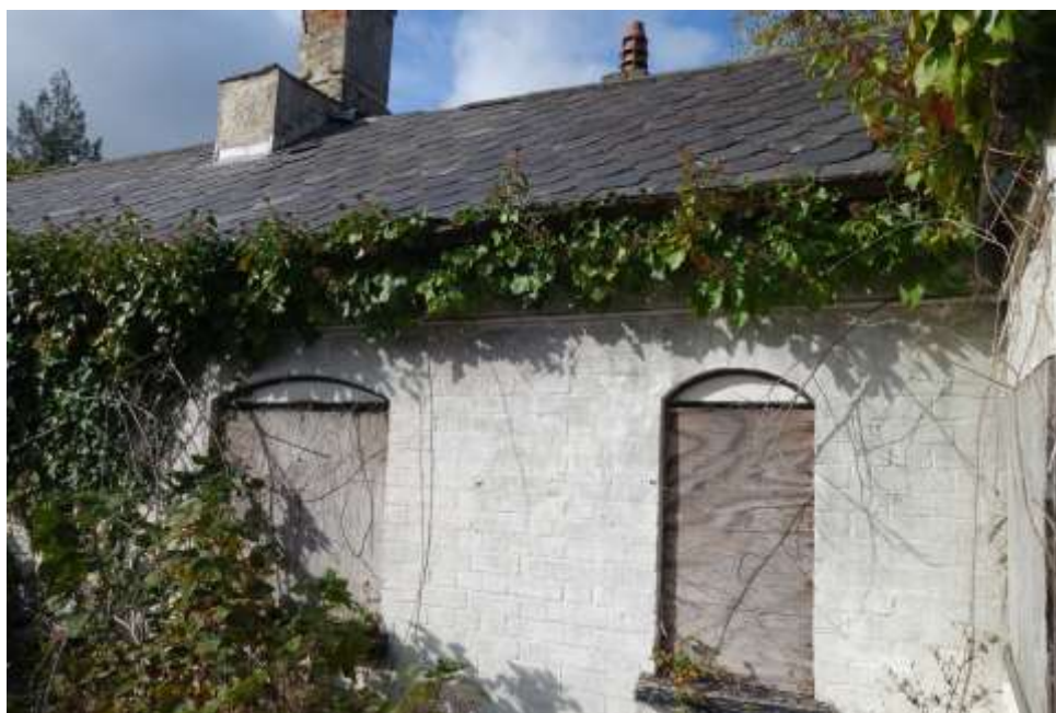
Plate 8: View looking W showing segmental and round arched windows in SE-facing elevation
