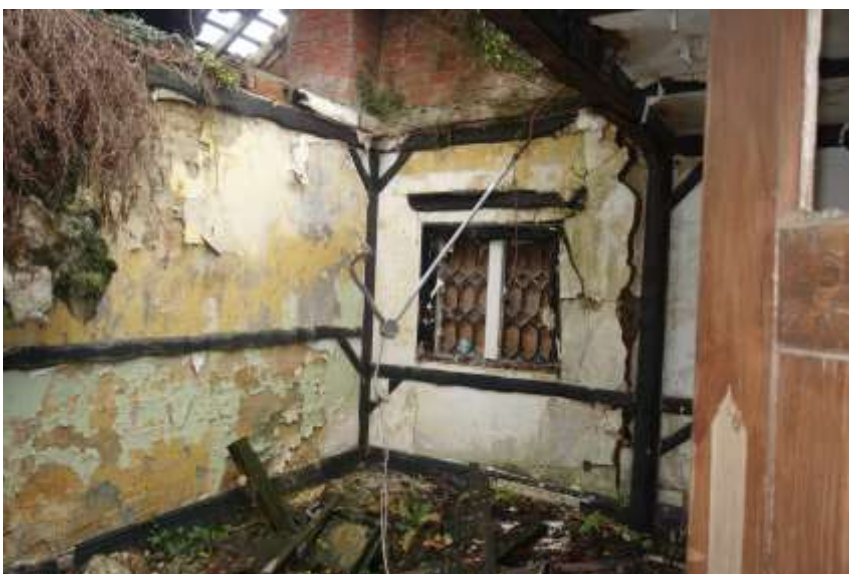
Plate 11: Interior view of NW room showing casement window in NW wall
