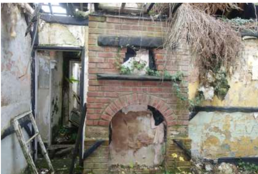
Plate 10: Interior view of NW room looking SW showing modern brick fireplace
