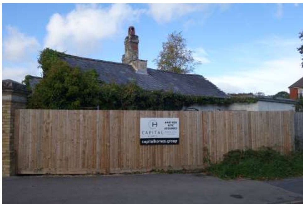
Plate 9: View looking NW showing SE facing elevation from Brook Lane
