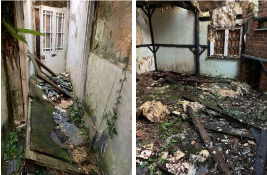
Plate 14: View looking SW along cross-axial hallway towards main entrance
