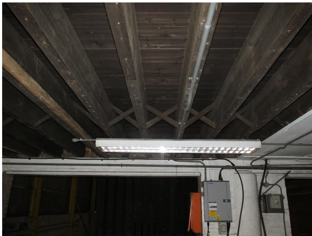
Plate 54: Internal view looking S within the central range
