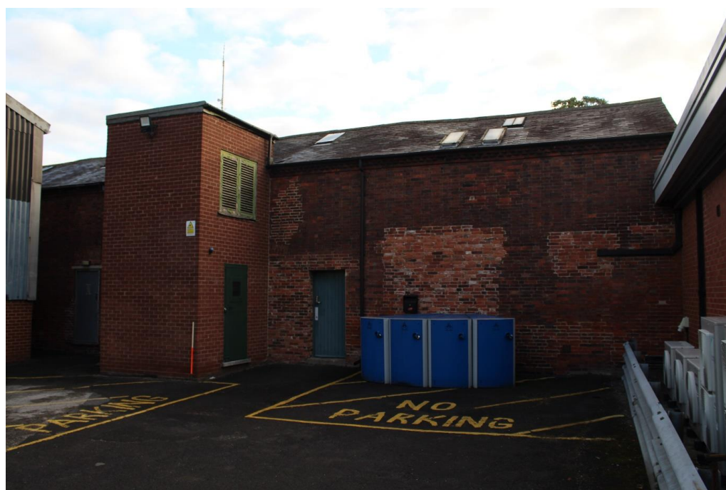
Plate 18: External view looking ENE towards the west-facing elevation of the E wing
