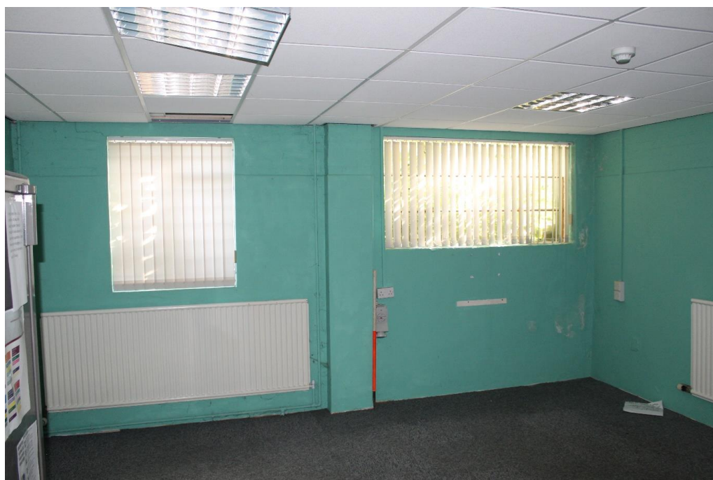
Plate 67: Internal view looking ESE within the E wing
