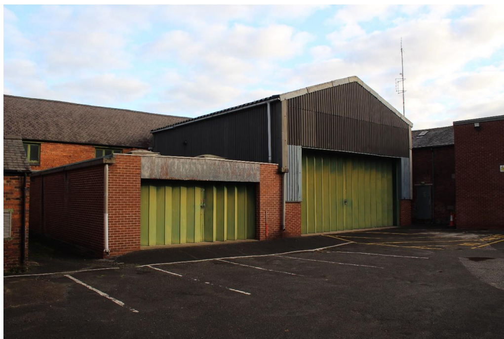
Plate 15: External view looking NE of the south-facing elevation of the central range
