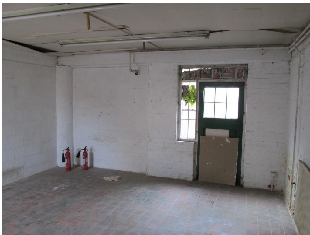
Plate 49: Internal view looking S within the central range
