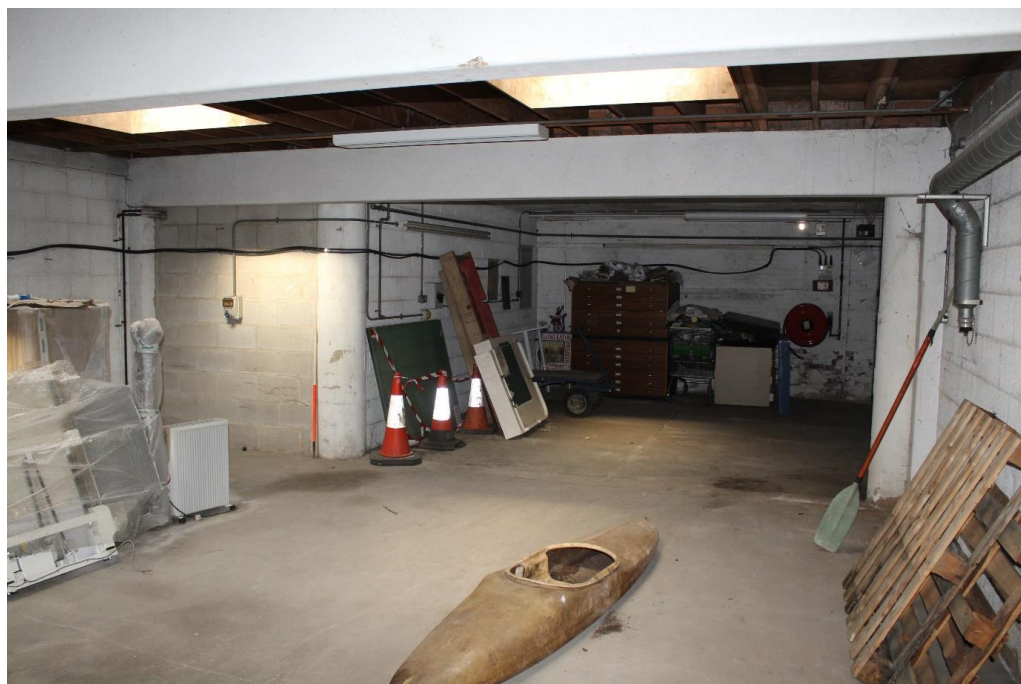
Plate 56: Internal view looking NNW within the westernmost modern workshop
