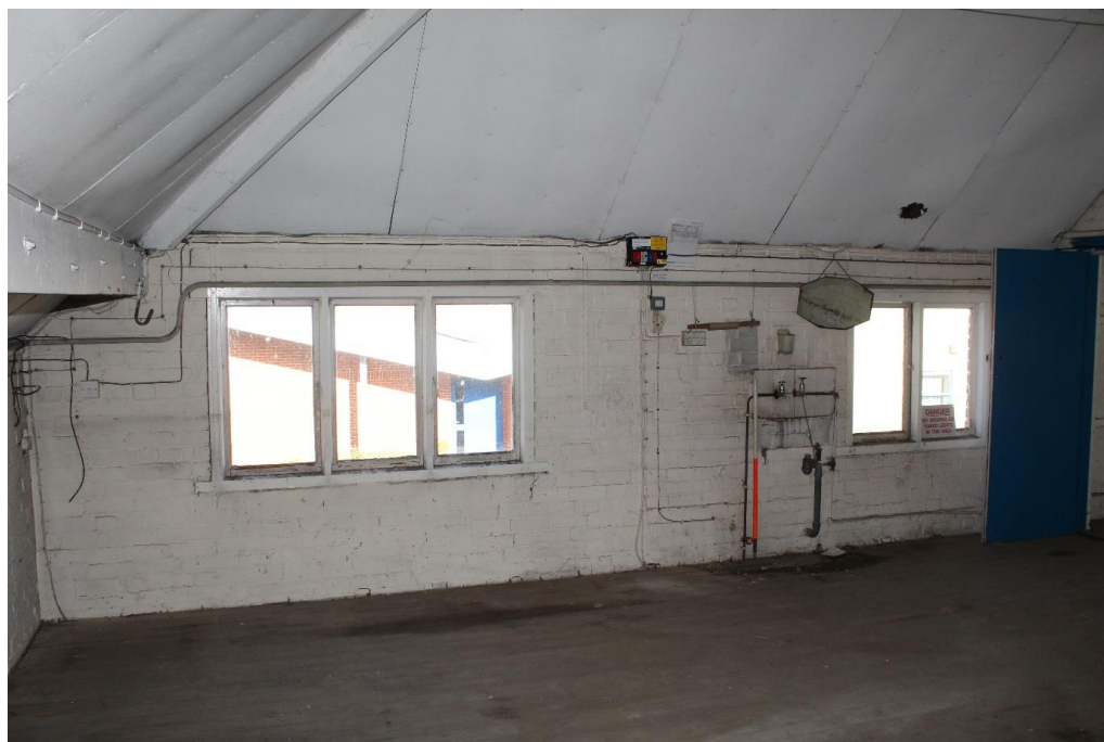
Plate 89: Internal view looking NNE within first floor of the central range
