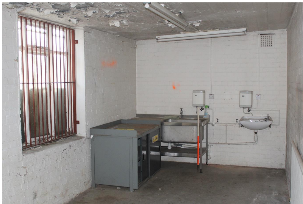
Plate 72: Internal view looking SW within the modern wash room
