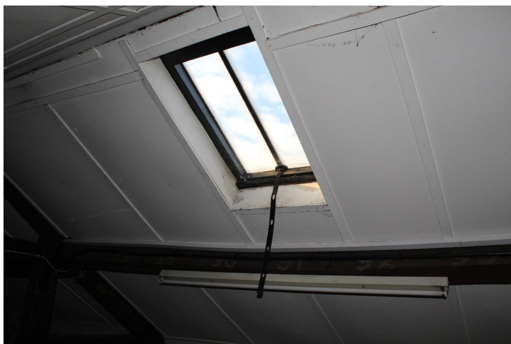
Plate 94: Internal view looking SW within the attic of the E wing
