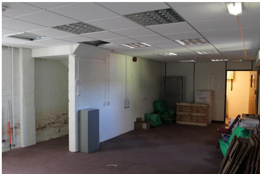
Plate 65: Internal view looking SE within the E wing
