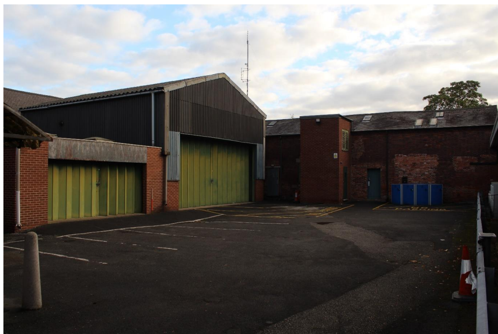
Plate 2: External view looking ENE
