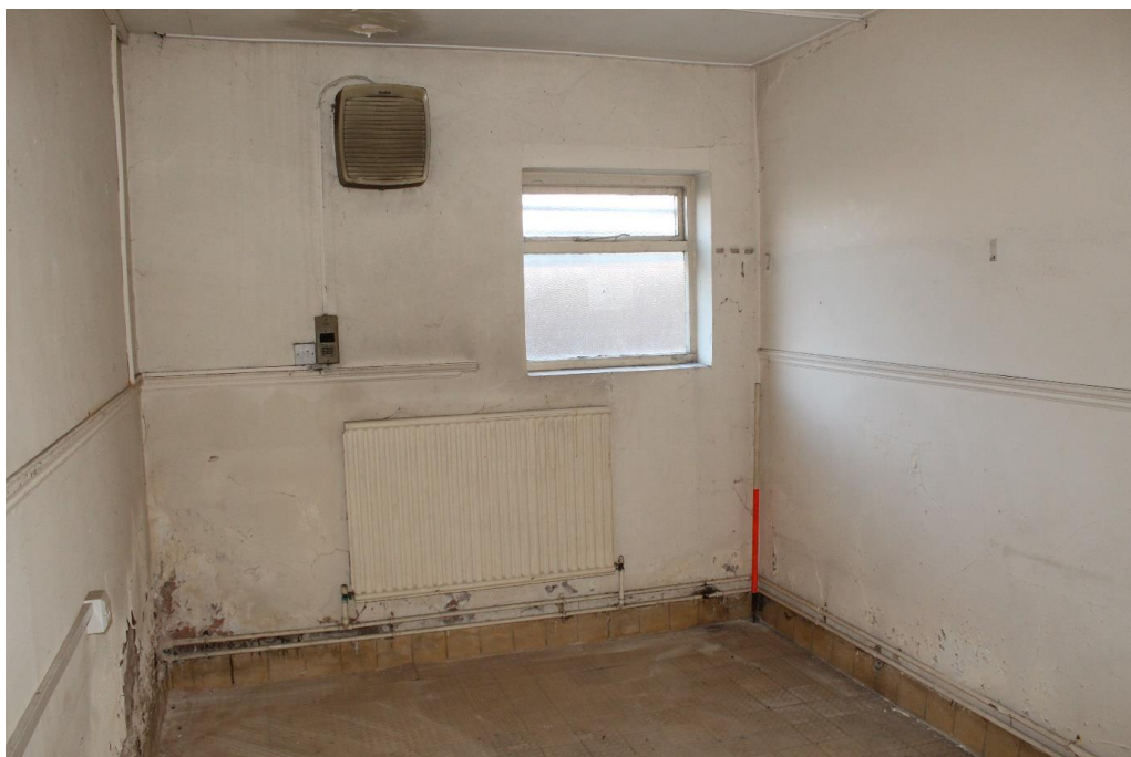
Plate 43: Internal view looking NNE within the central range
