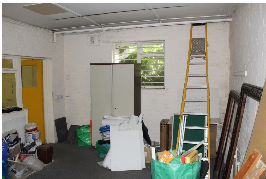
Plate 69: Internal view looking ENE within the E wing
