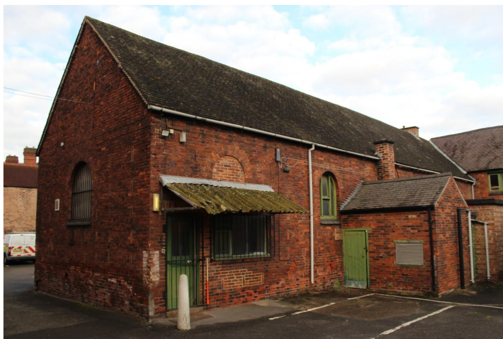
Plate 6: External view looking NW showing the south and east-facing elevations of the W wing
