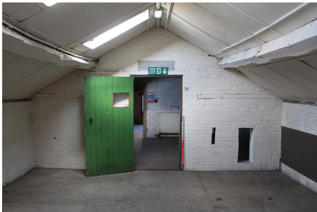
Plate 97: Internal view looking N within the attic of the E wing
