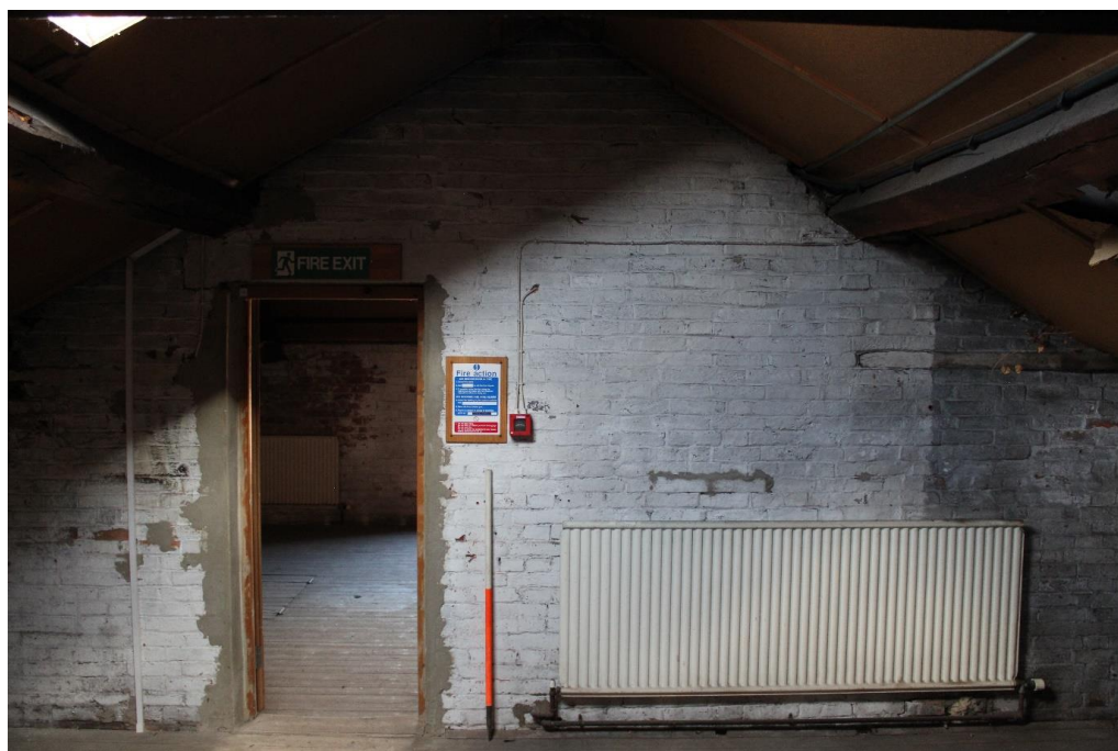
Plate 100: Internal view looking N within the attic of the E wing
