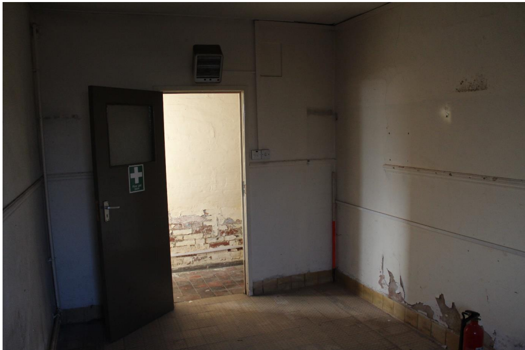
Plate 44: Internal view looking SSW within the central range
