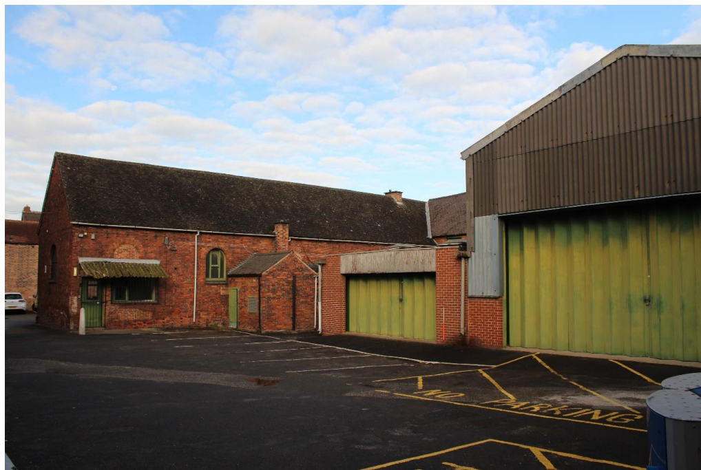
Plate 1: External view looking NW
