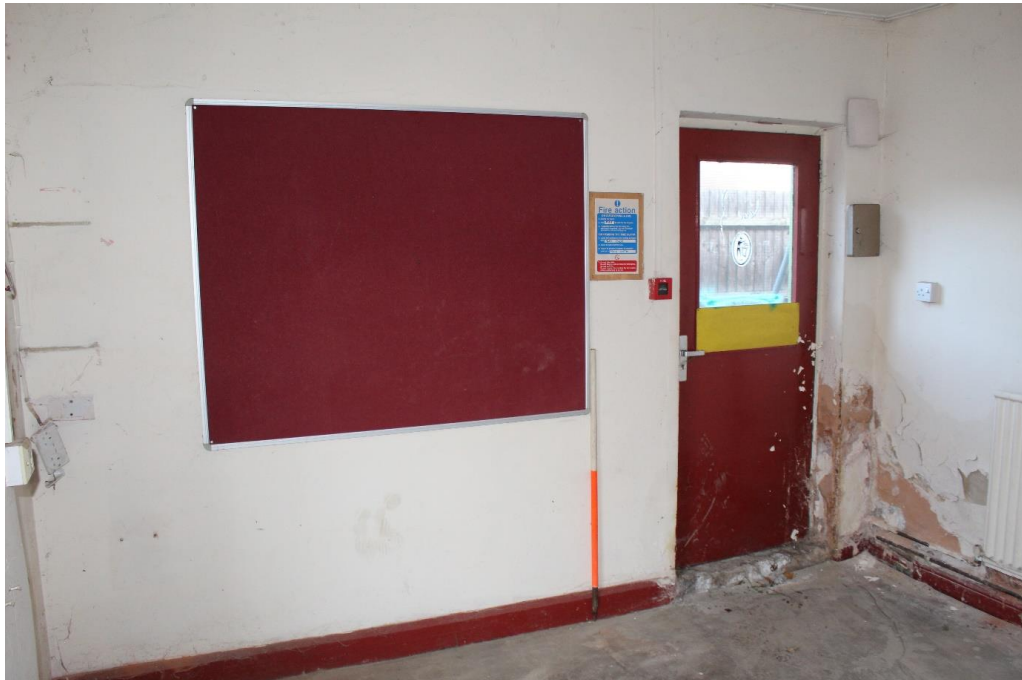
Plate 47: Internal view looking NNE within the central range
