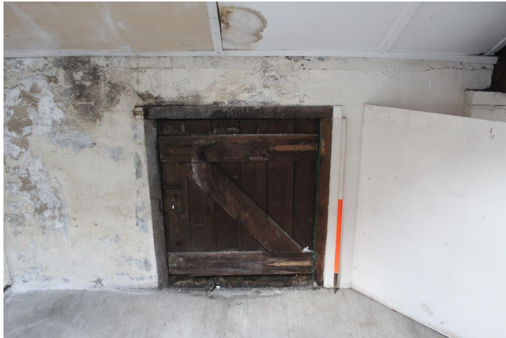
Plate 96: Internal view looking W within the attic of the E wing
