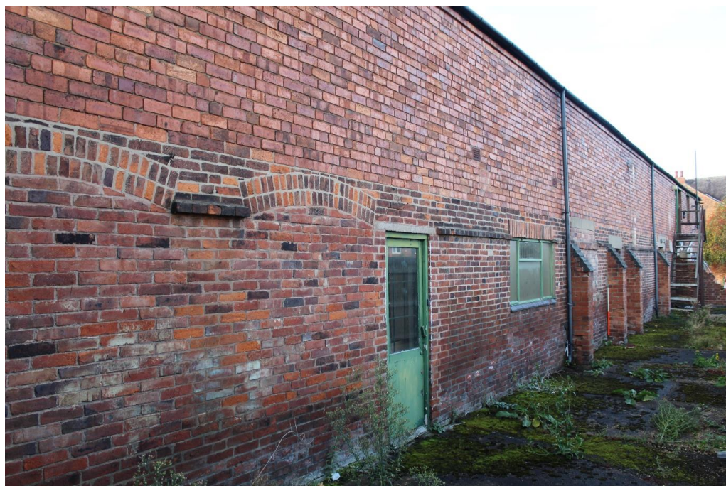
Plate 14: External view WSW of the north-facing elevation of the central range
