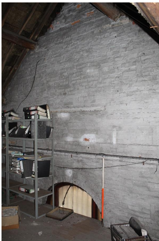
Plate 29: Internal view looking SE within the mezzanine floor within the W wing
