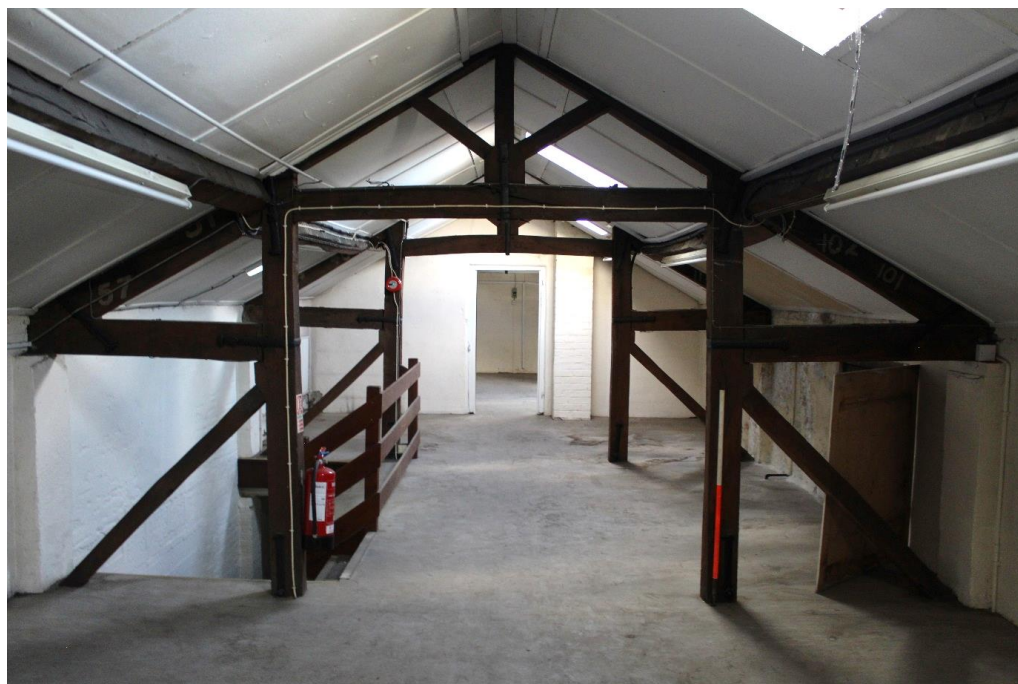
Plate 93: Internal view looking S within the attic of the E wing
