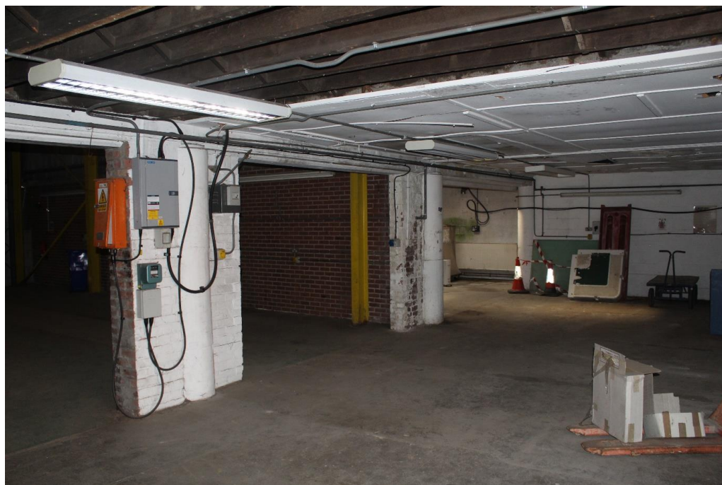
Plate 51: Internal view looking SW within the central compartment
