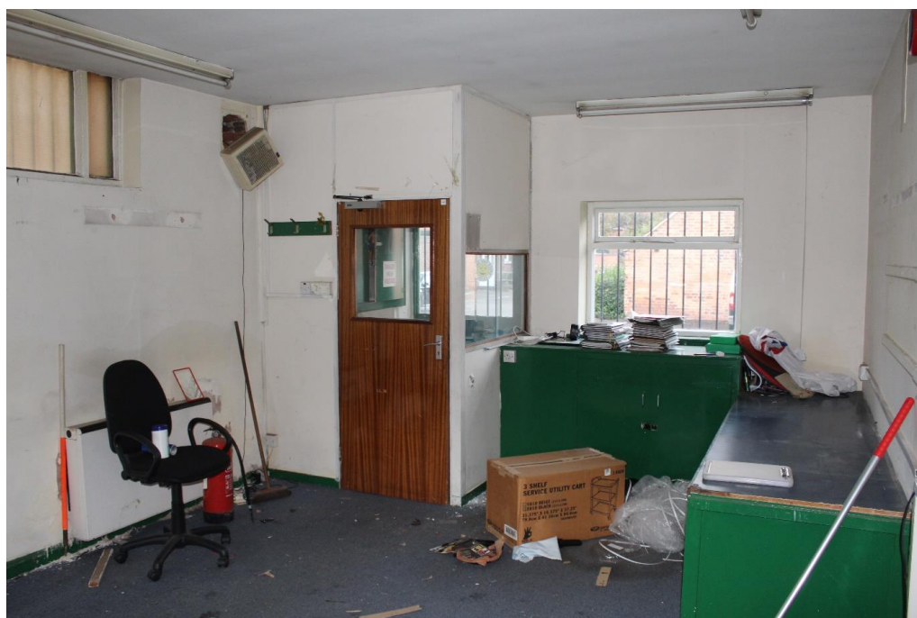
Plate 26: Internal shot looking WSW within the southernmost bay of the W wing
