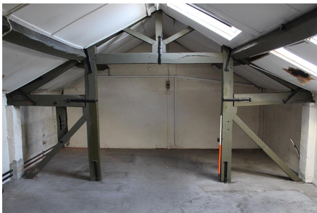
Plate 92: Internal view looking S within the attic of the E wing
