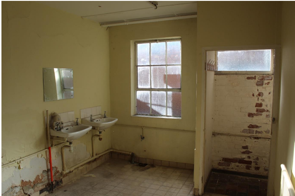
Plate 45: Internal view looking SSE within the central range
