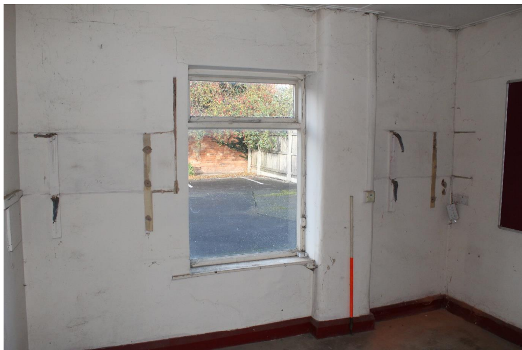
Plate 48: Internal view looking WNW within the central range
