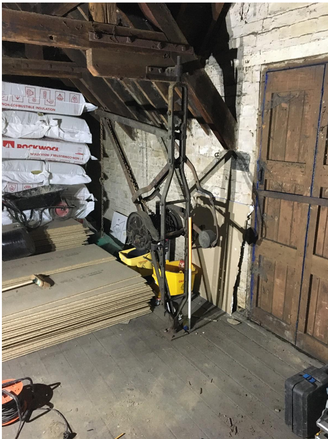
Plate 29: View SW showing detail of winch structure attached to tie beam
