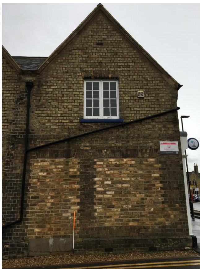
Plate 5: View E showing southernmost bay of W-facing elevation with blocked doorway and window
