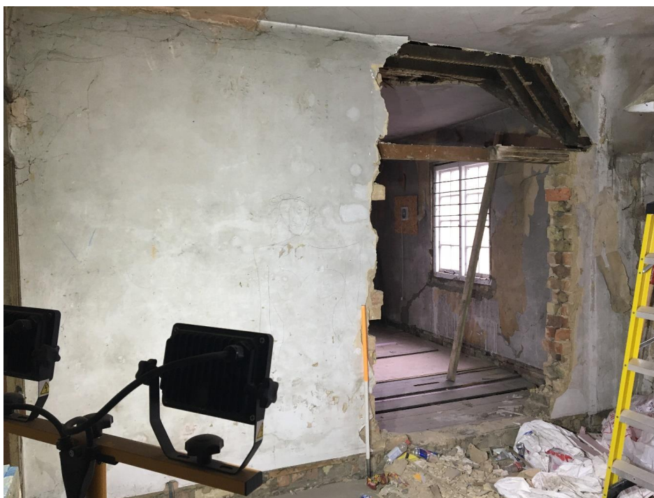
Plate 37: View showing S wall of compartment with evidence of covered ceiling (and exposed joists)
