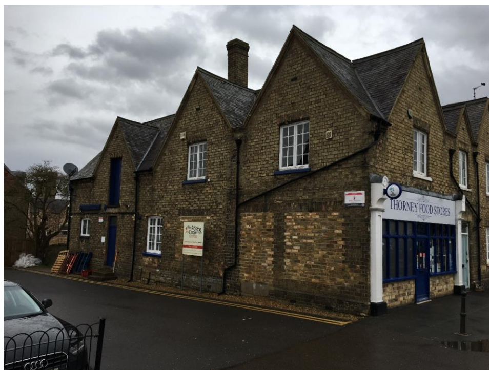
Plate 3: Oblique view NE showing W-facing elevation of No. 4 Wisbech Road
