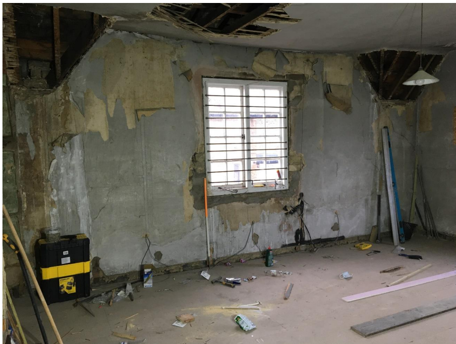
Plate 44: General view of southernmost room on first floor looking SE
