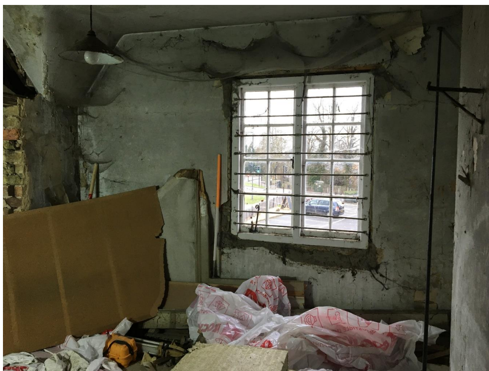
Plate 36: View W showing casement window in W wall of room to S of main compartment
