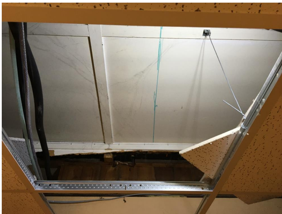
Plate 20: View S showing exposed older ceiling panels concealed by modern plasterboard
