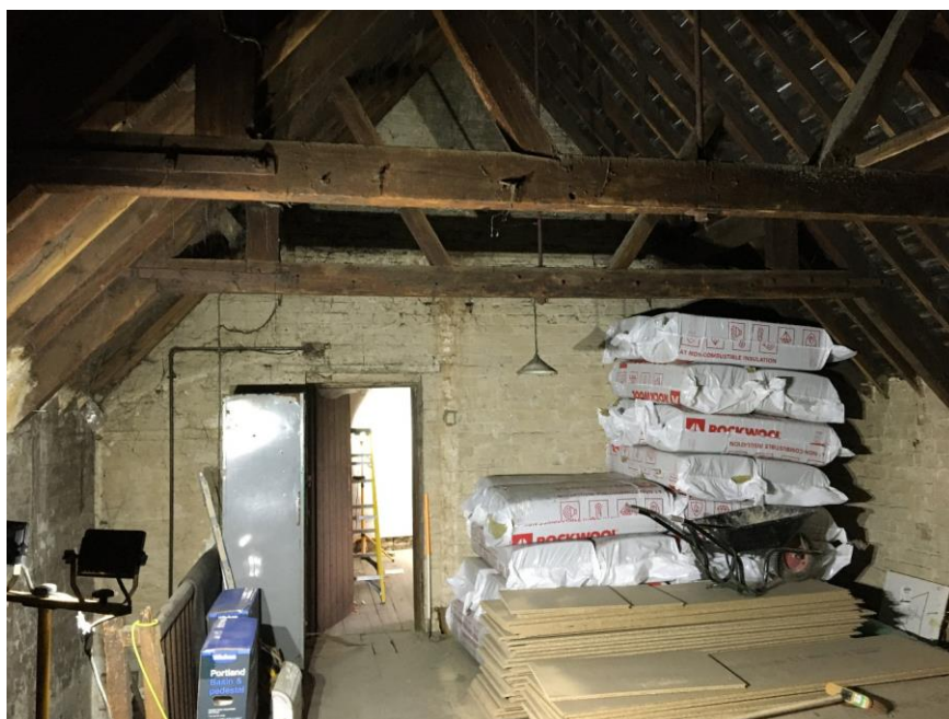
Plate 25: View SSE showing interior of southernmost bay of main compartment
