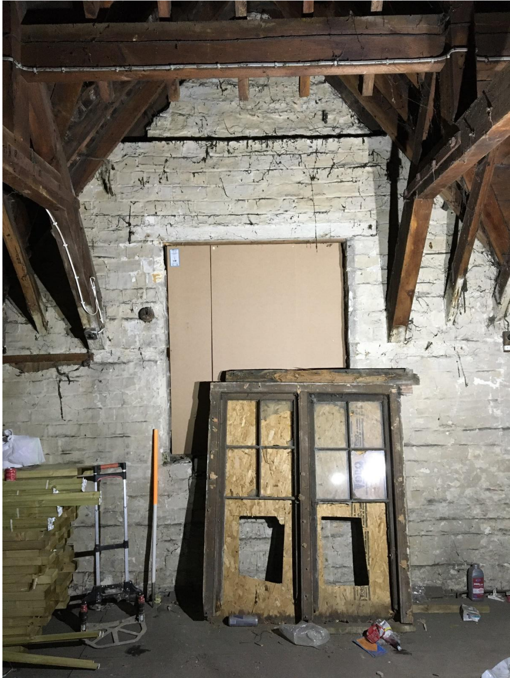
Plate 32: View looking E showing E wall of central bay with blocked opening and frame of original casement window beneath
