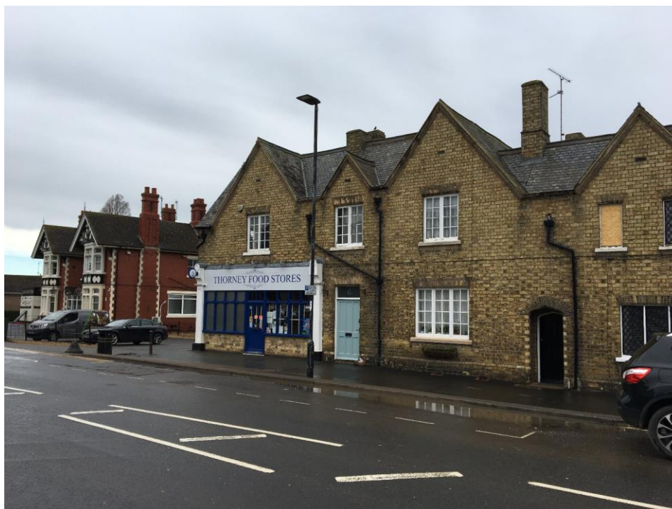
Plate 1: General view NW showing exterior of No. 4 Wisbech Road (currently occupied by Thorney Food Stores)
