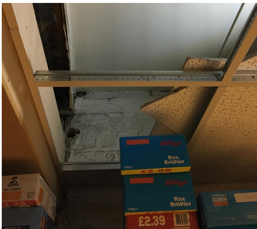
Plate 21: View W showing exposed ceiling beams concealed by modern plasterboard panels
