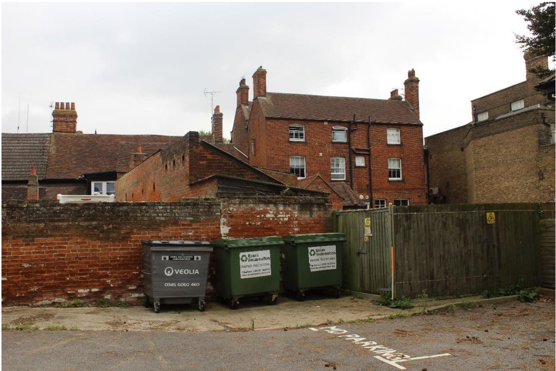
Plate 5: External view ESE of W-facing elevation
