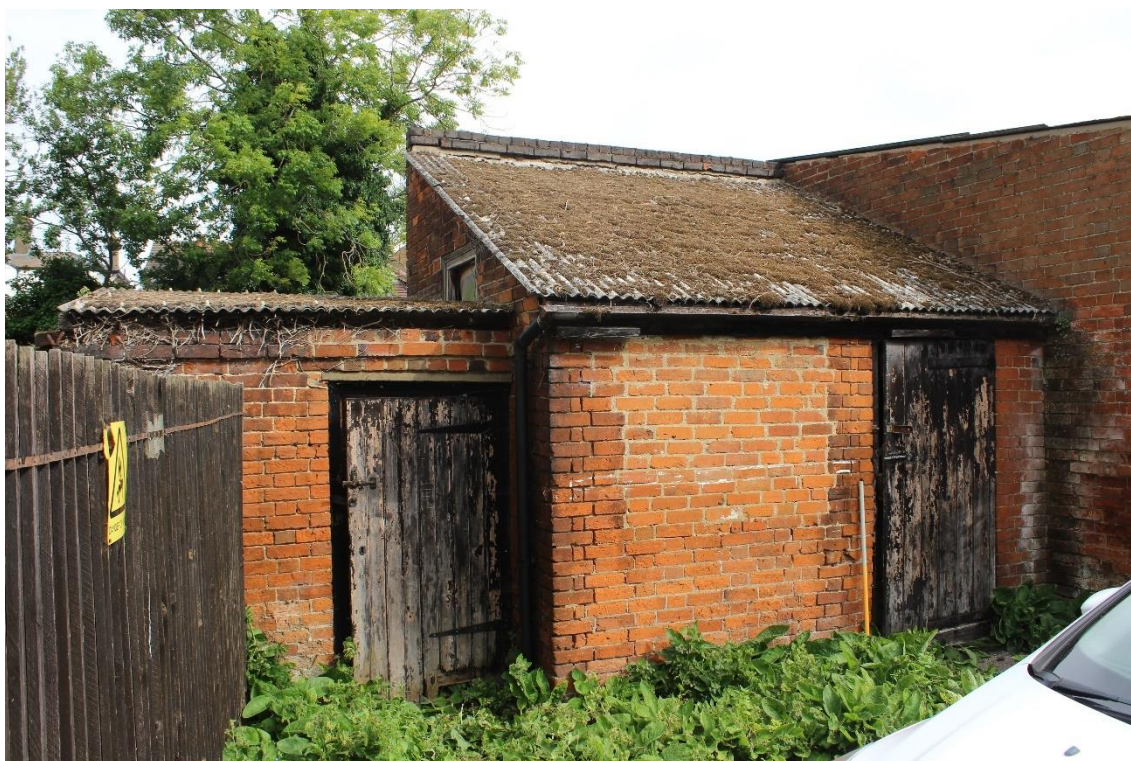
Plate 3: External oblique view NNE of adjoining storerooms – S-facing elevation
