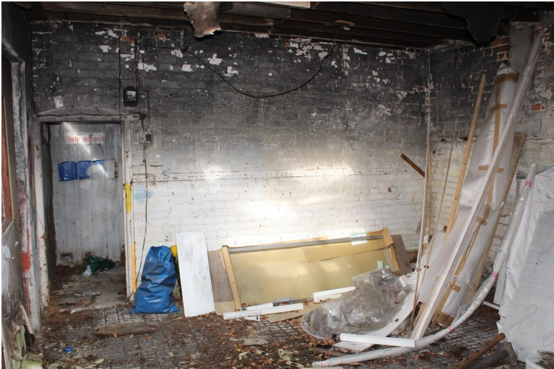
Plate 16: Internal view NW of office compartment
