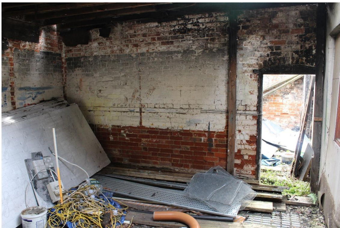
Plate 14: Internal view ENE of office compartment
