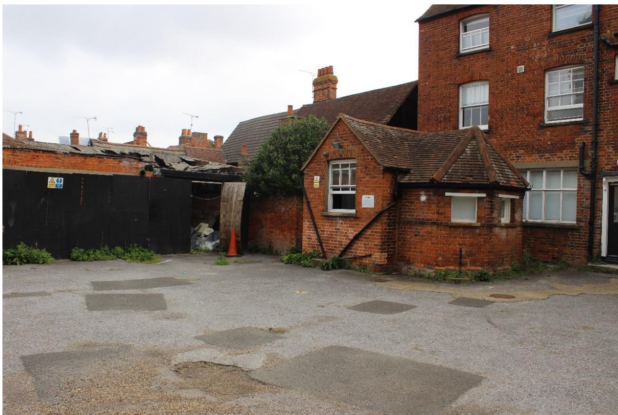
Plate 1: External view NE showing rear of No.22 South Street (right) and outbuilding (left)
