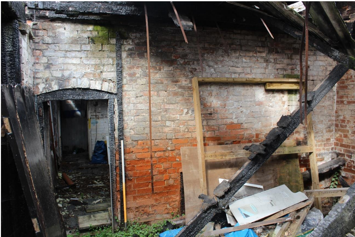
Plate 11: Internal view W of garage compartment
