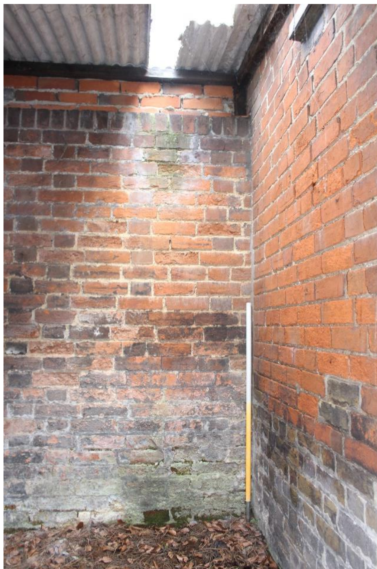
Plate 26: Internal view WNW of storage room
