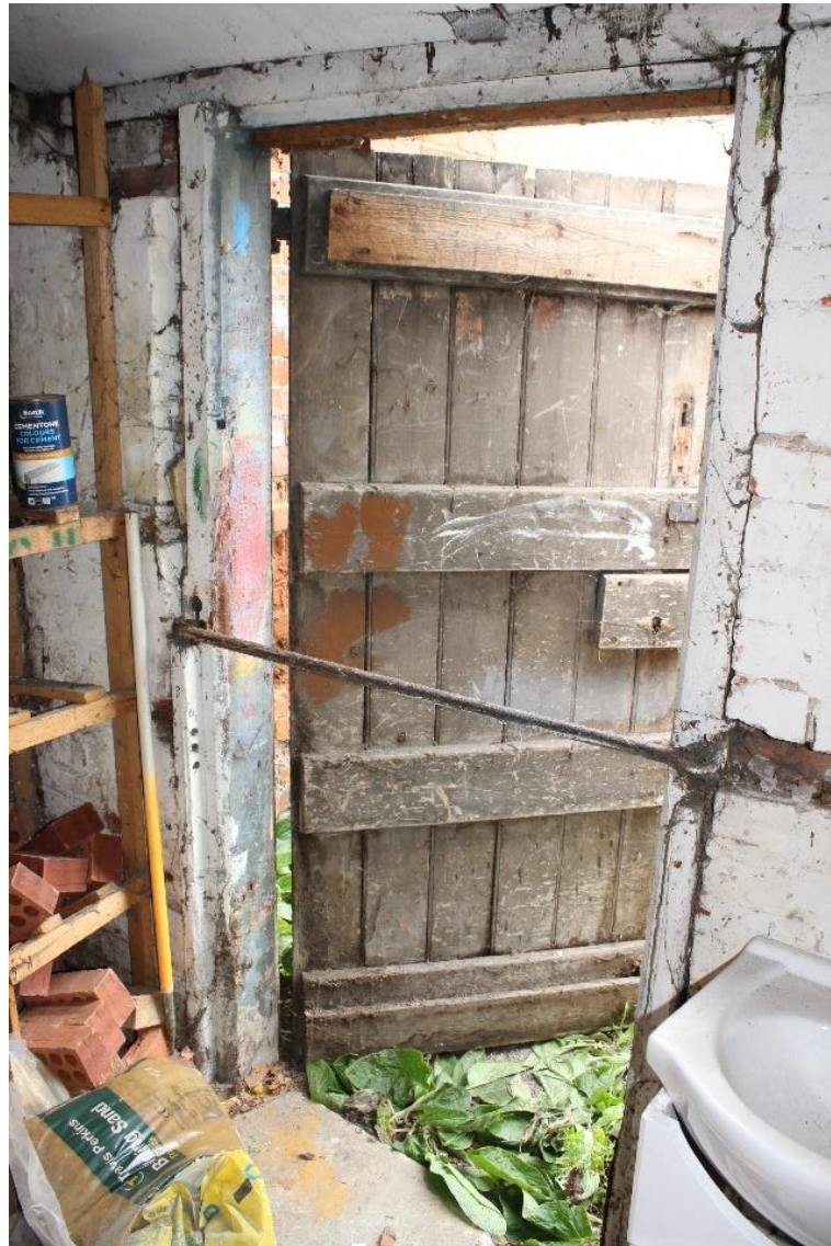
Plate 25: Internal view ESE of the kick-bar in the doorway of storage room
