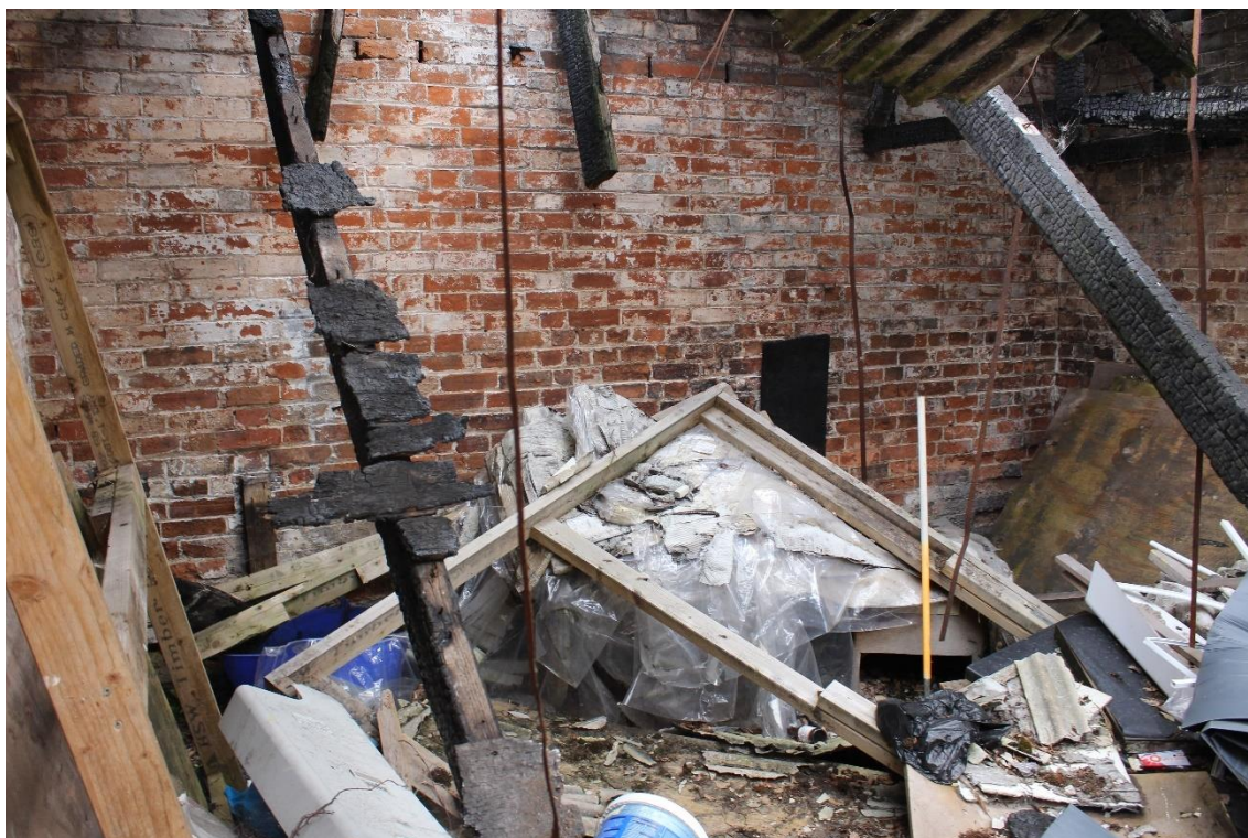
Plate 8: Internal view N of garage compartment
