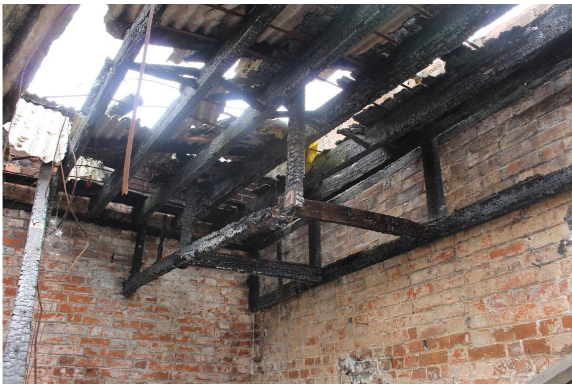
Plate 12: Internal view NE of storage feature within garage compartment
