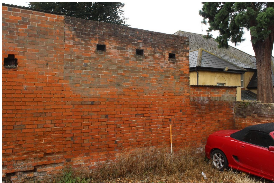
Plate 7: External oblique view SSW of storeroom extensions – N-facing elevation
