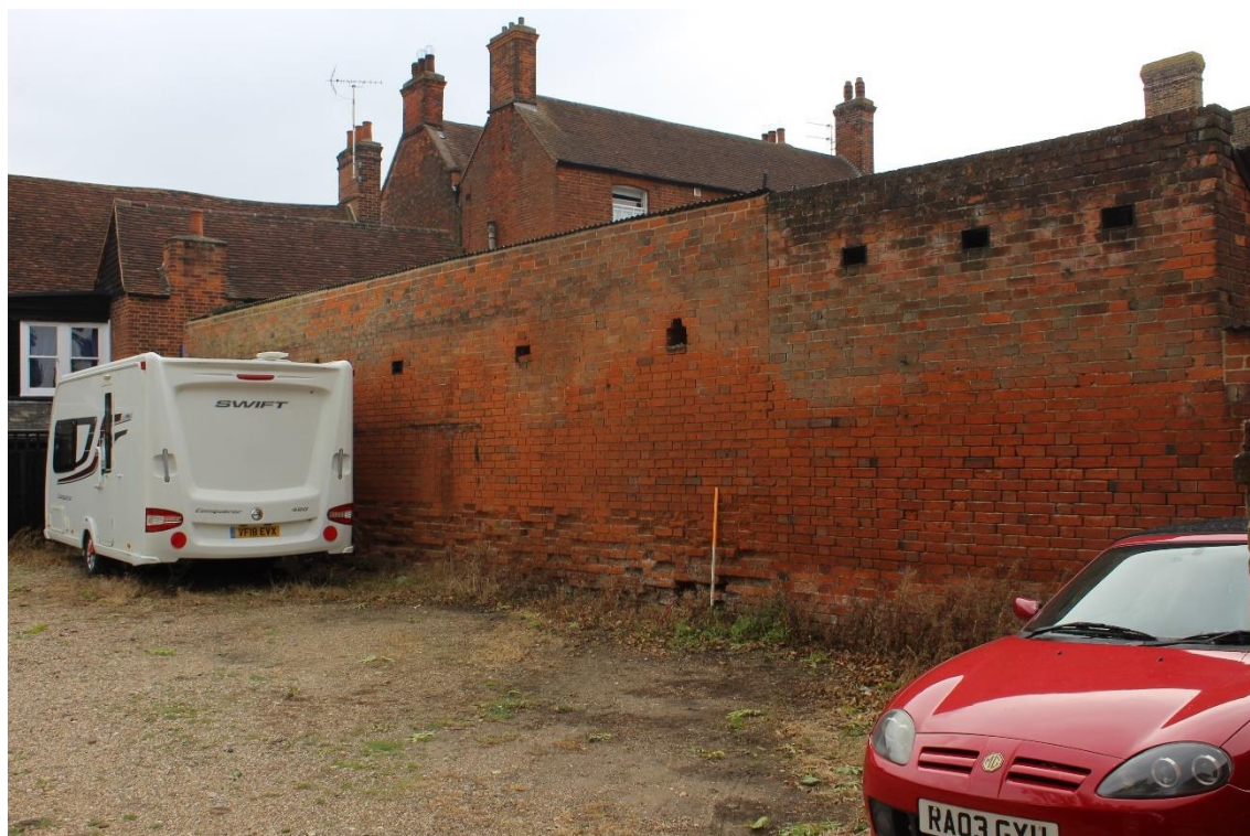
Plate 6: External oblique view SE of N-facing elevation
