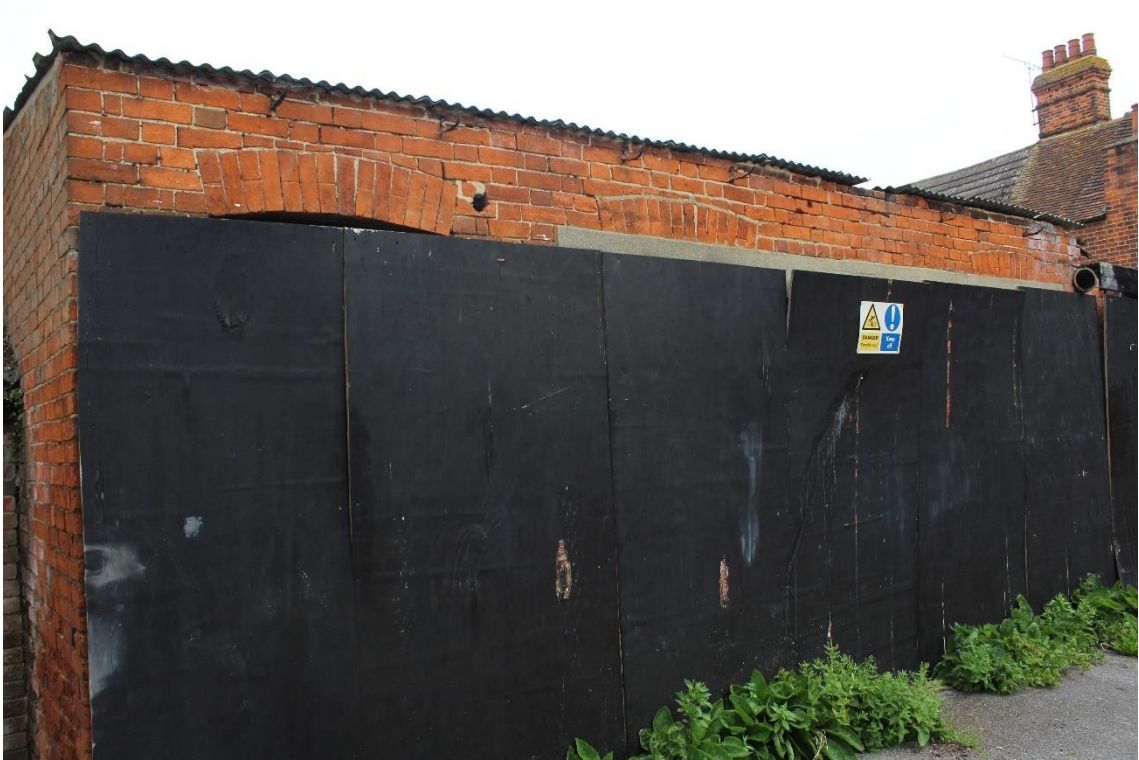
Plate 4: External oblique view NE of brick lintels – S-facing elevation
