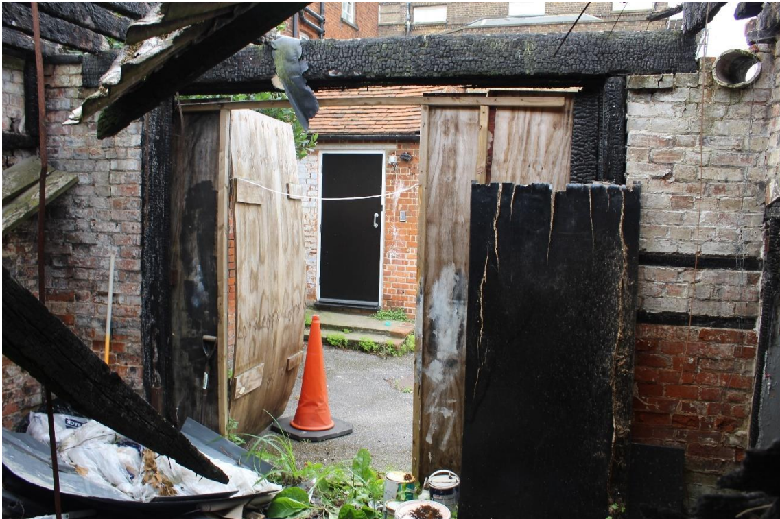
Plate 10: Internal view SSE of garage compartment
