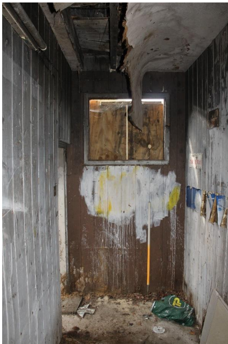
Plate 20: Internal view SSE of storage area adjoining office compartment
