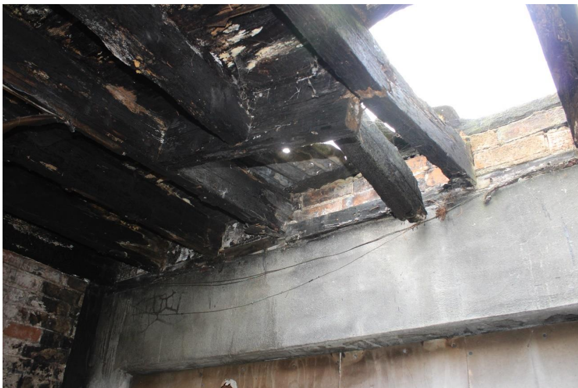
Plate 18: Internal view SSE of ceiling hatchway within office compartment
