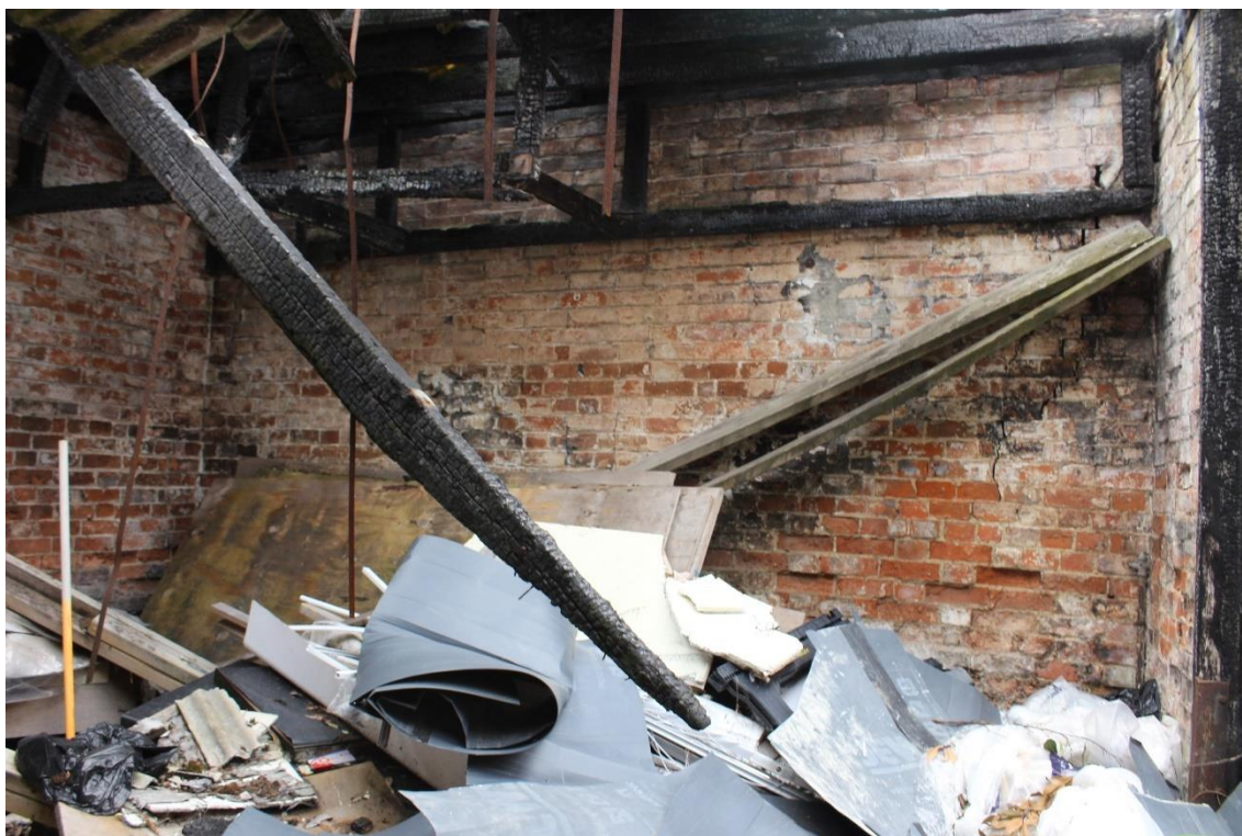
Plate 9: Internal view ENE of garage compartment
