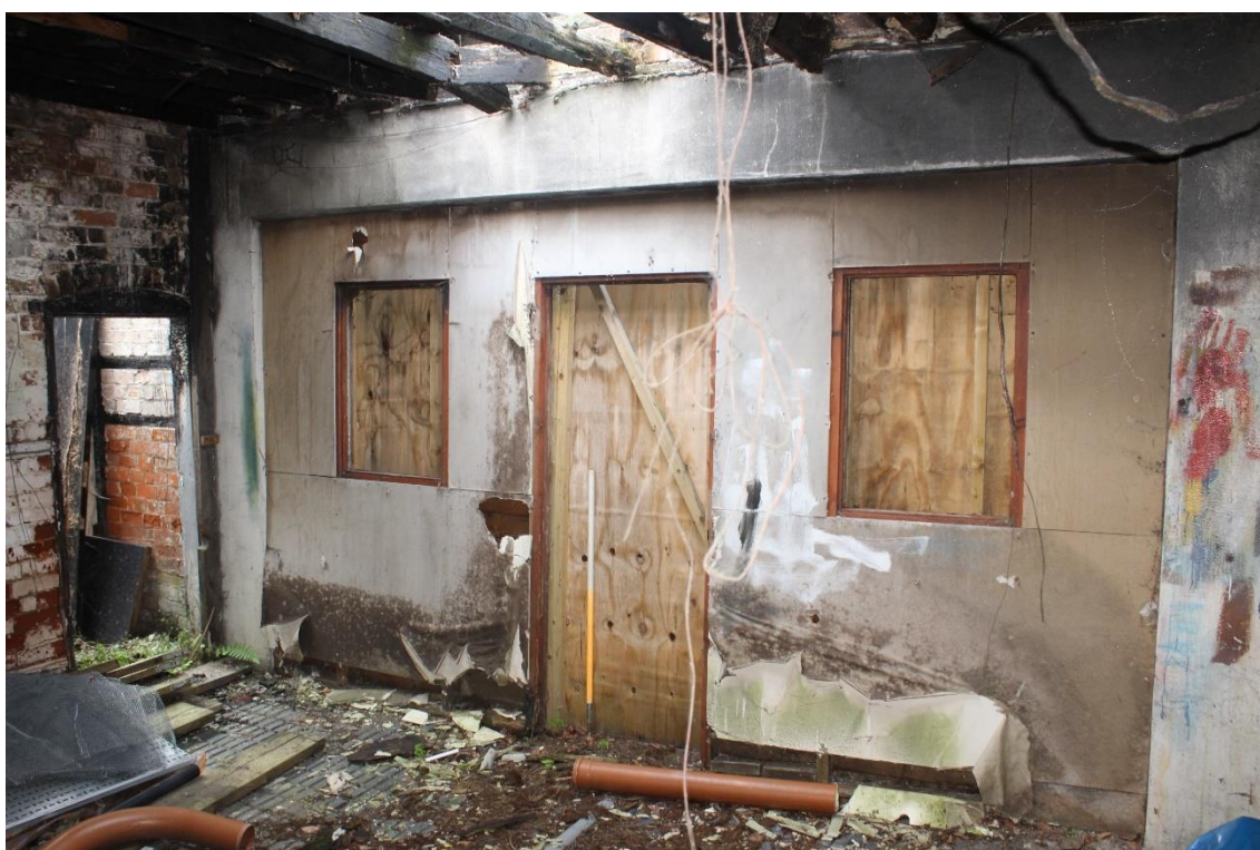
Plate 15: Internal view SSE of stud-wall within office compartment
