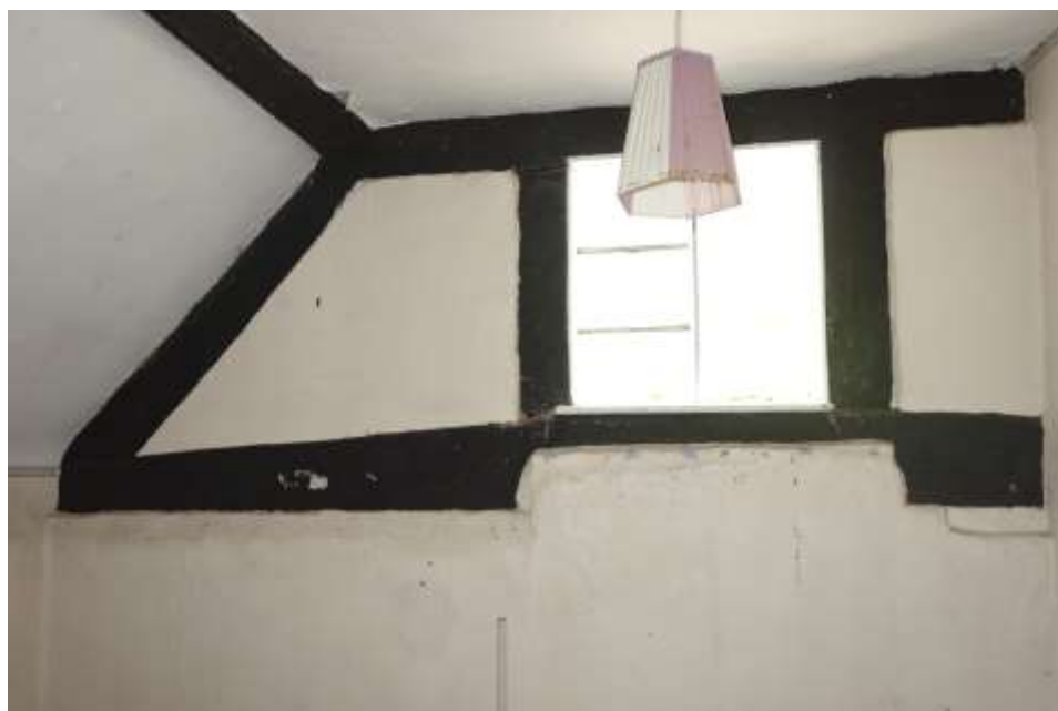
Plate 31: Internal view showing exposed timber framing and casement window in W wall of first floor room overlooking the staircase
