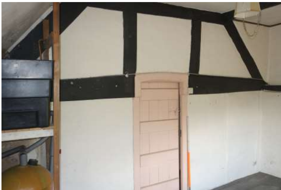
Plate 37: Internal view looking NW showing W wall of first floor SE bedroom with exposed timber framing and central low-arched plank and batten door
