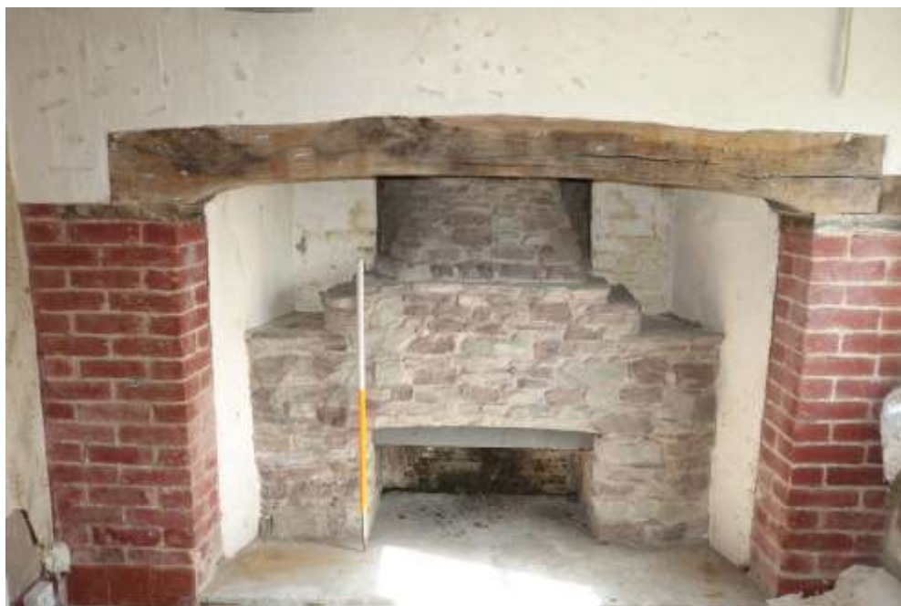
Plate 25: Internal view looking N showing inglenook fireplace in living room with stone flue flanked by brick jambs with a broad wooden overmantel
