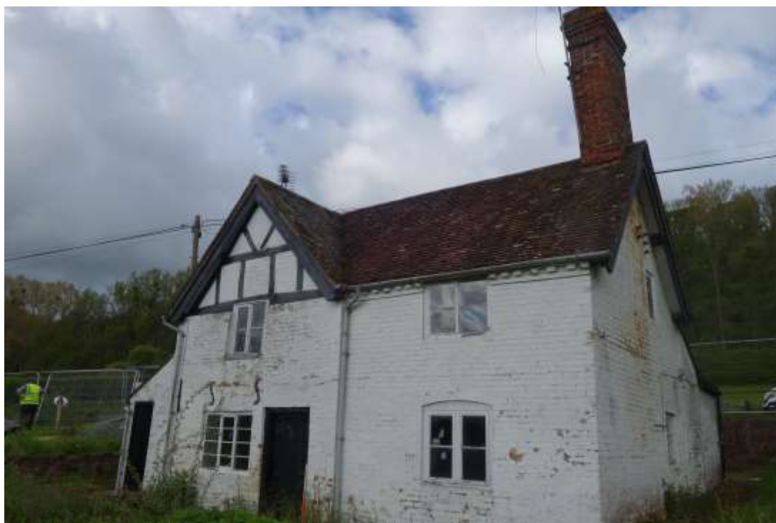
Plate 8: View looking SW of the rear elevation of the farmhouse, showing the two-storey range with dentilled eaves cornice attached to the gabled crosswing
