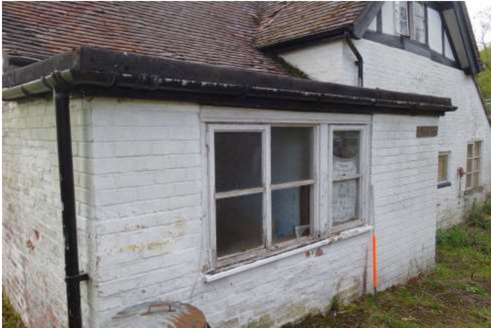
Plate 6: Oblique view looking SE showing modern single storey flat-roofed extension
