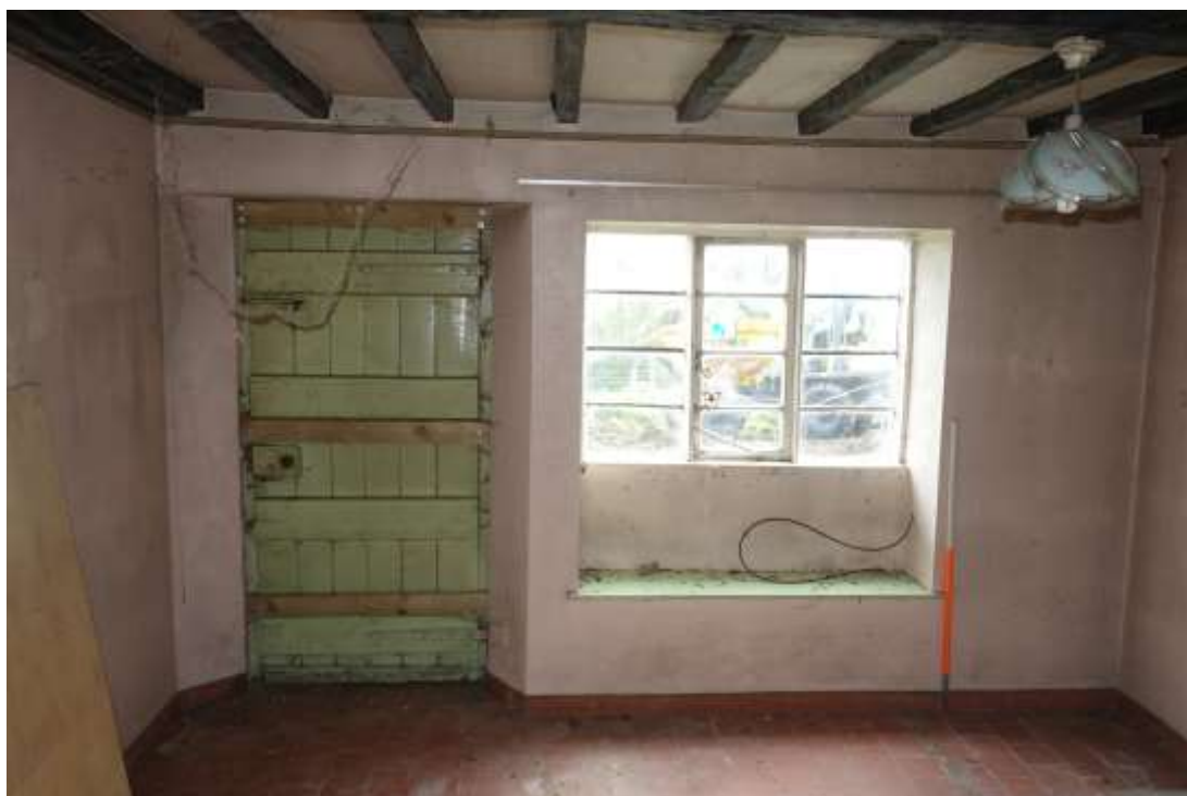
Plate 20: View looking E showing interior of dining room with 19 th century quarry tiled floor and plank and batten door to left of splayed window with modern glazed casement
