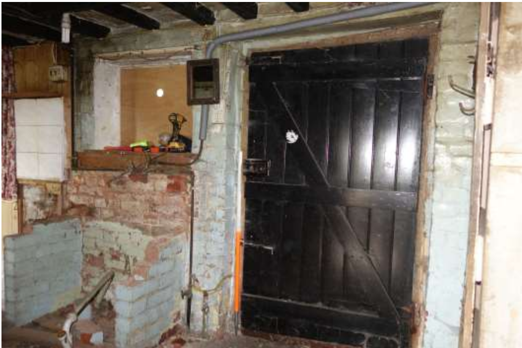
Plate 11: Internal view looking W showing ground floor lobby and main entrance
