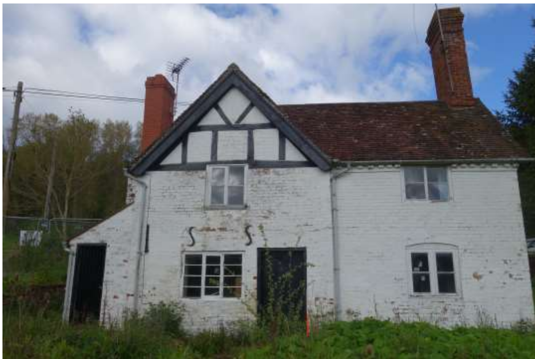
Plate 7: View looking W showing rear (E-facing) elevation with exposed timber-framing in the apex of the gable
