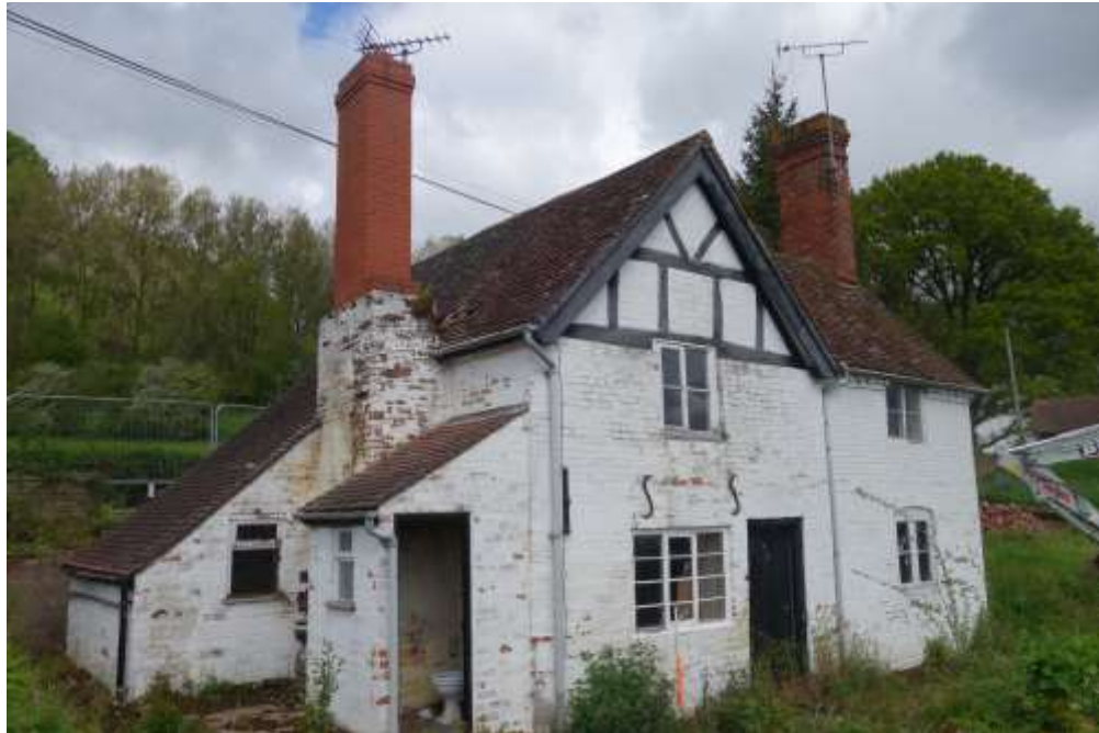
Plate 9: Oblique view looking NW showing the chimney at the S end of the farmhouse flanked by lean-to outhouse and kitchen extensions
