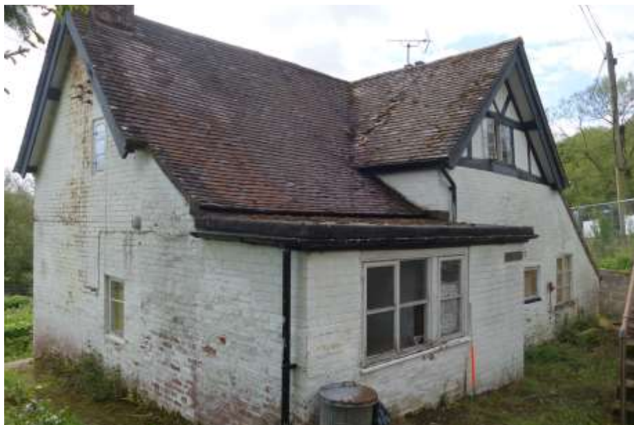
Plate 2: Oblique view SSE showing front elevation farmhouse with gabled crosswing and modern flat-roofed extension
