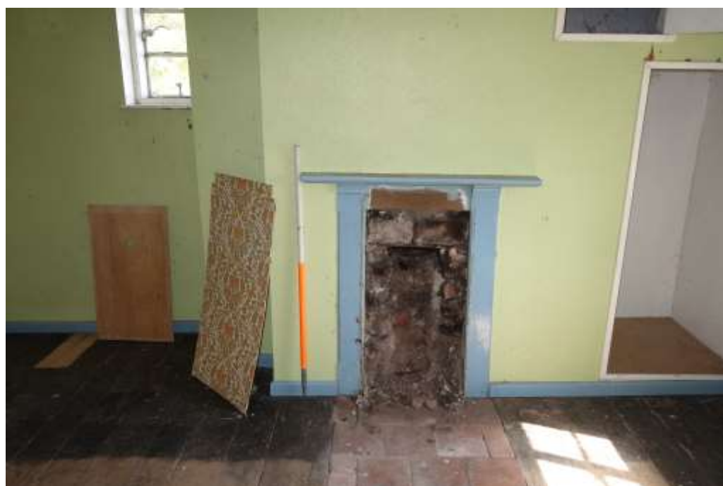
Plate 42: View looking N showing detail of fireplace in master (NE) bedroom
