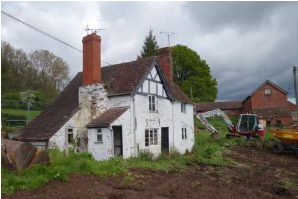
Plate 1: General view NNW showing the rear of the farmhouse with range of brick outbuildings to the N
