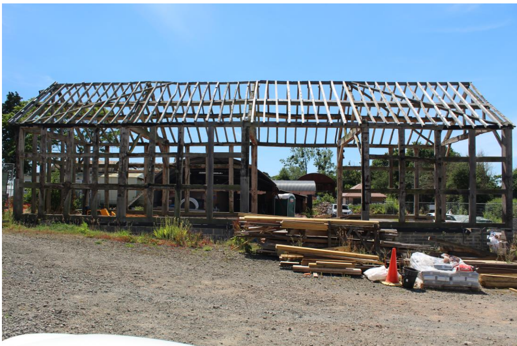
Plate 7: External view S of the N elevation
