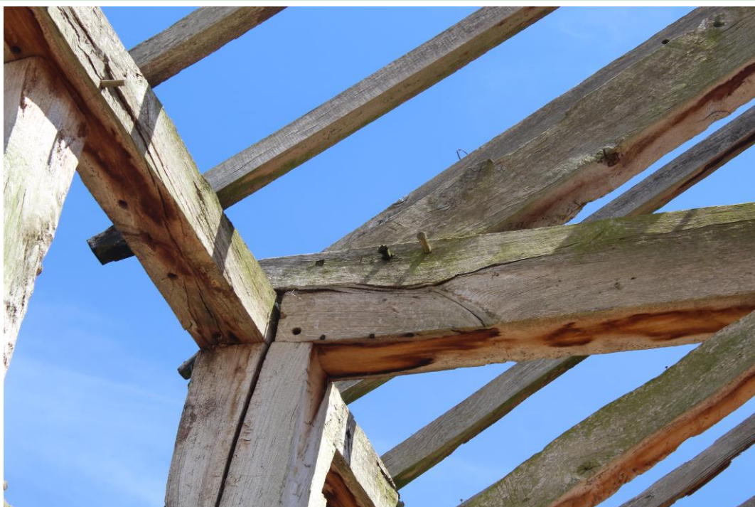
Plate 19: Internal view ENE showing the carpenters' marks on the N end of the E roof-truss
