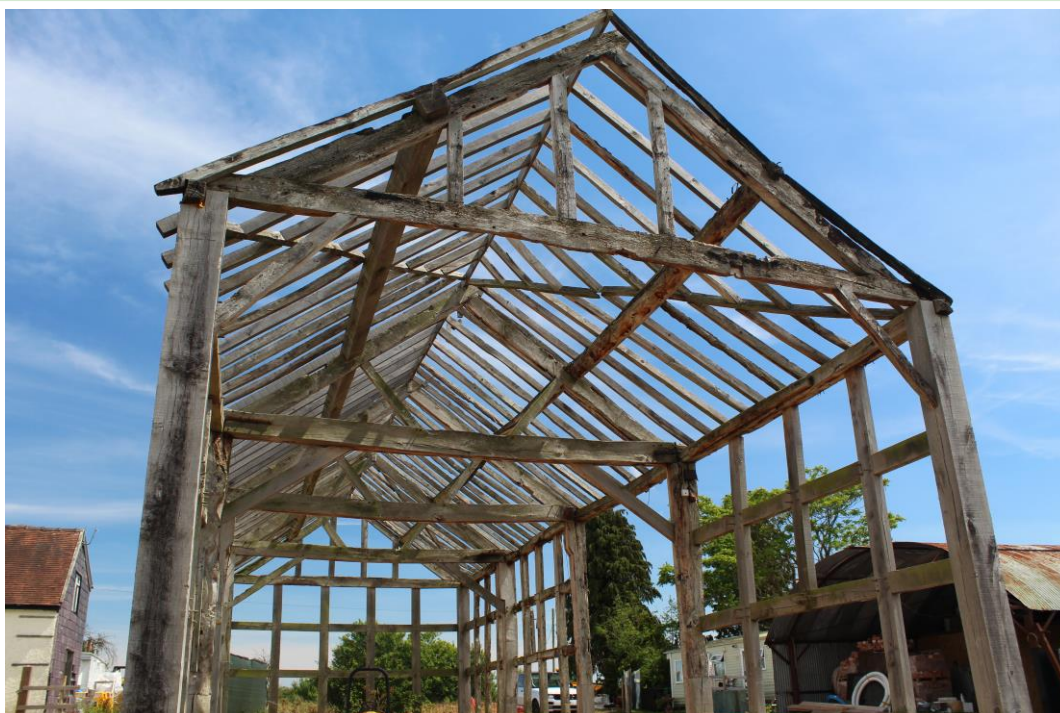
Plate 11: External view ESE showing the roof structure
