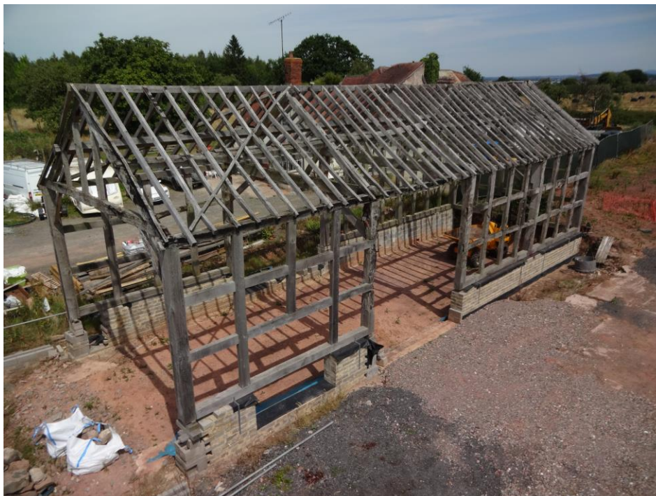
Plate 1: External view ENE of the S and W facing elevations
