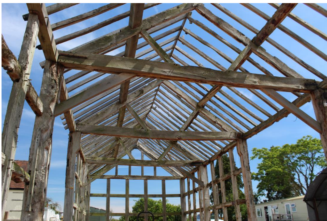
Plate 12: Internal view ESE of the roof-trusses
