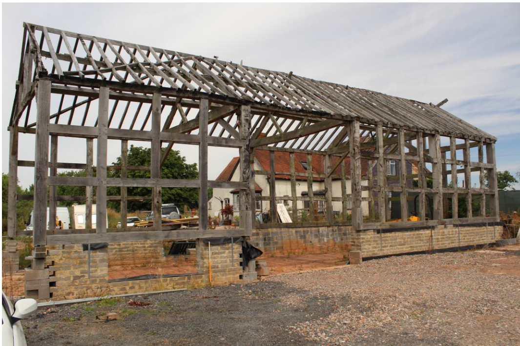
Plate 6: External view NNE showing the principal S-facing elevation
