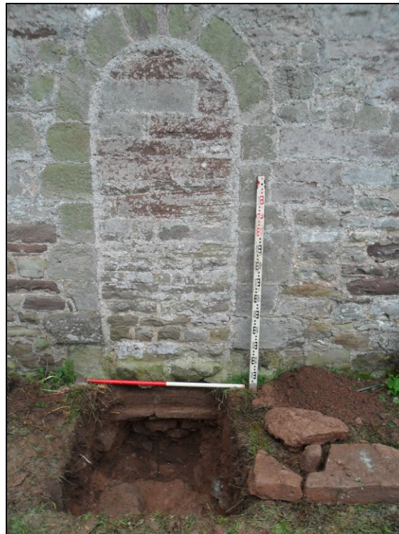
Plate 5: South facing view of wall [114] in relation to wall [116]
