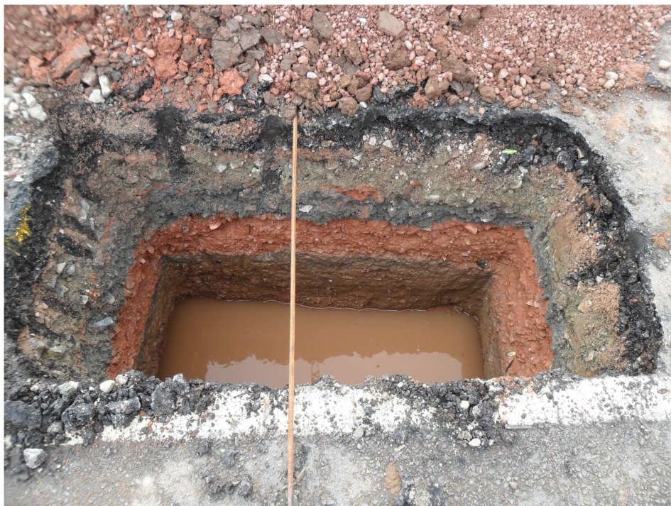
Plate 8: N-facing section of TP108
