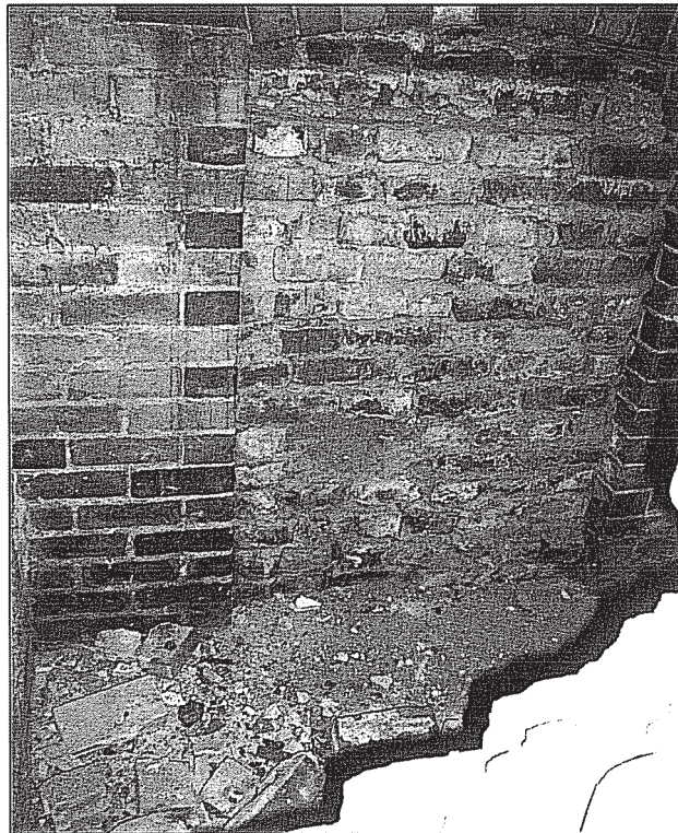
Fig. A5.2 Bricked-up archway in western protrusion wall
