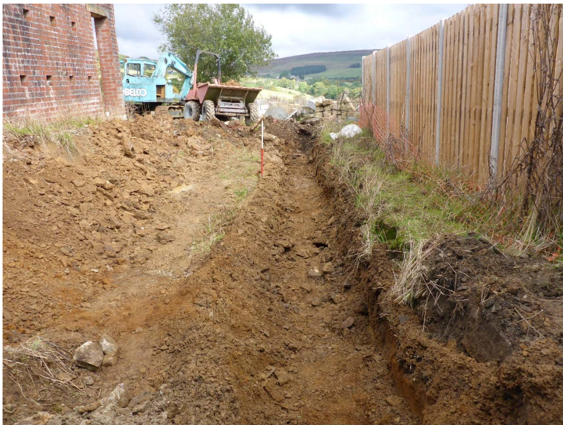
Plate 5: Post-excitation view of north-south foundation trench, viewed facing north
