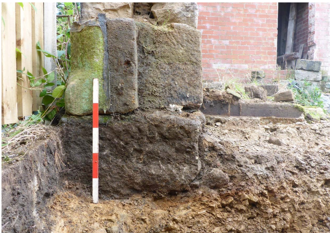
Plate 2: East end of standing wall with chamfered stone and foundation, viewed facing west
