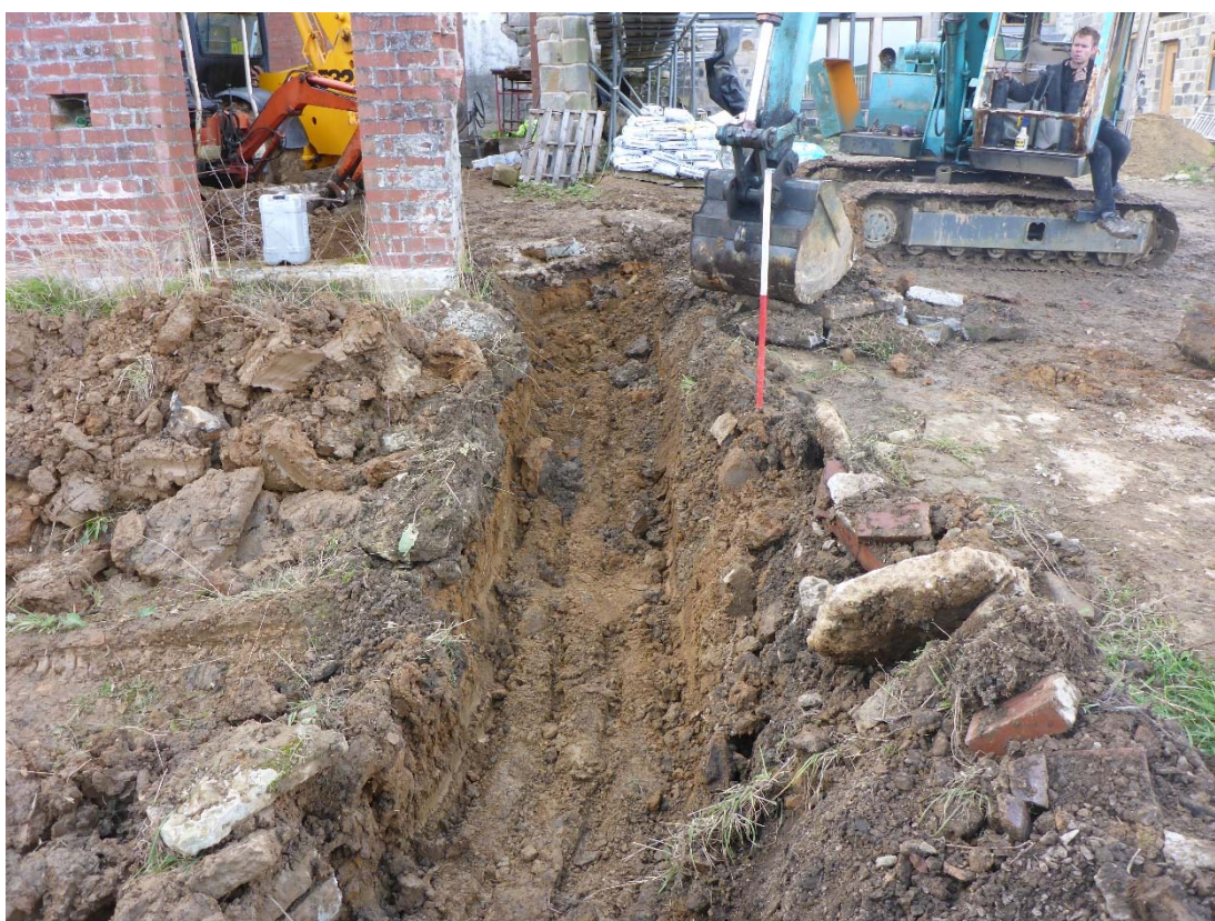
Plate 6: Western continuation of foundation trench, viewed facing west.
