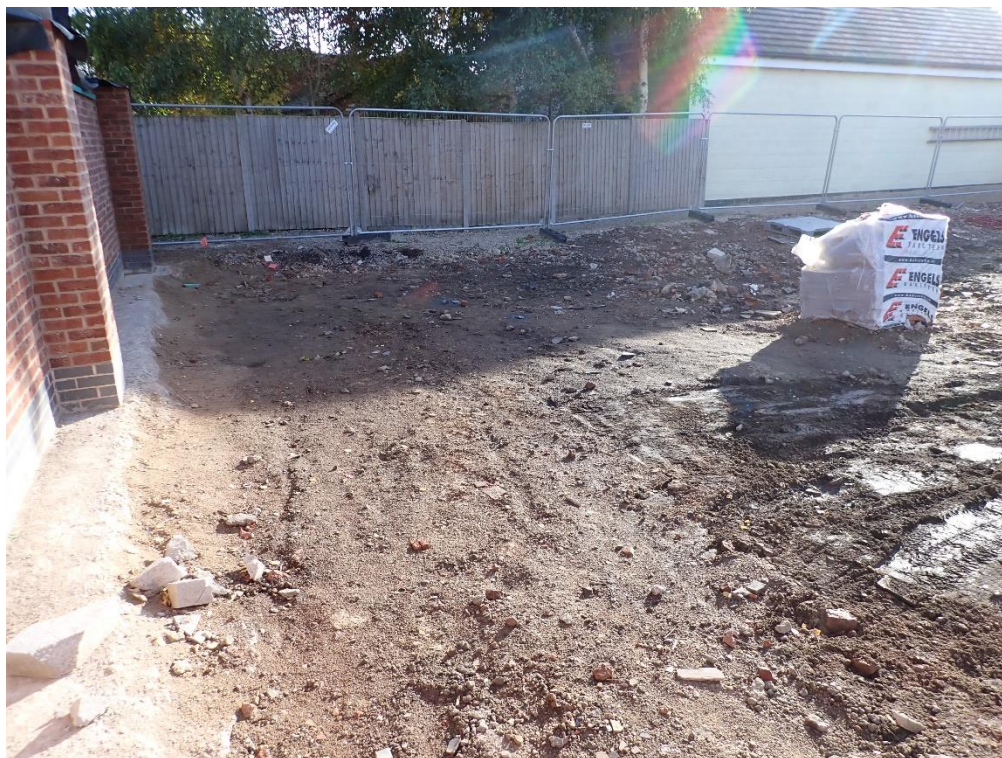
Plate 11: Trench Two, pre excavation, looking east, no scale
