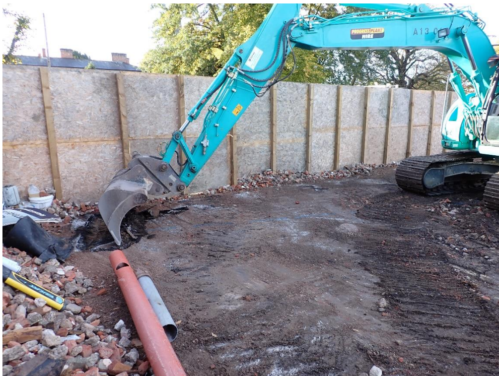
Plate 01: Pre excavation, general site view looking northwest, no scale
