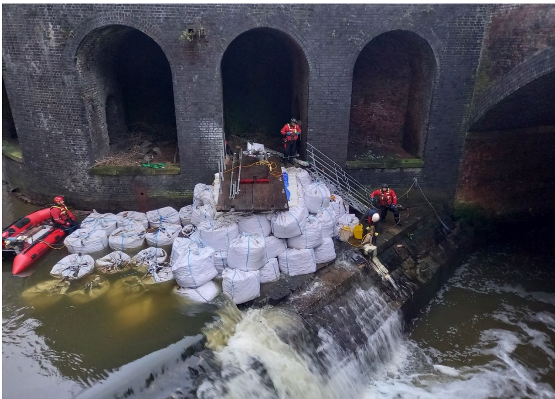
Plate 2: Coring undertaken through the Scotland Weir.
