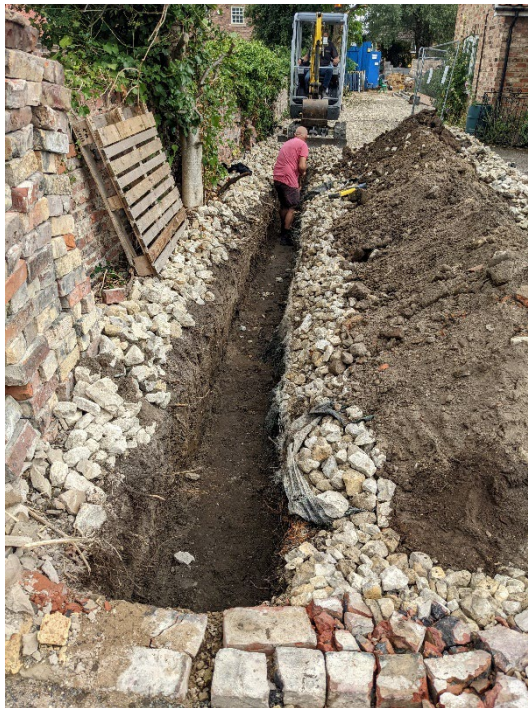
Plate 6 Location of service trench, looking north
