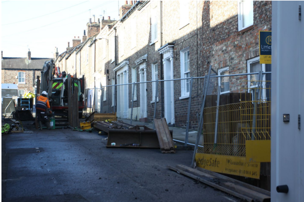
Plate 1 View of works, facing south-west
