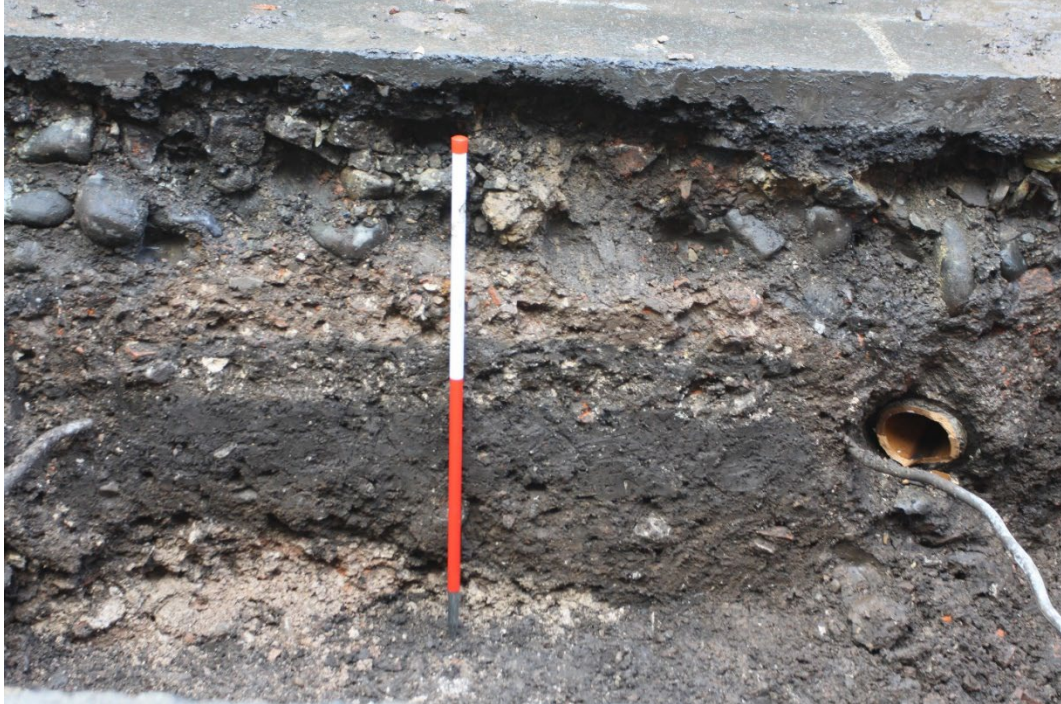
Plate 4 South-west facing section of Trench 2
