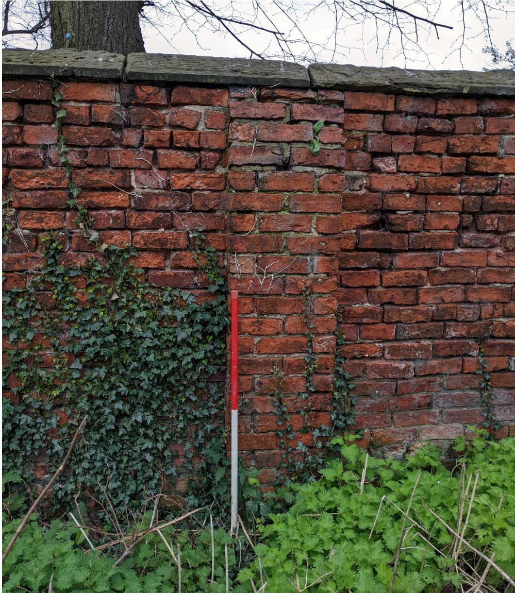
Plate 3 Condition of interior wall
