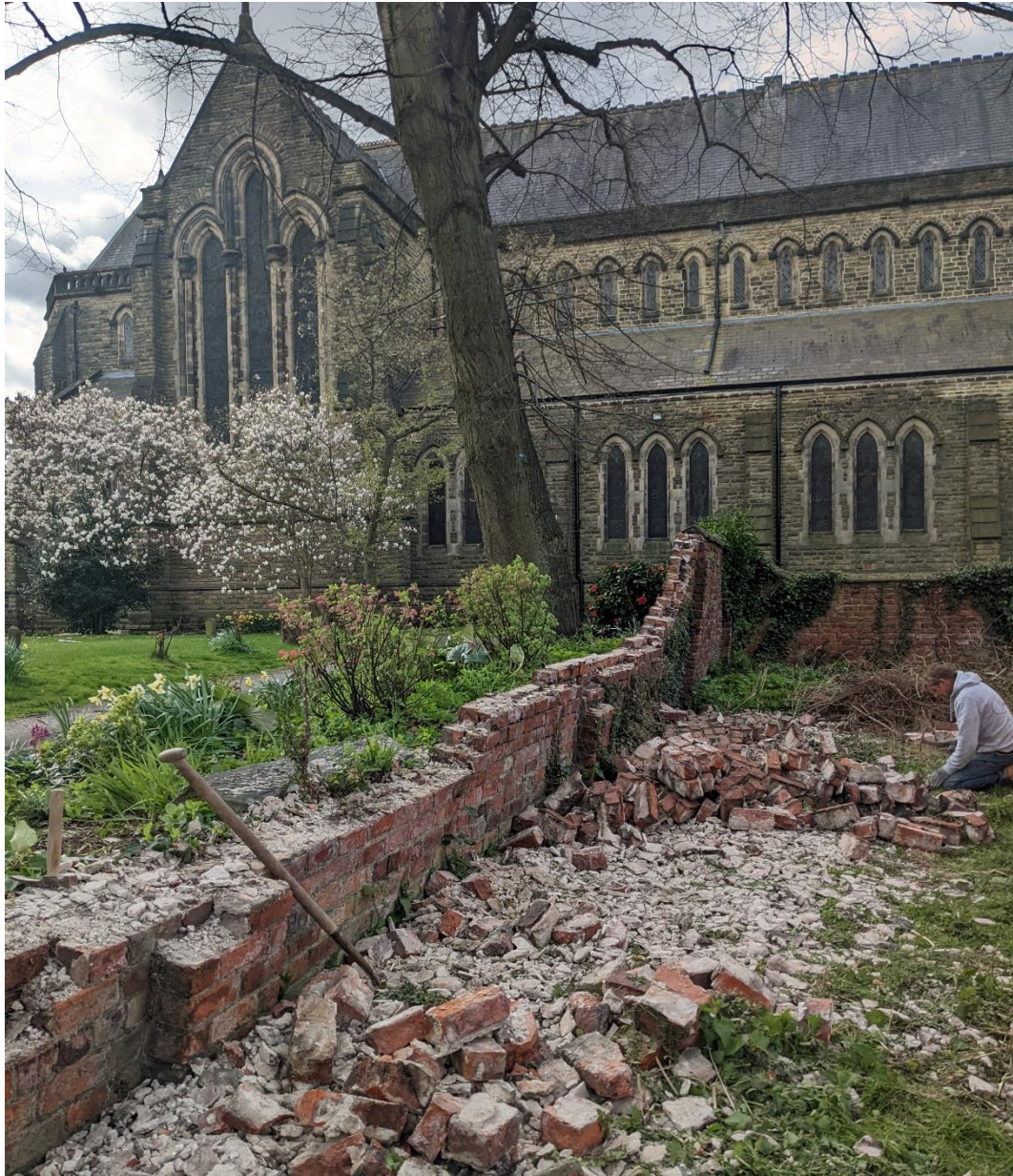
Plate 5 Wall during demolition process
