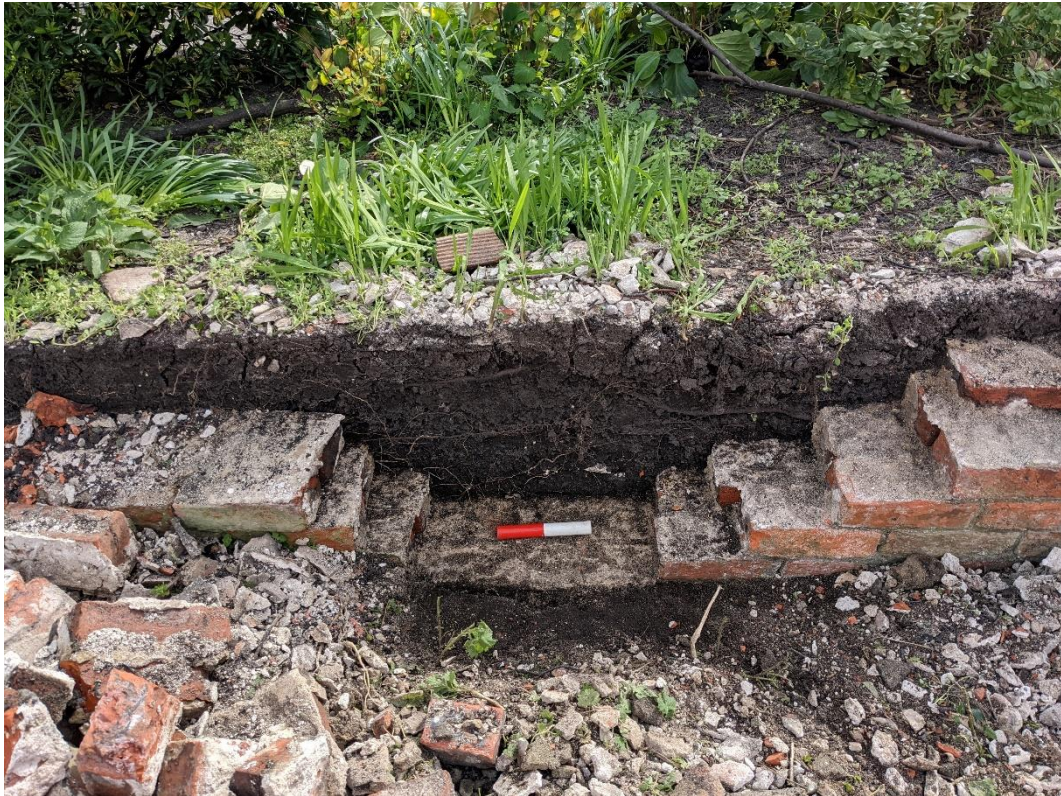
Plate 6 Wall demolished to ground level
