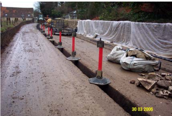
Final stages of Wessex Water sewer pipe being laid
