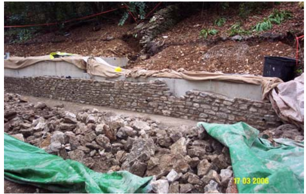
Facing stone work to the north east wall progressed well
