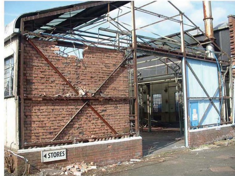
Plate 2 Mid 20th Century light-framed industrial unit
