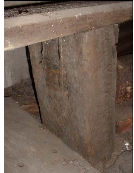
Plates 14 and 15 Original wartime benches constructed from re-used railway sleepers
