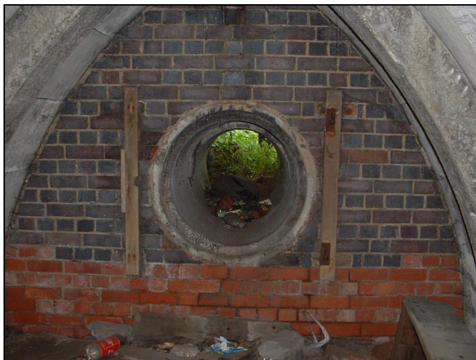
Plates 9 and 10 Rear wall of the shelter with emergency exit
