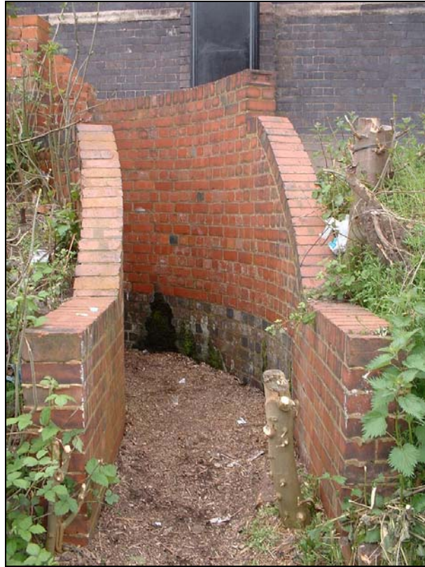
Plate 8 Anti-blast wall at entrance to Shelter 2
