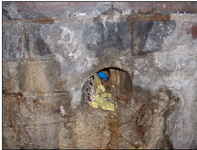
Plate 11 Detail of the flue for the stove
