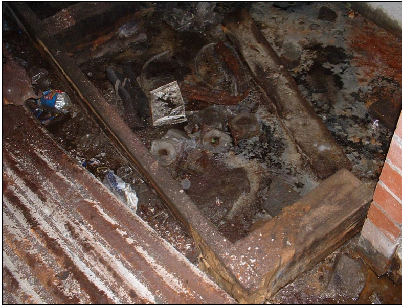
Plates 14 and 15 Original wartime benches constructed from re-used railway sleepers
