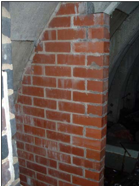
Plates 12 and 13 Brick dividing walls to provide WC cubicles
