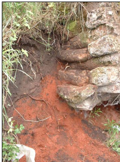
Plate 4 Detail of sand and sandbag covering
