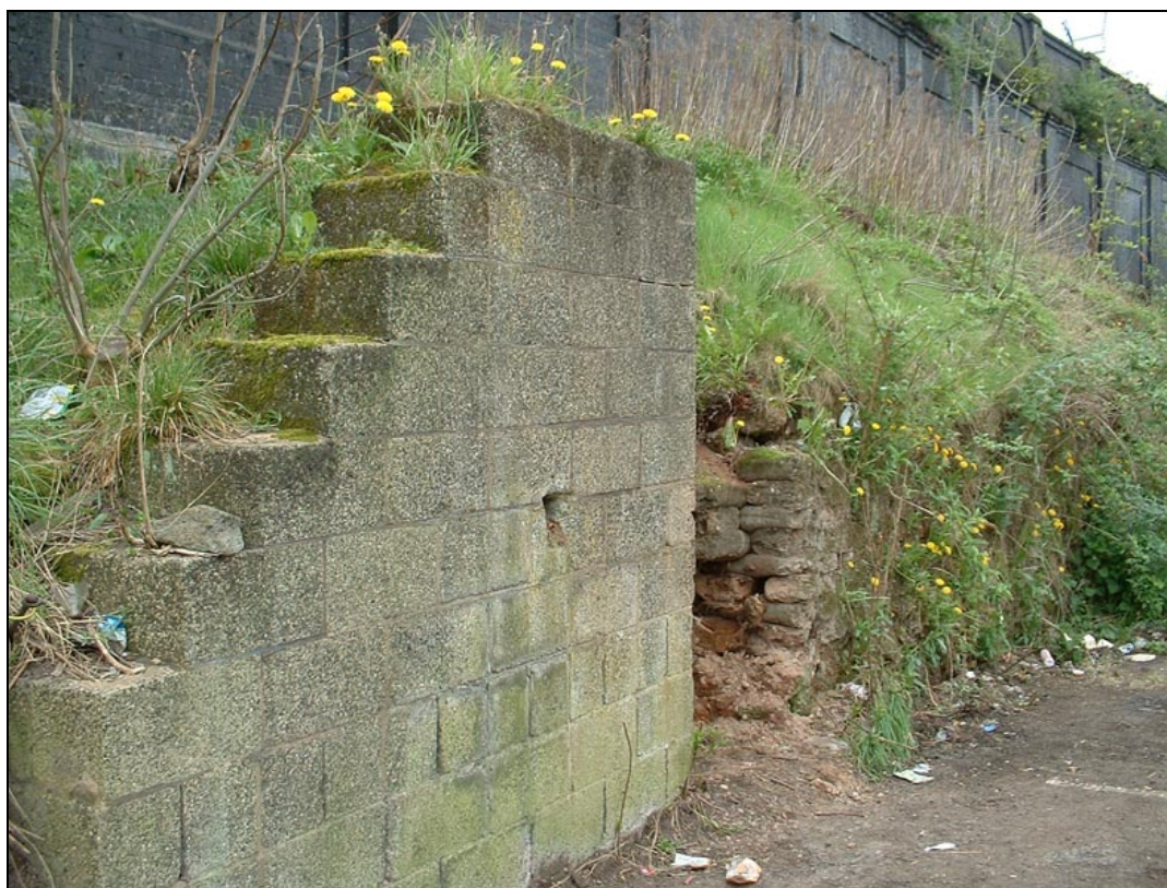
Plate 7 Anti-blast wall at entrance to Shelter 1
