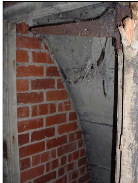
Plates 12 and 13 Brick dividing walls to provide WC cubicles
