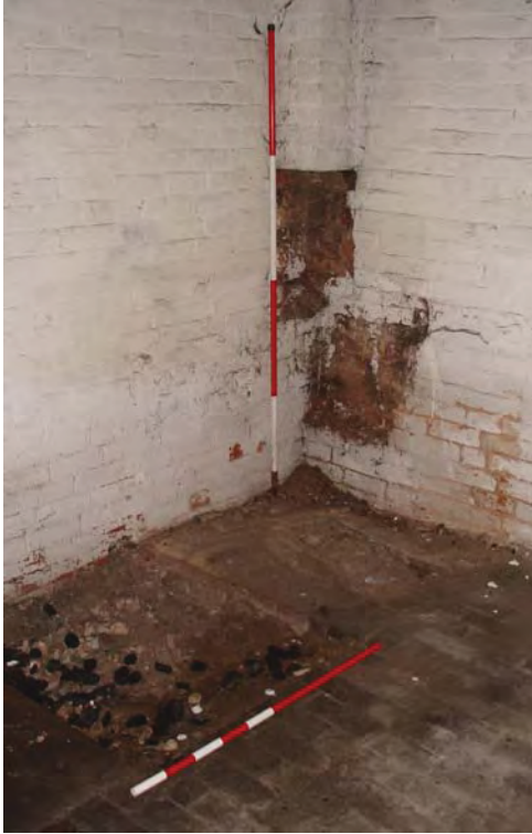
Plate 20: Block C, Room 9; detail of flue.
