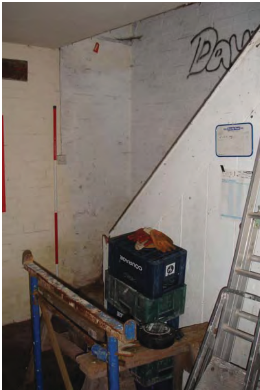
Plate 16: Block B, Room 3; staircase.
