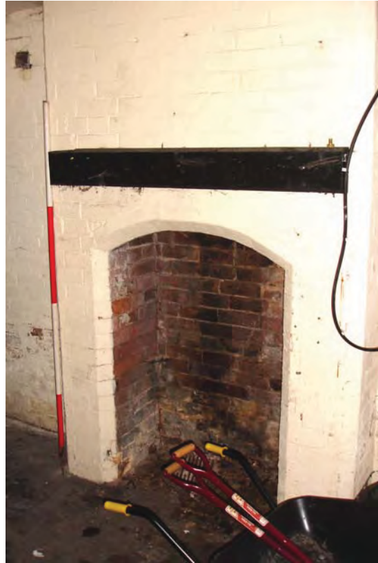
Plate 15: Block B, Room 3; fireplace
