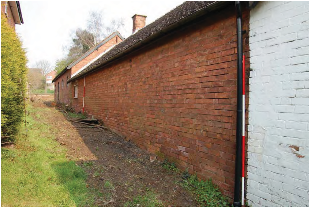
Plate 12: Block C, west elevation; oblique view from south-west.
