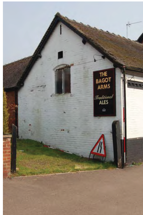
Plate 11: Block A (west); note blocked door to left.
