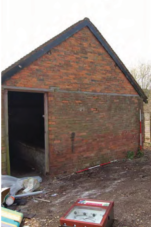
Plate 8: Block D, north elevation.
