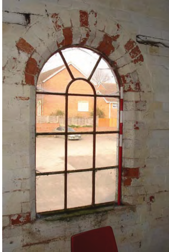
Plate 17: Block B, Room 4; window detail.
