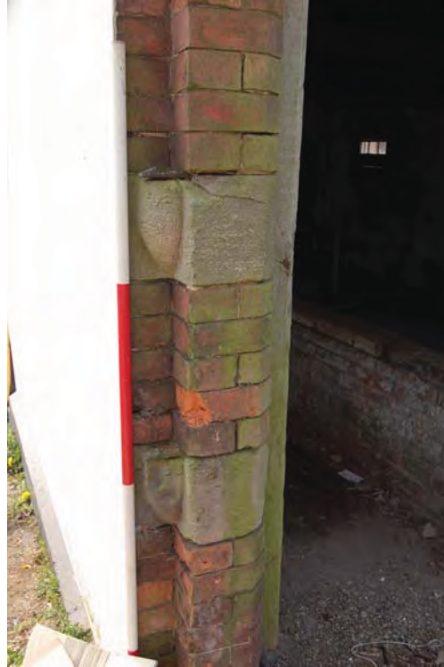
Plate 9: Block D; detail of jamb at NE corner.
