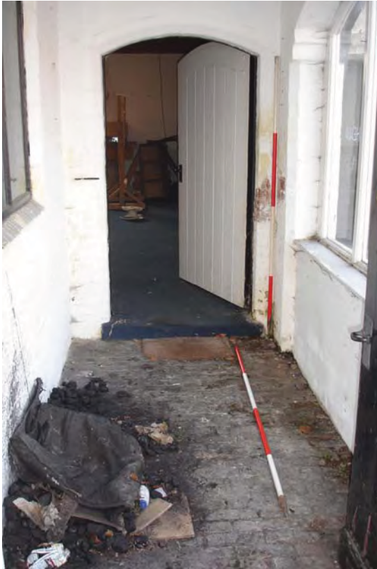
Plate 14: Block B, Passage 2, looking west.
