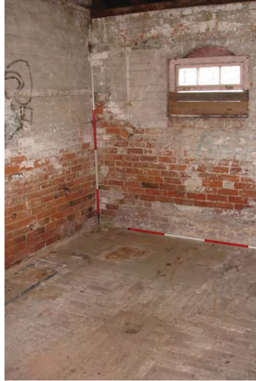
Plate 21: Block D, Room 10 looking south-west.
