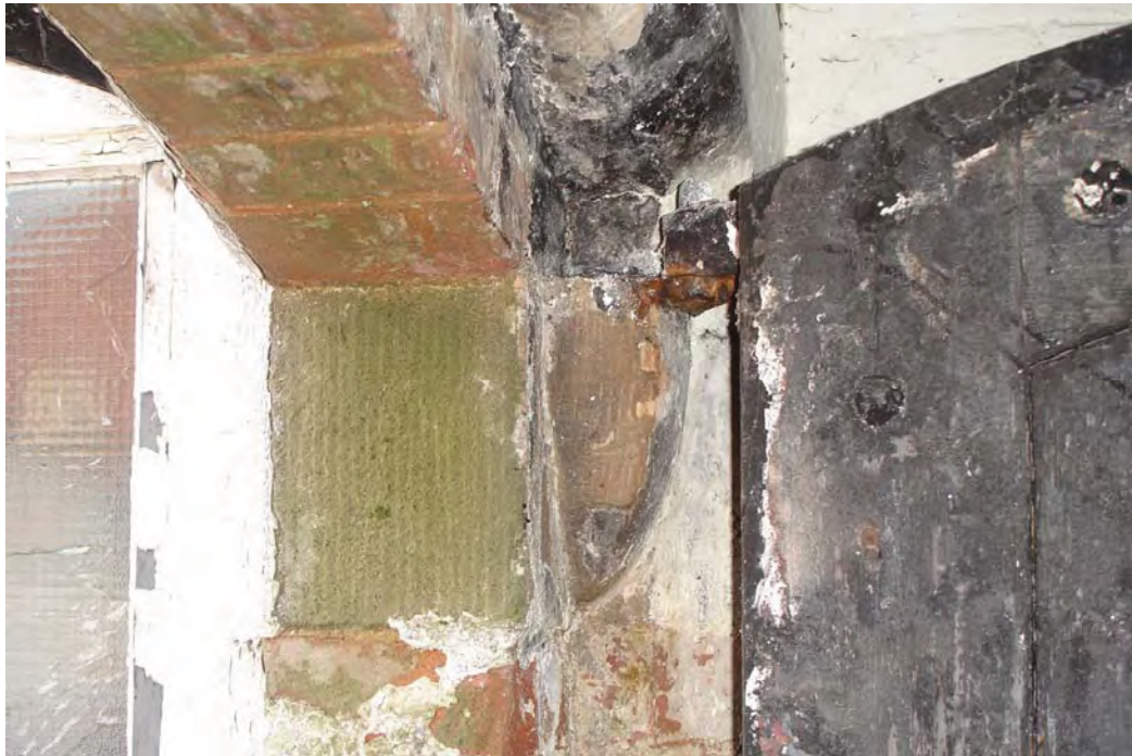
Plate 19: Block C, Room 5; detail of moulded stone block in jamb supporting iron door pintle (compare Plate 9).
