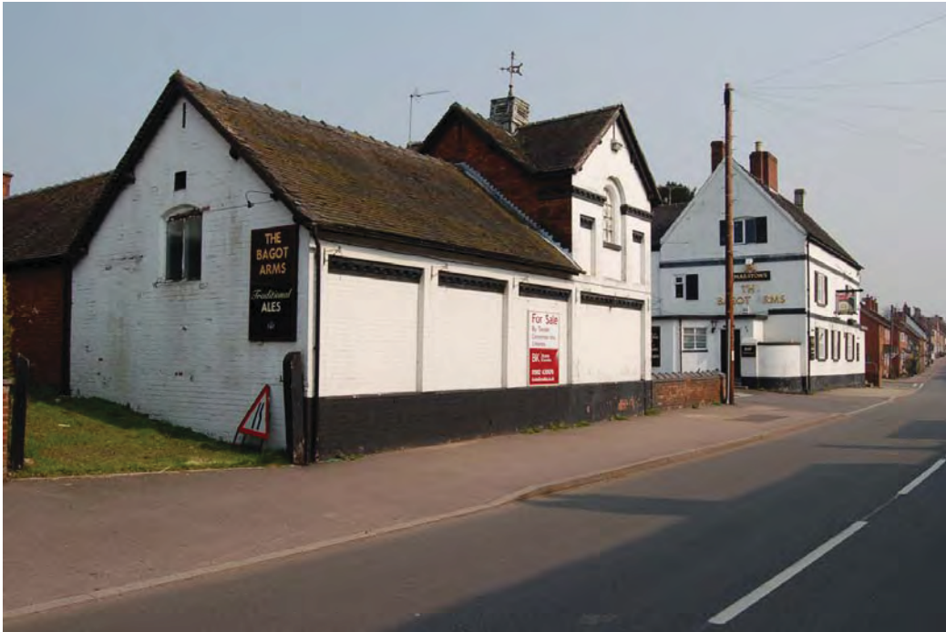
Plate 1: Contextual view from the south-west with C18th Bagot Arms Public House in background.
