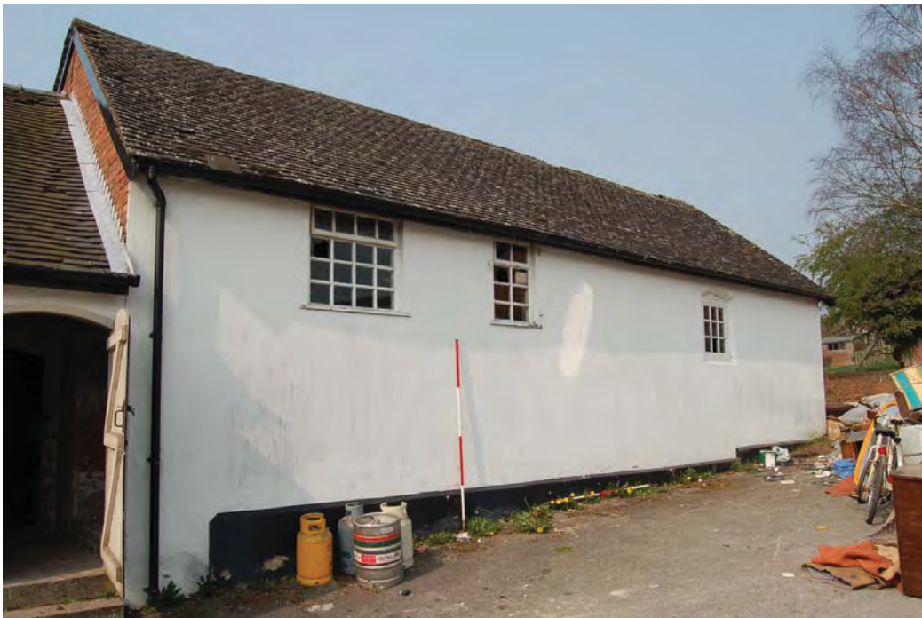
Plate 7: Block D, east elevation.
