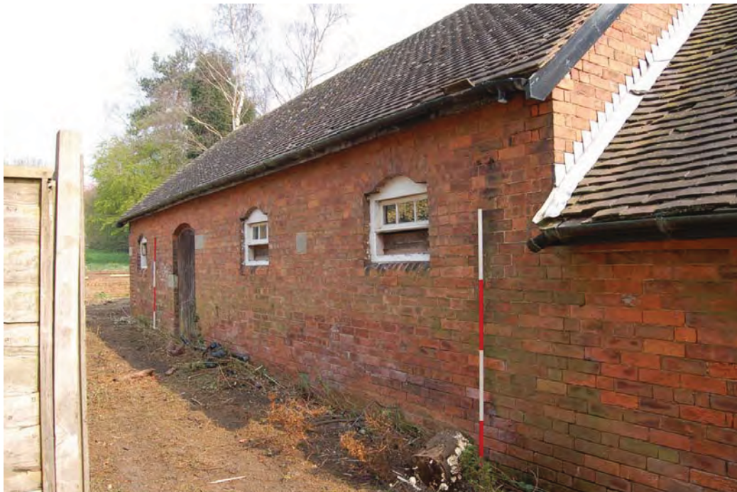
Plate 13: Block D, west elevation; oblique view from south-west.
