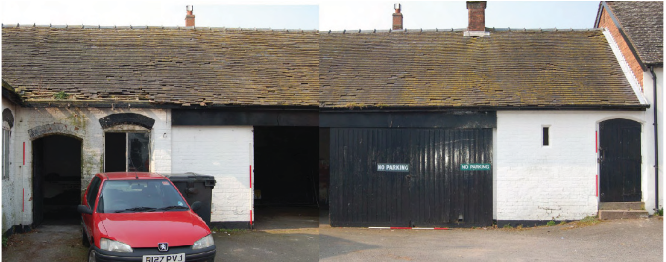
Plate 6: Block C, east elevation (composite photograph).
