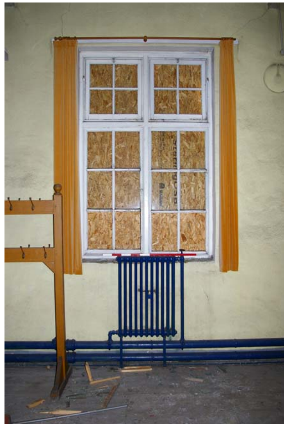
Plate 10: West Range; fenestration detail.
