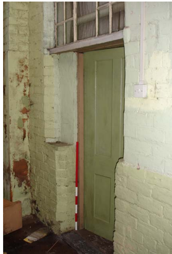
Plate 6: West Range; door formed from window.
