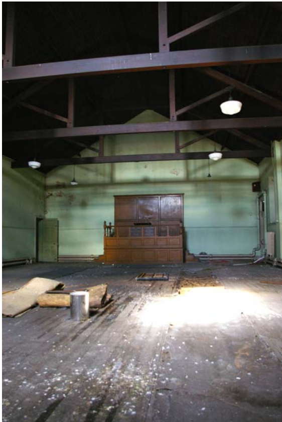
Plate 11: East Range, looking north.
