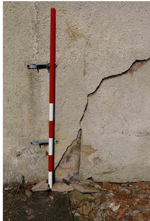
Plate 3: South elevation, straight joint.
