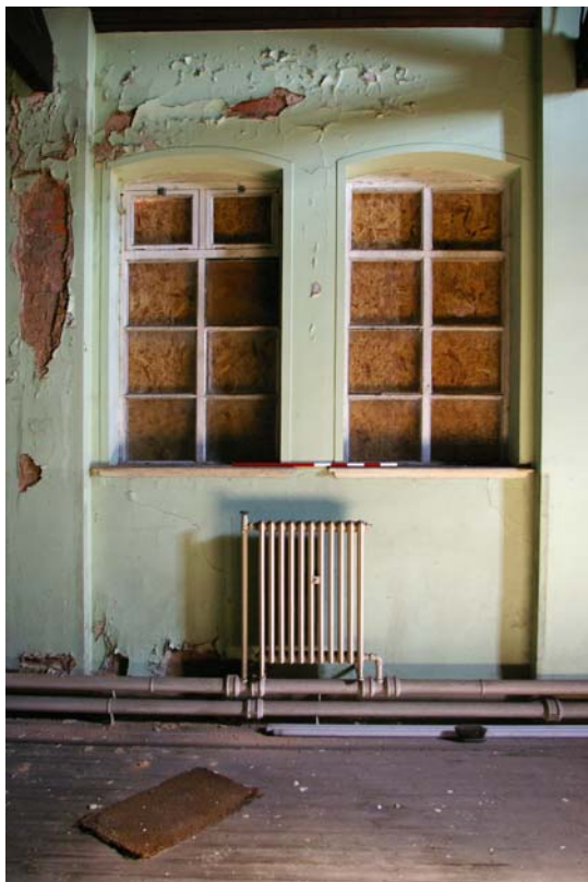
Plate 13: West Range; detail of fenestration.
