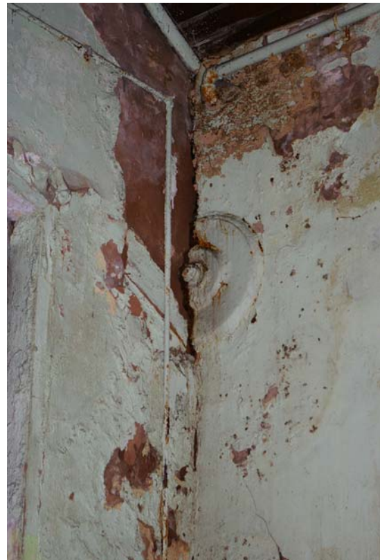
Plate 14: West Range brickwork butting against endplate of tie of earlier east range.
