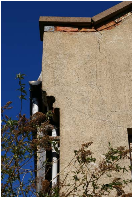
Plate 2: Detail of moulded brick eaves.
