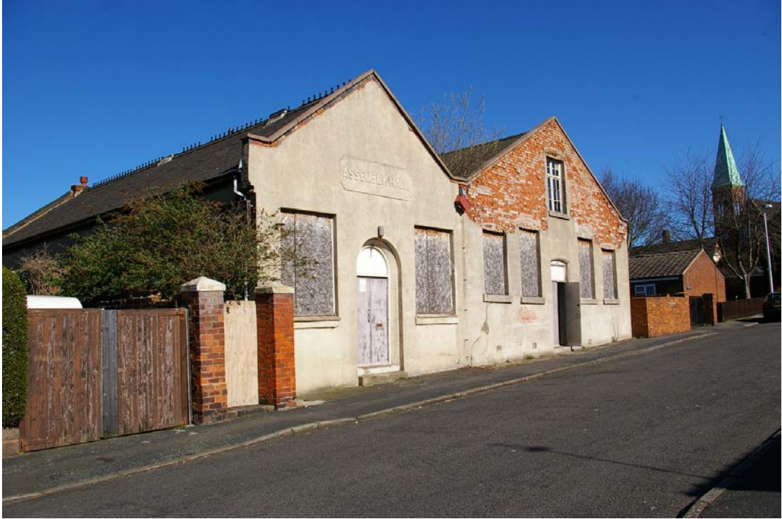
Plate 1: General exterior view from the south-west.
