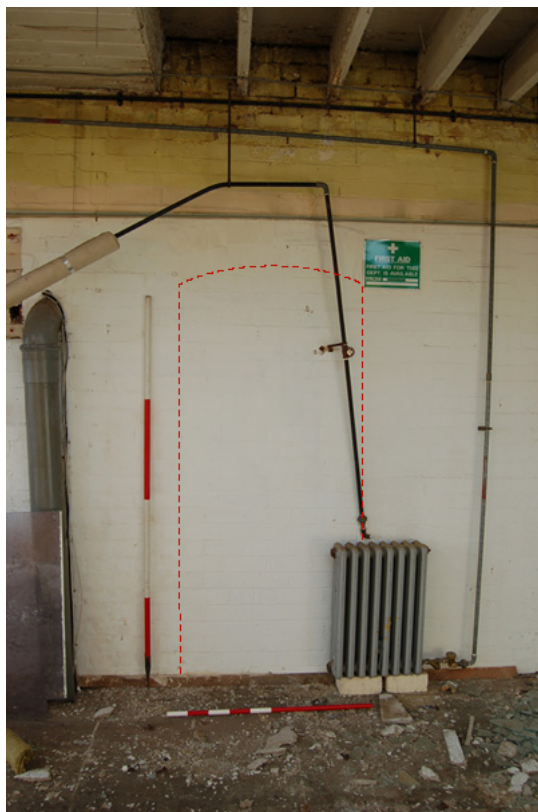
Plate 39: Room F9, blocked door (in red)
