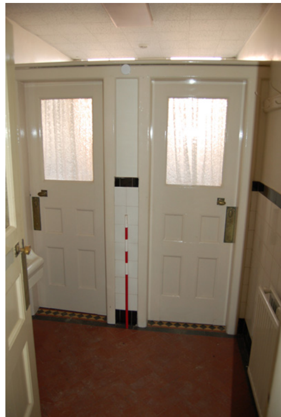
Plate 22: Room G11, original doors.
