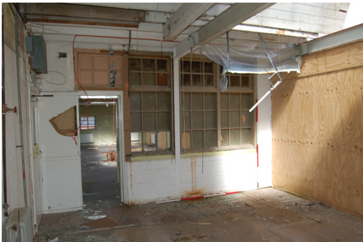
Plate 38: Room F9, west wall.
