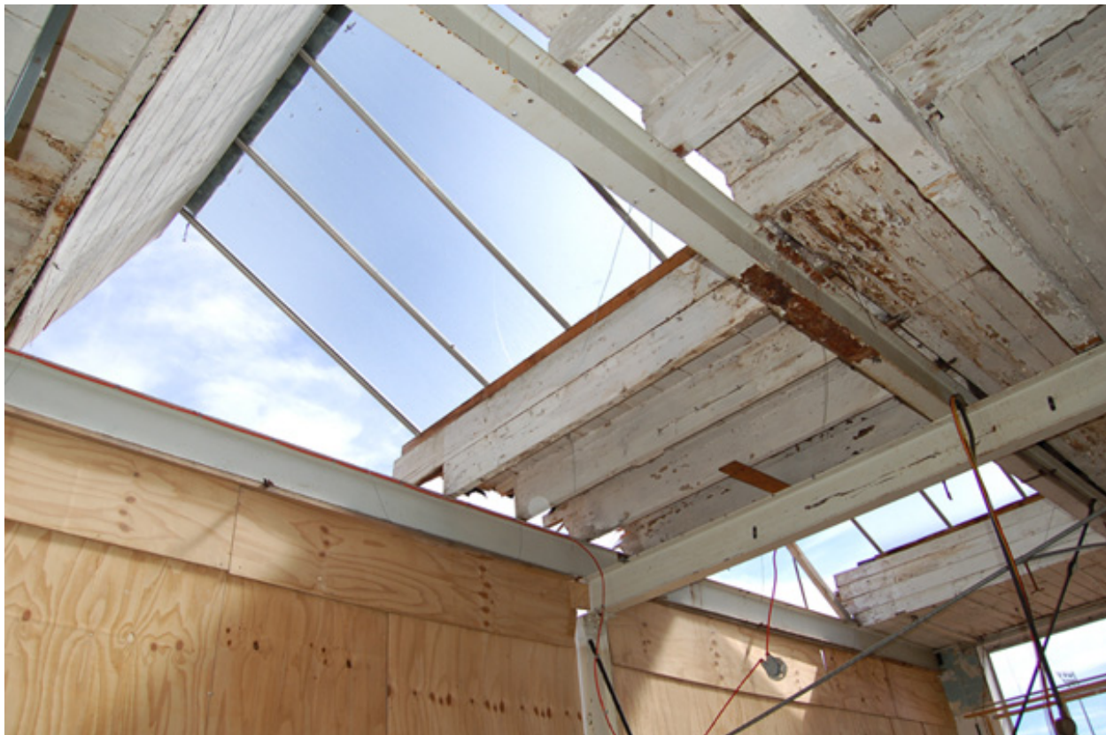
Plate 37: Room F9, roof structure.
