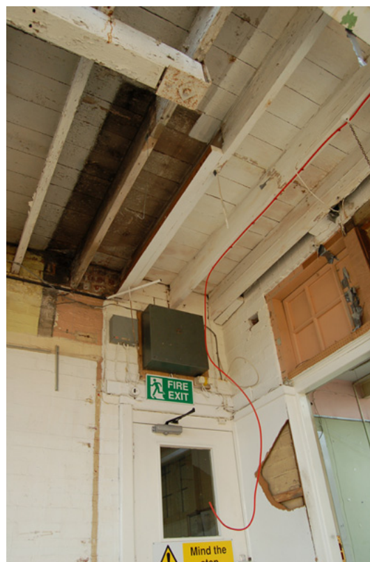
Plate 40: Room F9, south-west corner.
