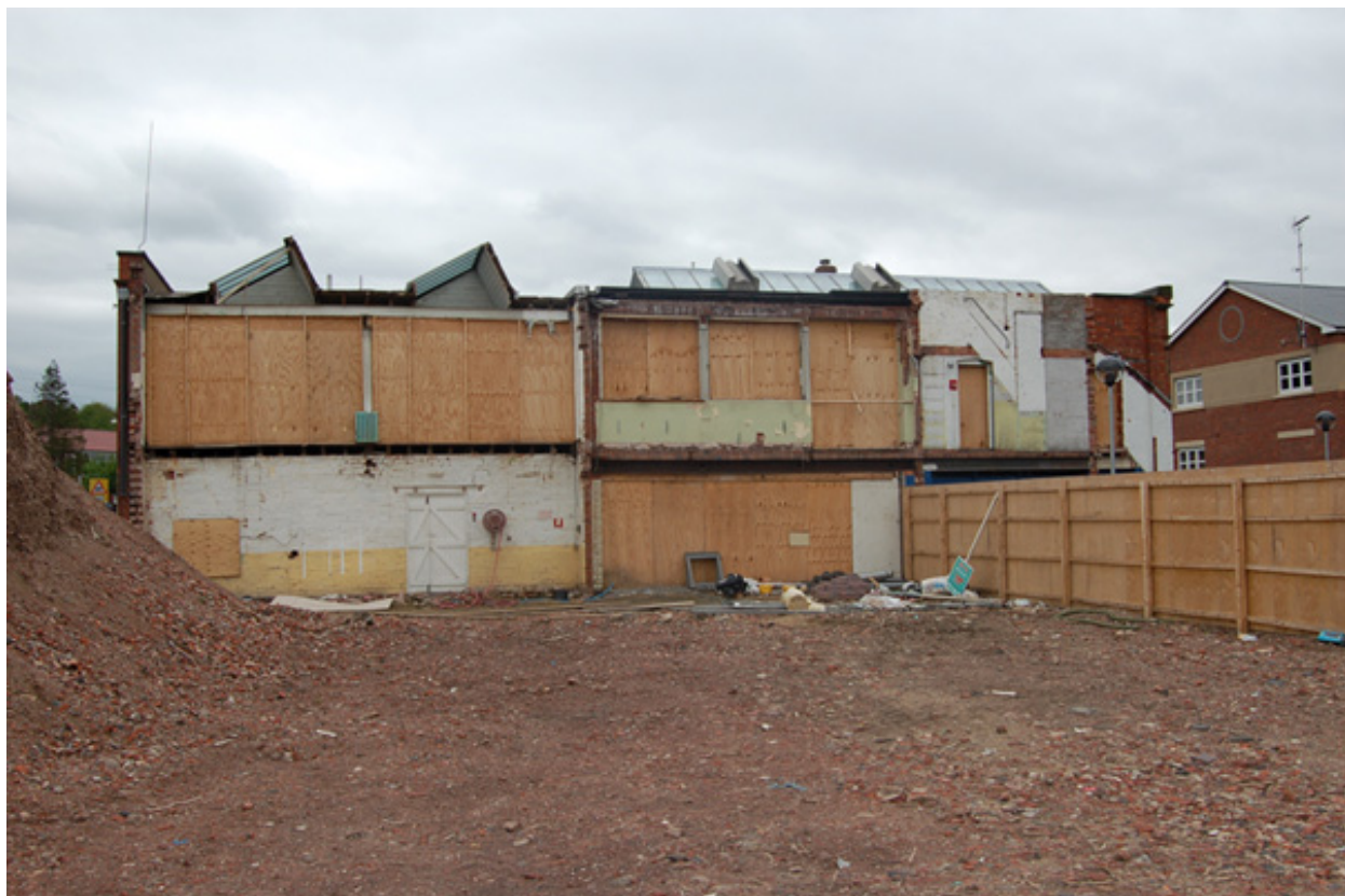
Plate 7: North (rear) elevation.
