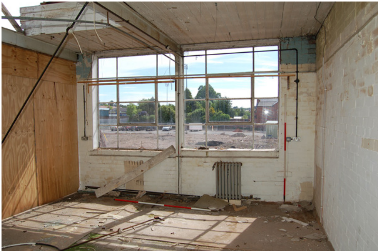
Plate 36: Room F9, looking east.
