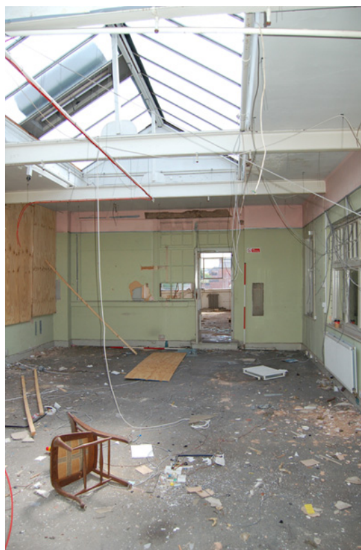
Plate 35: Room F8, looking east.
