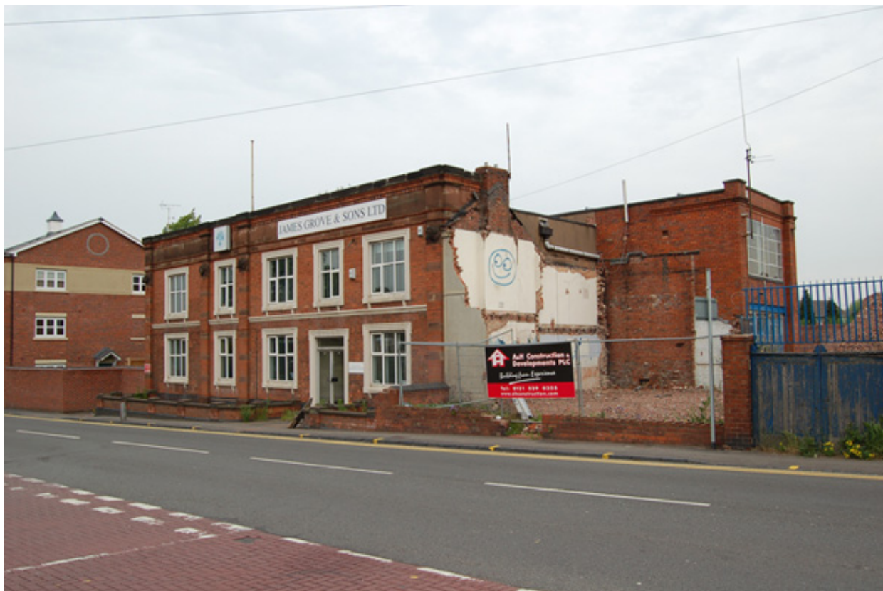
Plate 1: Contextual view from the south-east.
