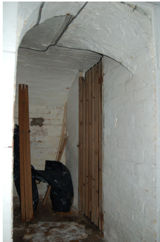
Plate 13: Basement Room B2 and lobby.
