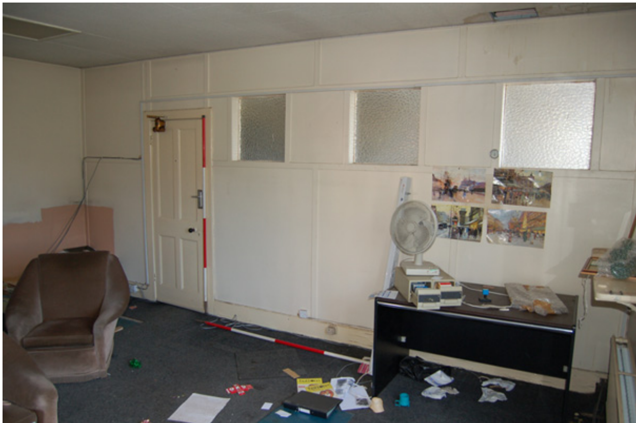
Plate 31: Room F4, looking north-east.
