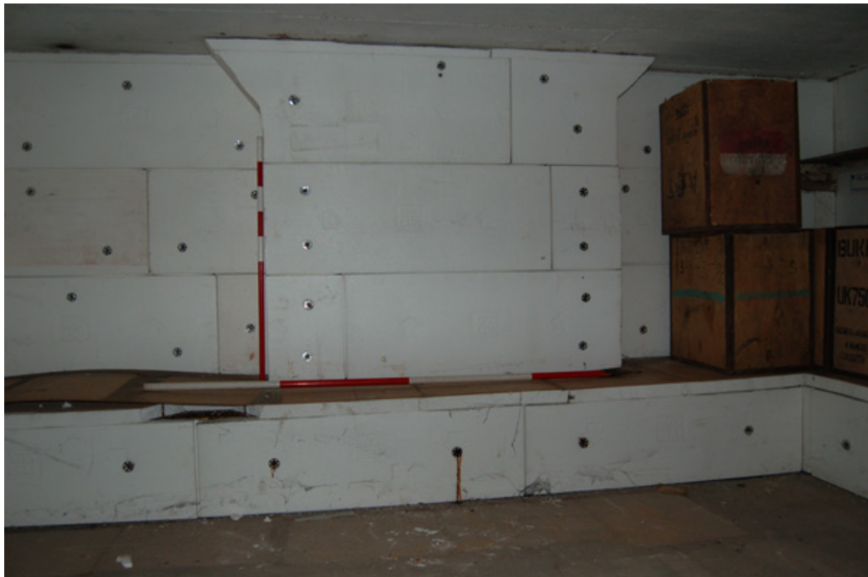
Plate 11: Basement Room B1; central projection within west wall.
