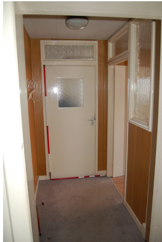
Plate 18: Studwork partitions to W end of range (G5-G8).
