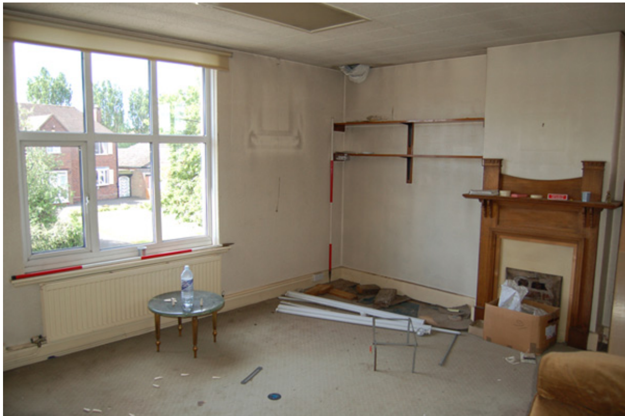
Plate 30: Room F3, looking south-west.
