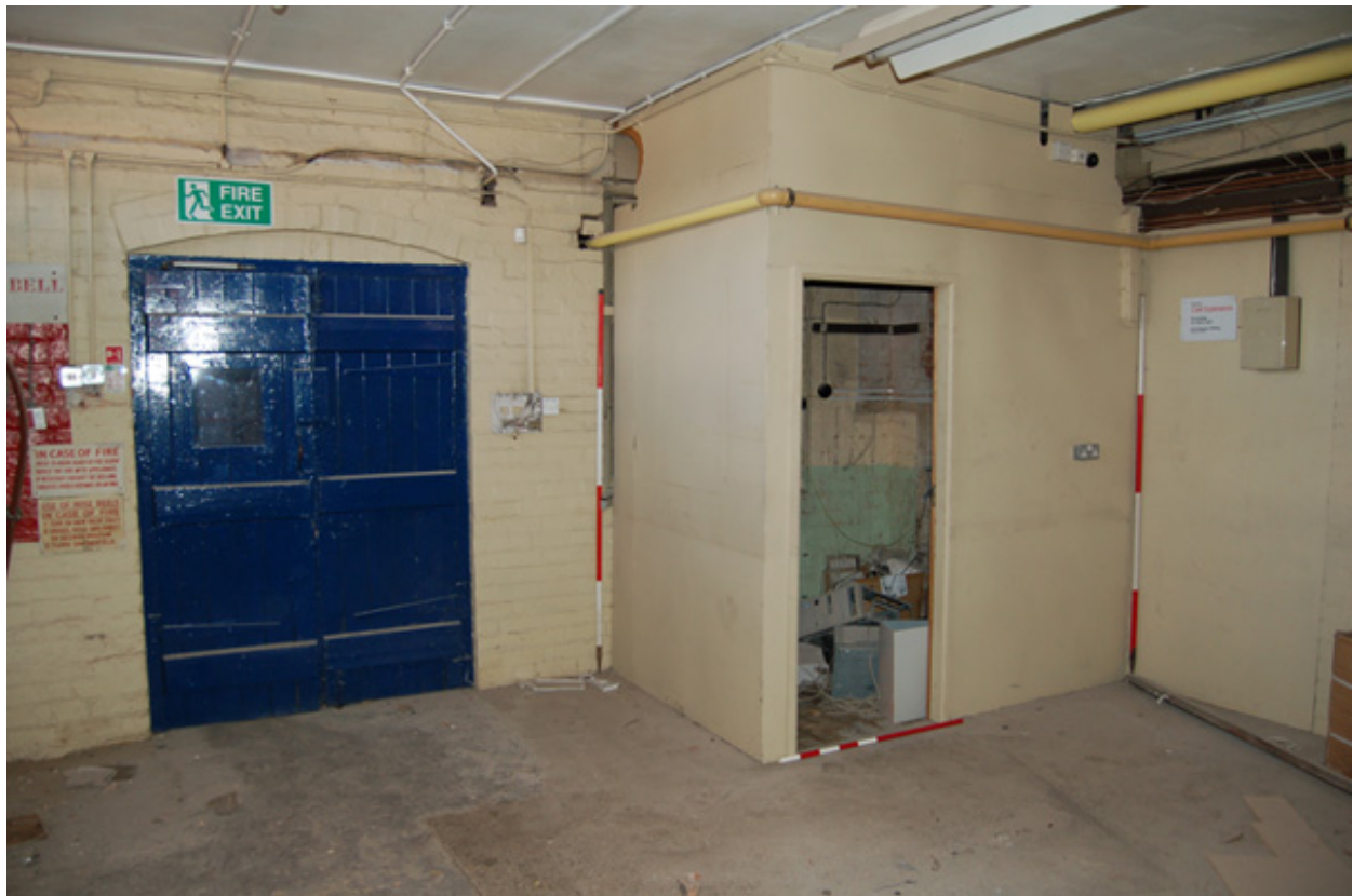
Plate 23: Room G12, looking south-east.
