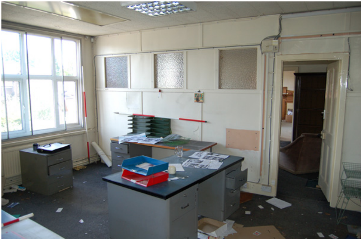
Plate 32: Room F5, looking south-west.
