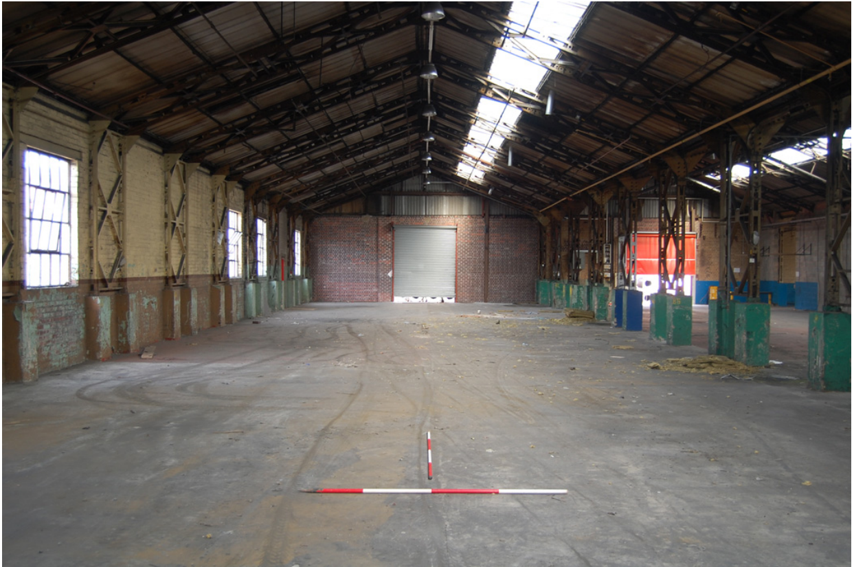
Plate 73: Building 28, Range 1; interior view looking west.
