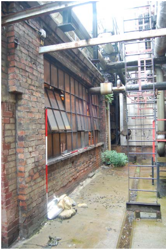
Plate 17: Building 8, east elevation looking N.
