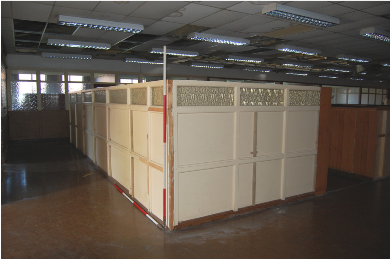
Plate 07: Building 1, interior: early partitioning.
