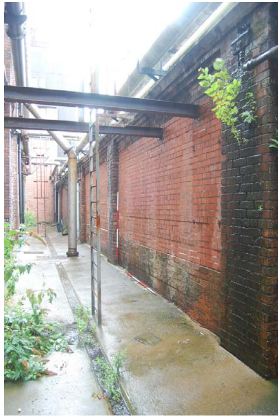
Plate 18: Building 8; east elevation looking S.
