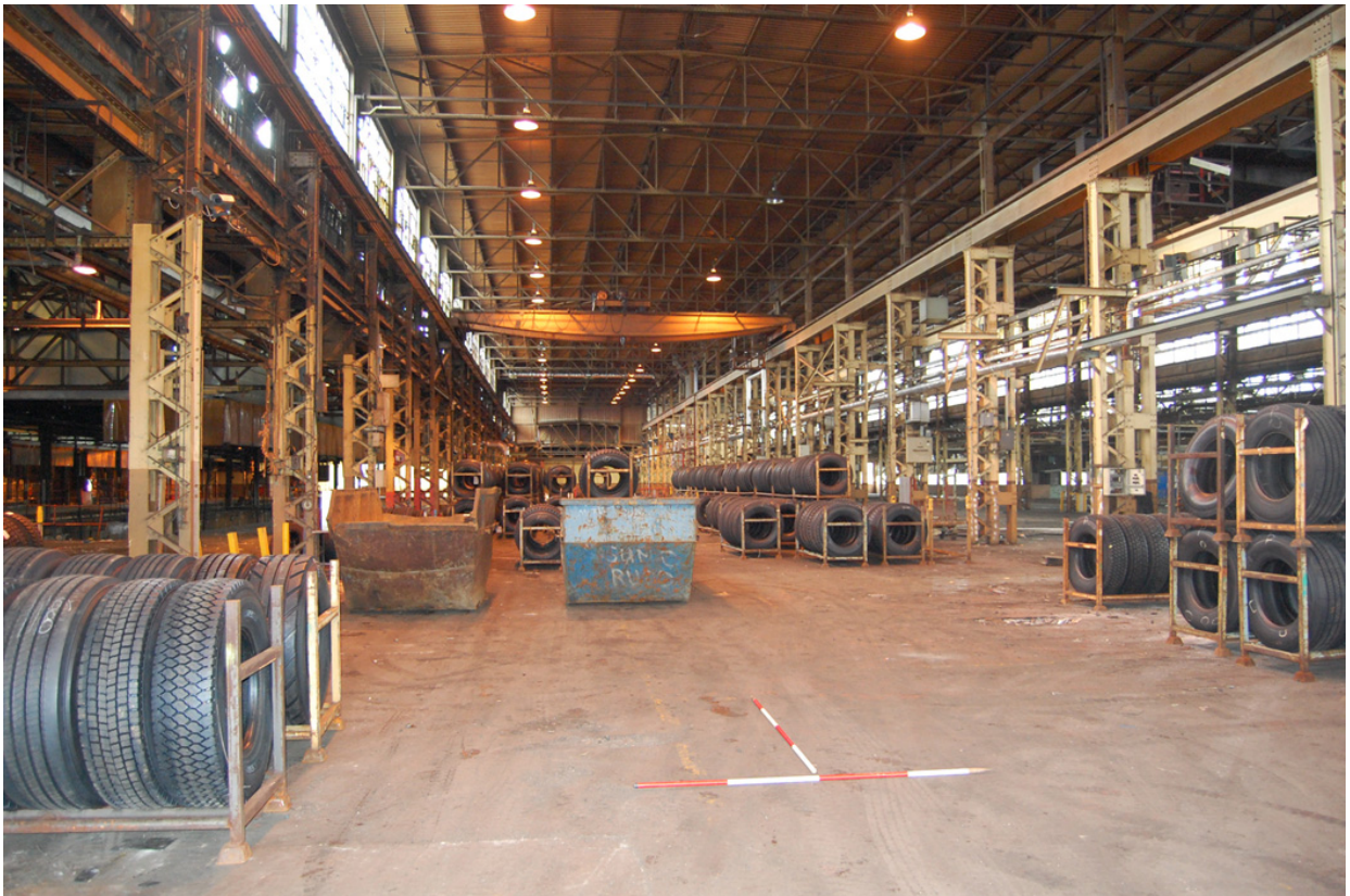
Plate 62: Building 18; interior, Range 9 (double height), looking south.
