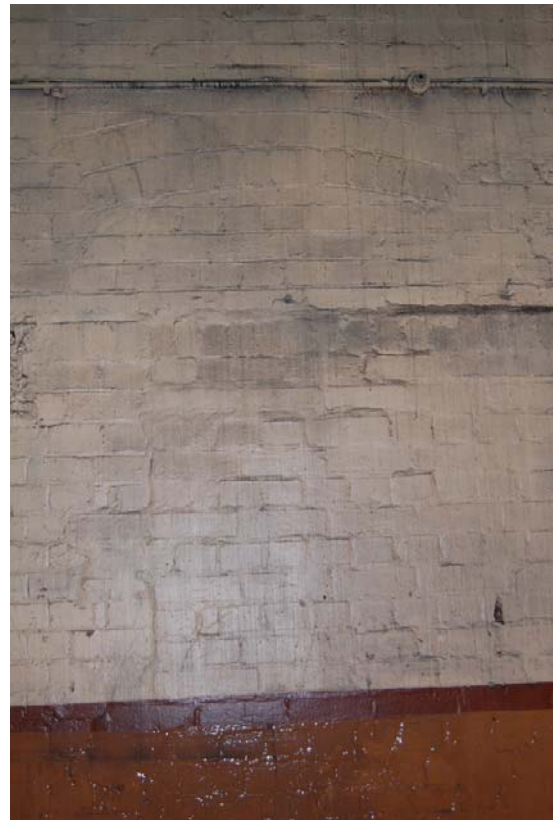
Plate 22: Blocked segmental headed window.
