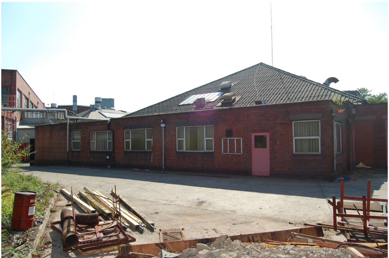
Plate 04: Building 1, north-east elevation.
