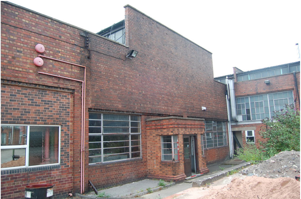
Plate 48: Building 12, exterior, south elevation with porch.
