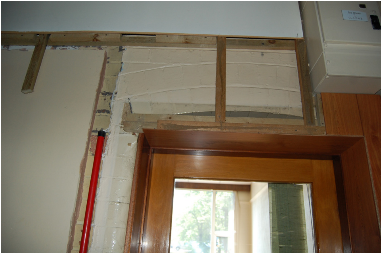
Plate 08: Building 1, interior: segmental arch over G1 door.
