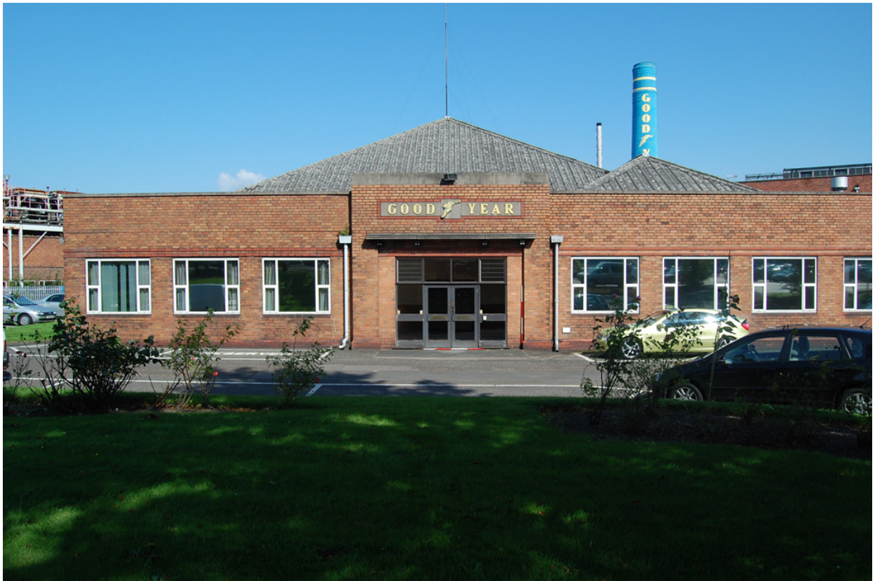
Plate 01: Building 1, south-west elevation.
