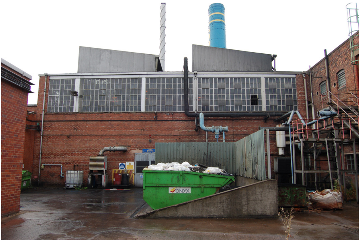
Plate 66: Building 22, exterior view from the north.
