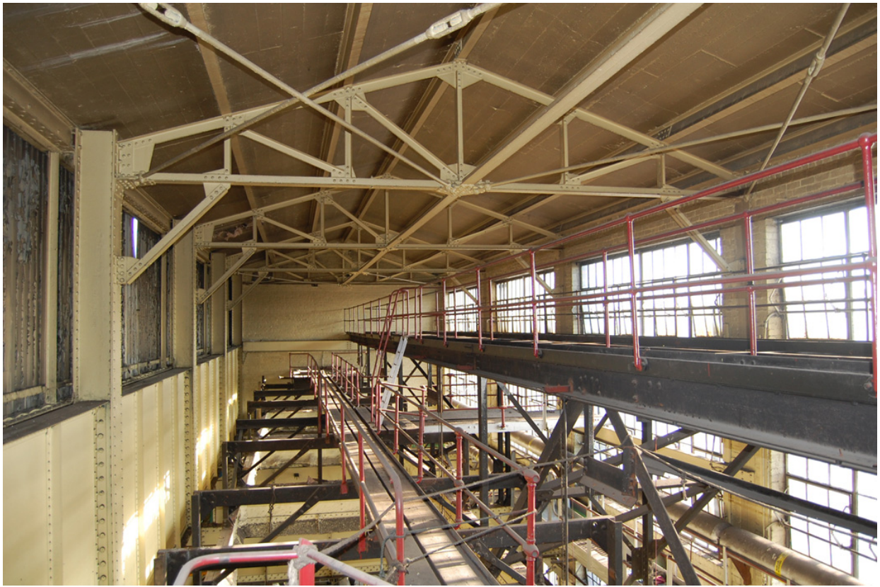
Plate 35: Building 21A; Roof structure over Bays 4 – 7.
