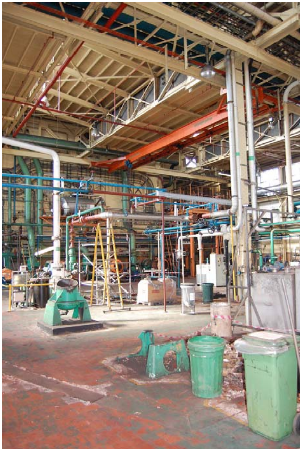
Plate 68: Building 22; interior view looking SE.
