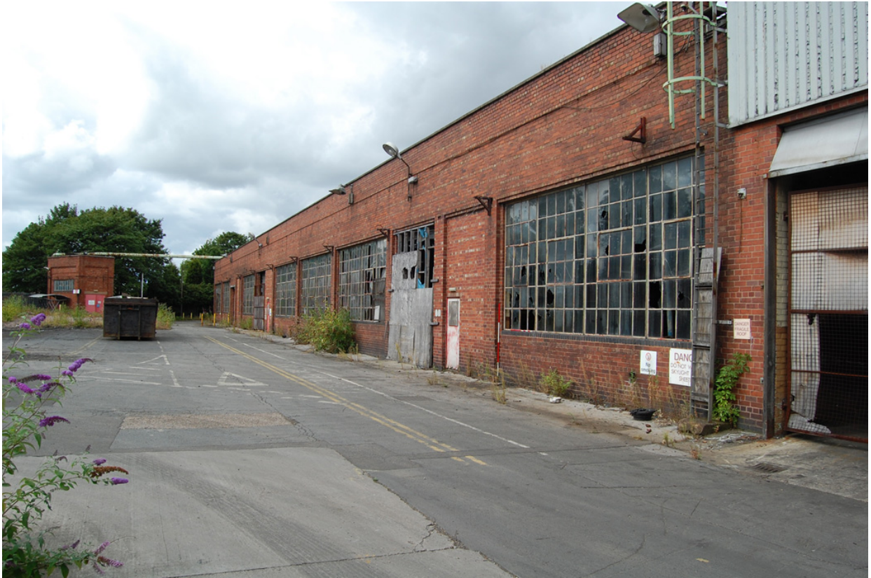
Plate 83: Building 44; south elevation, west (Ranges 4 – 8).
