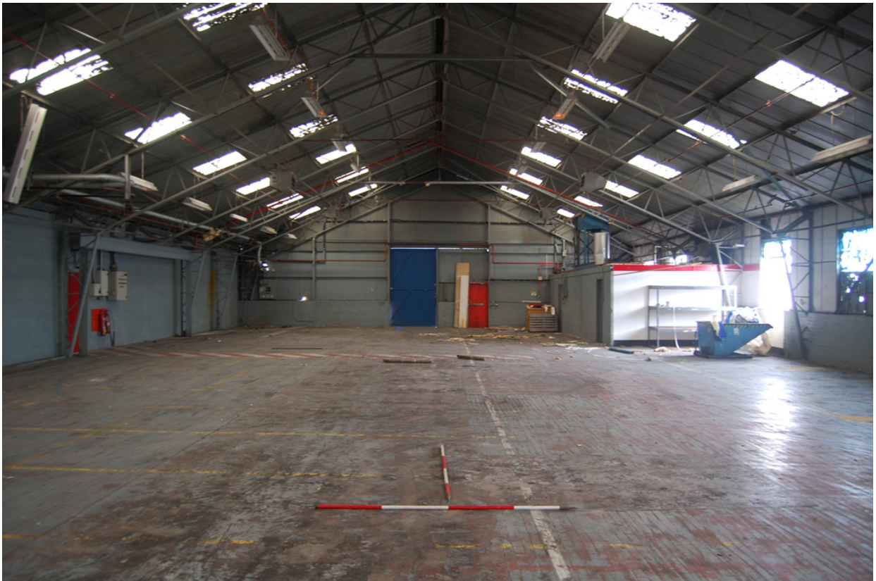
Plate 95: Building 45, west range looking south.
