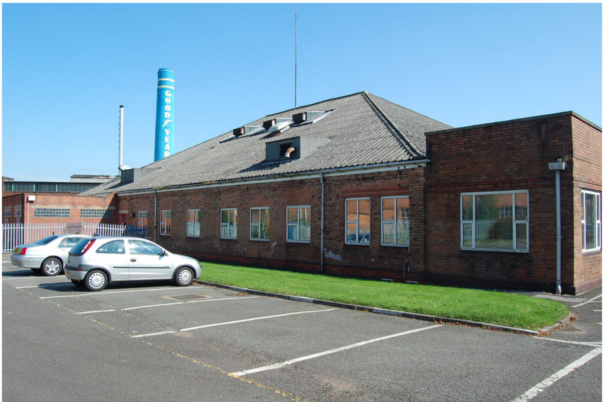
Plate 02: Building 1, north-west elevation.
