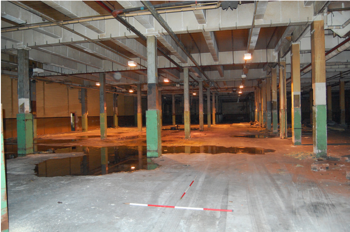
Plate 91: Building 44; south block, level 2 interior looking south.
