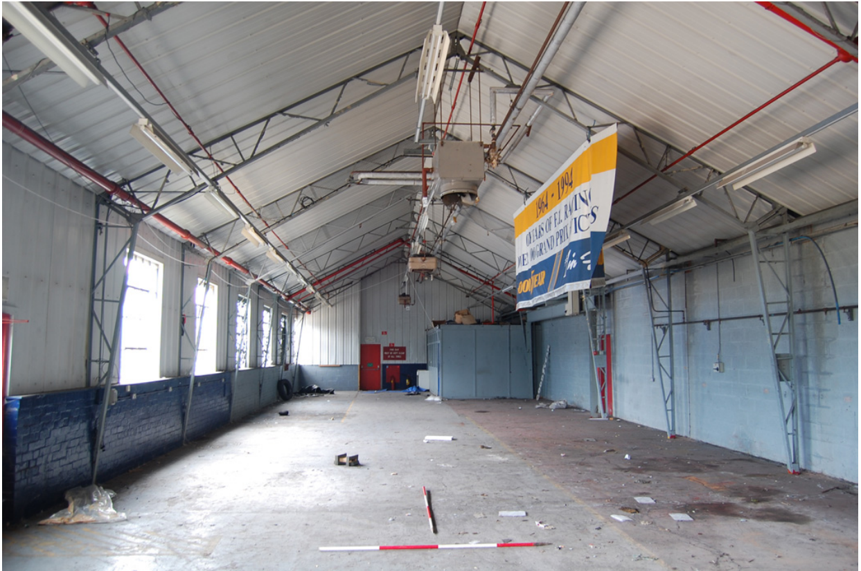
Plate 94: Building 45, east range interior looking south.
