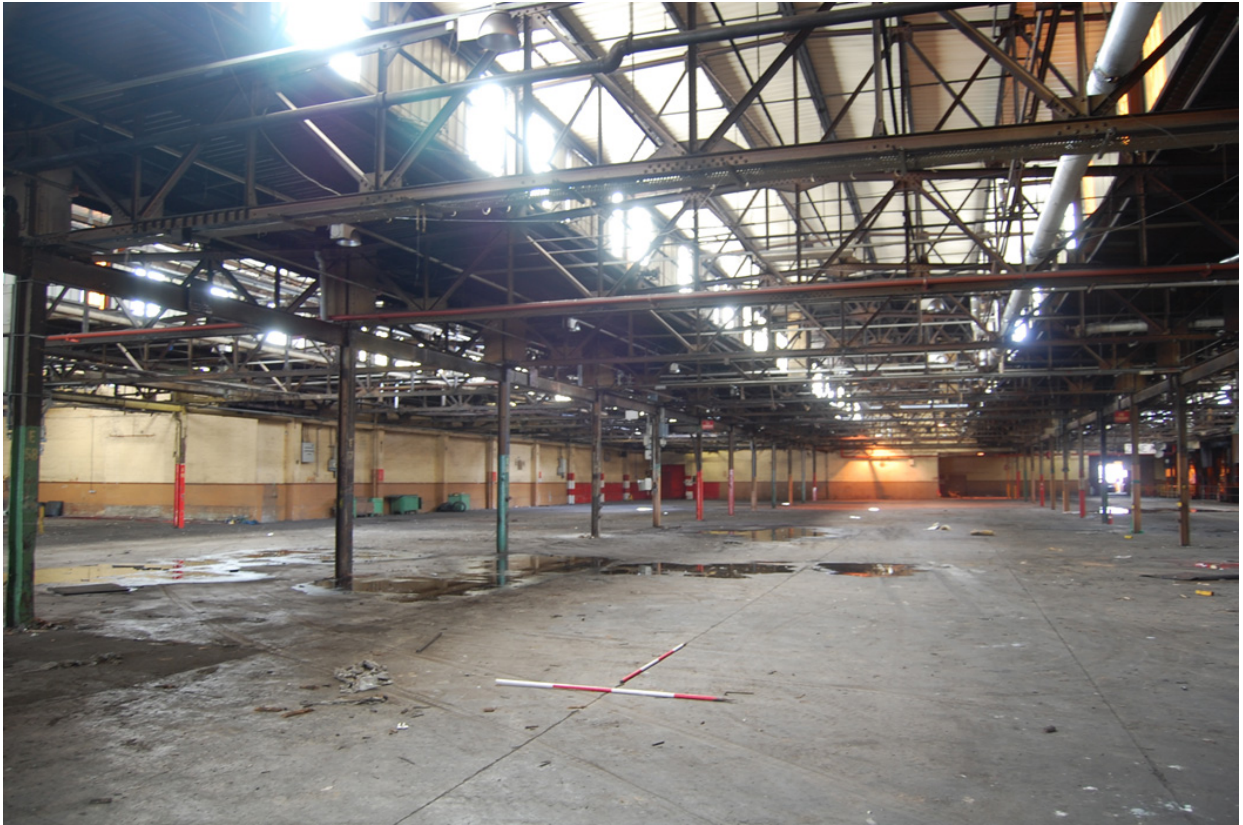
Plate 49: Building 12, interior Range 4 looking south.
