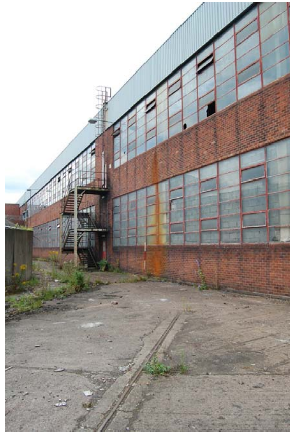
Plate 86: Building 44, south block, E elevation.
