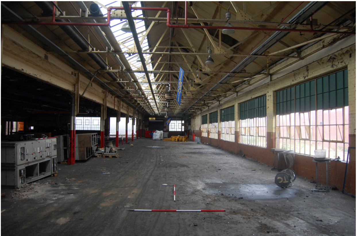
Plate 46: Building 11; east range interior view looking north.
