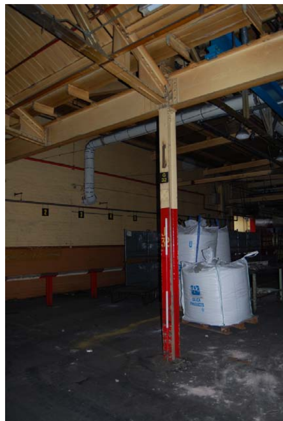
Plate 16: Building 8, western support column.
