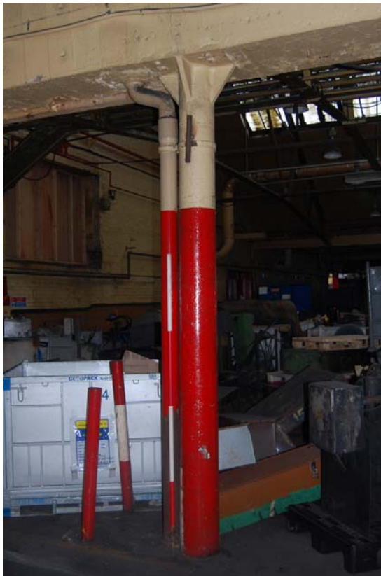
Plate 15: Building 8, central support column.
