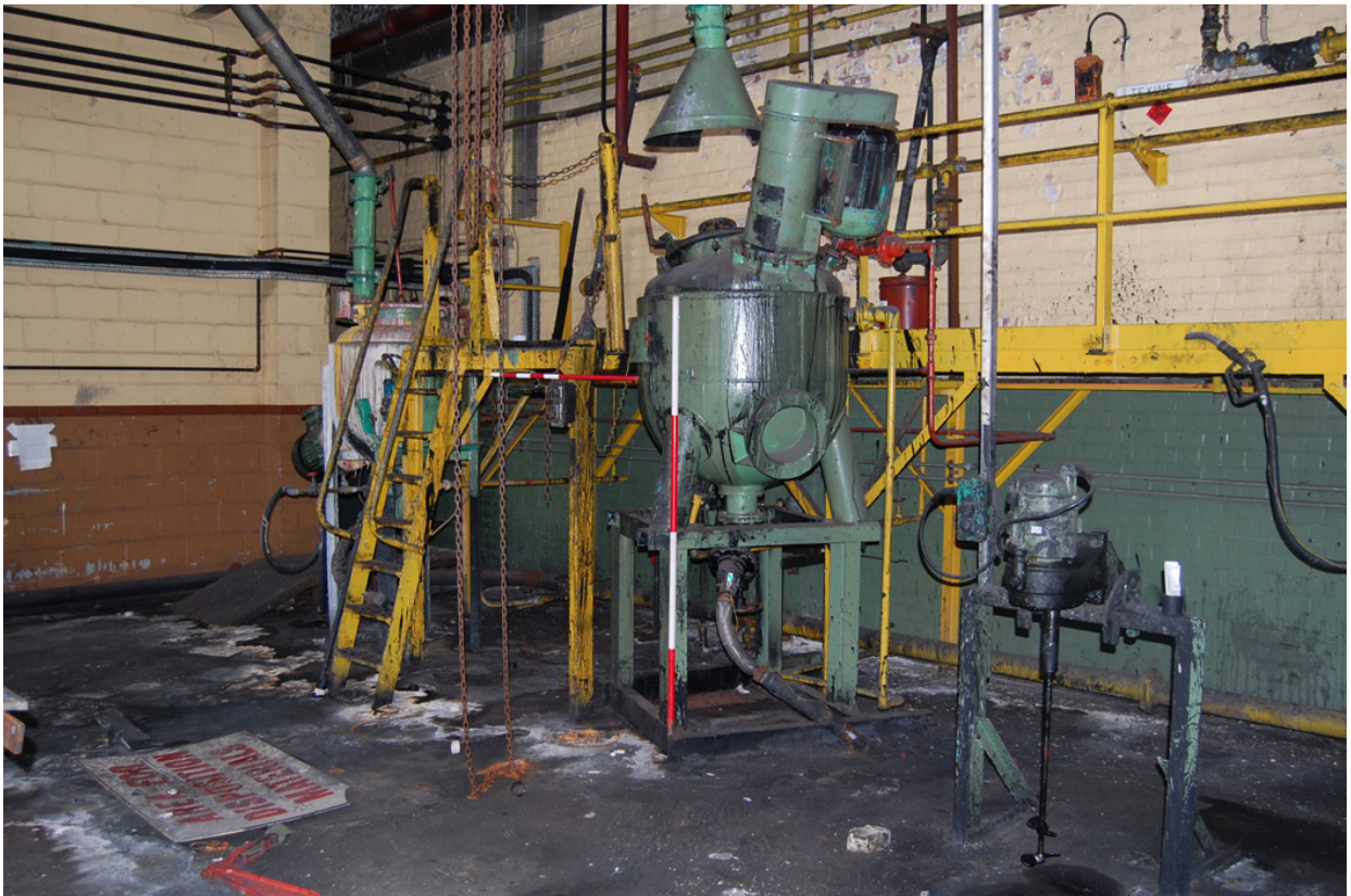
Plate 56: Building 17; Bay 13 'cement' machinery.
