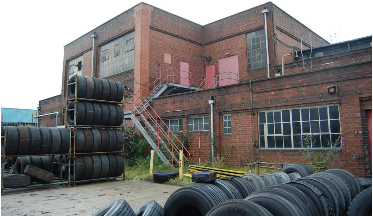
Plate 52: Building 17; 2-storey section from the north-east.
