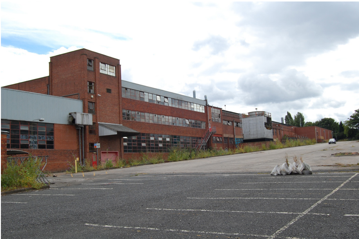
Plate 89: Building 44, south block west elevation, oblique view.
