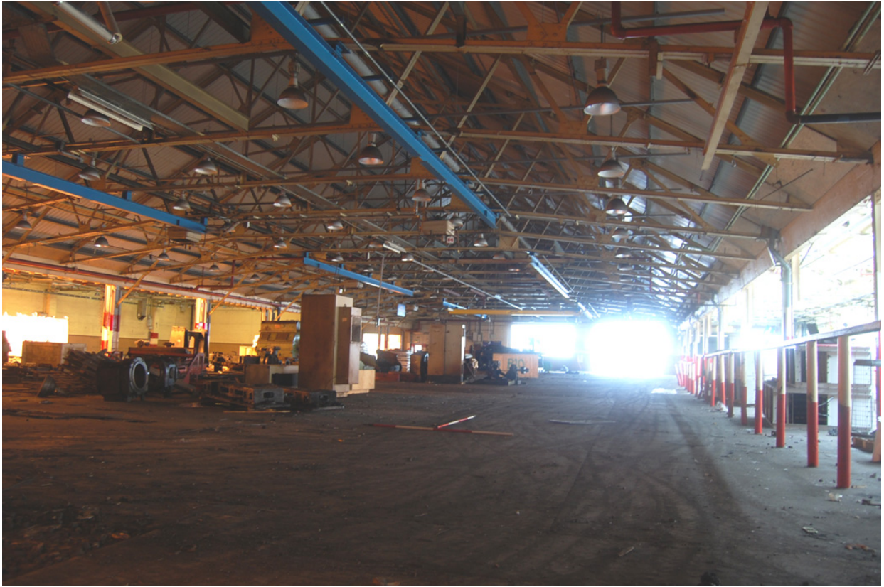
Plate 47: Building 11; west range interior view looking north.
