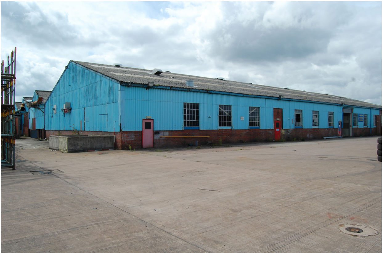
Plate 72: Building 28; exterior view from the north-east.
