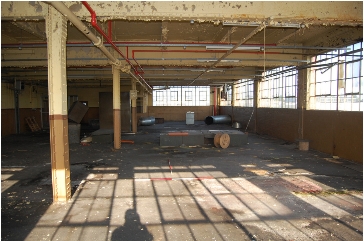
Plate 78: Building 29, first floor looking west.
