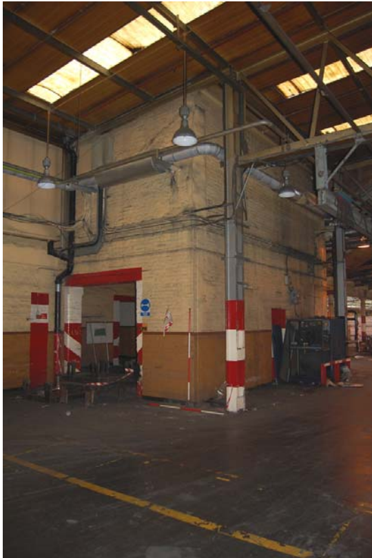
Plate 21: Building 9B, lower level walls.
