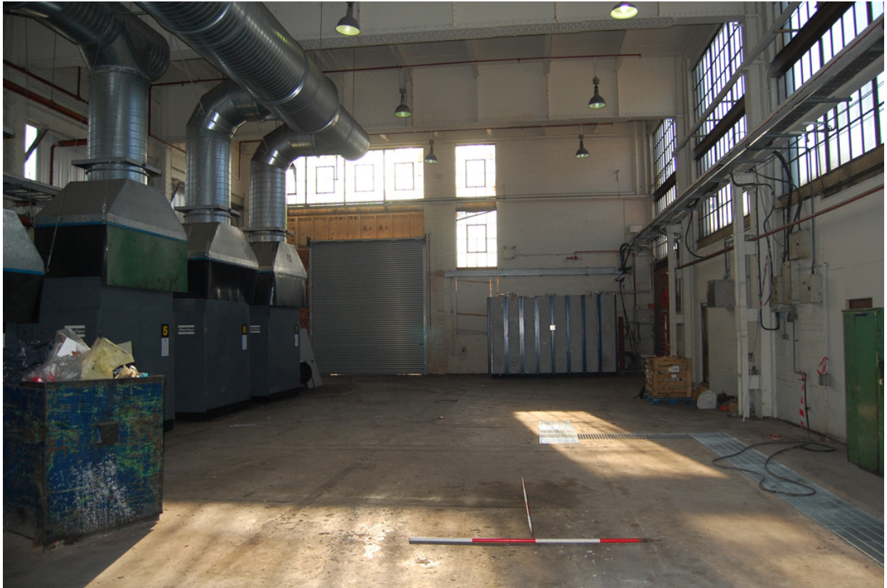
Plate 77: Building 29, Ground floor looking east.
