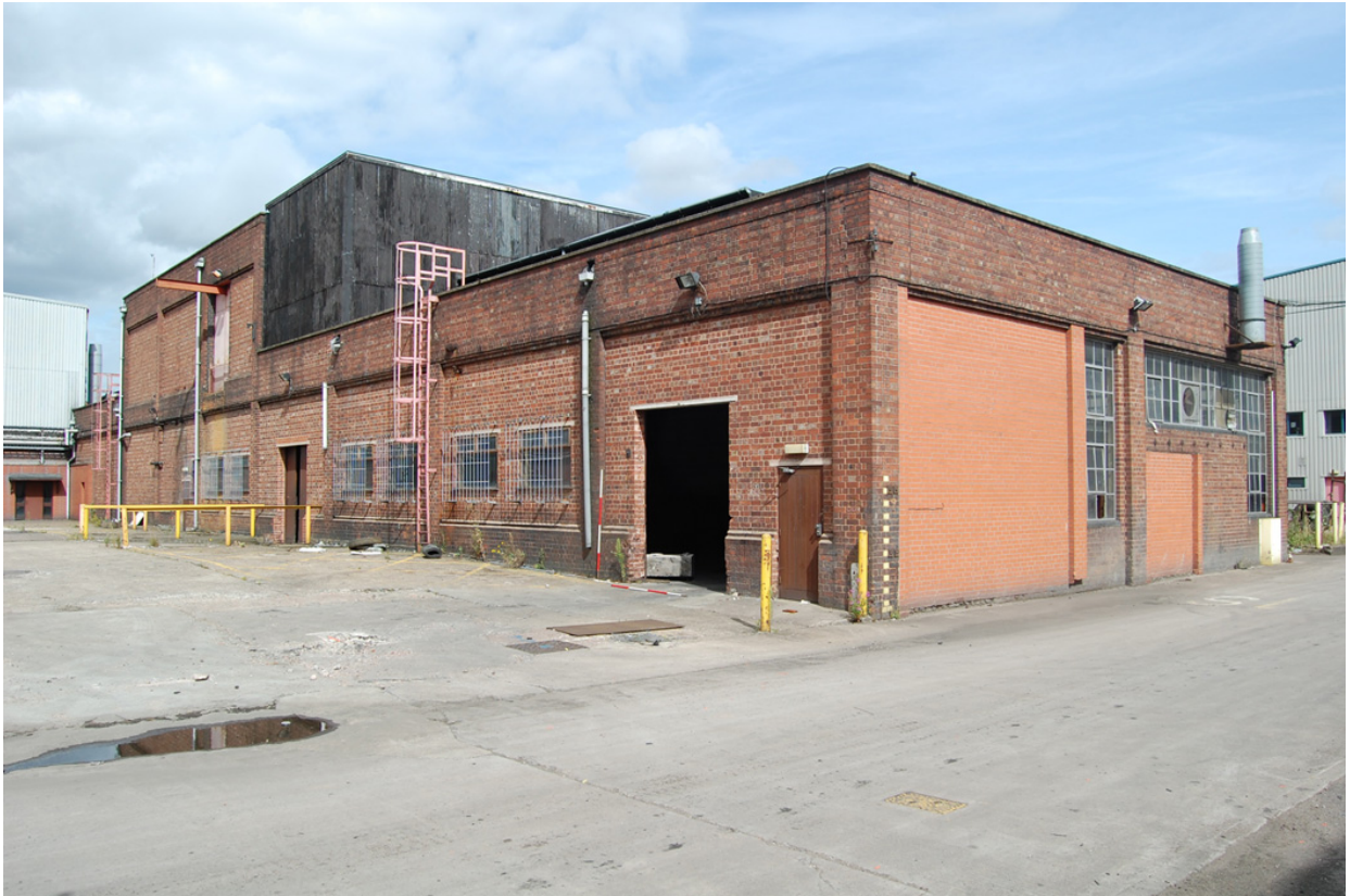
Plate 51: Building 17; exterior view from the south-west.
