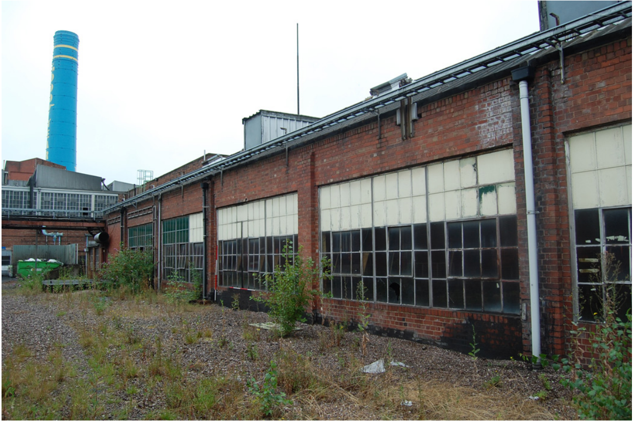
Plate 45: Building 11, exterior view from the north-east.
