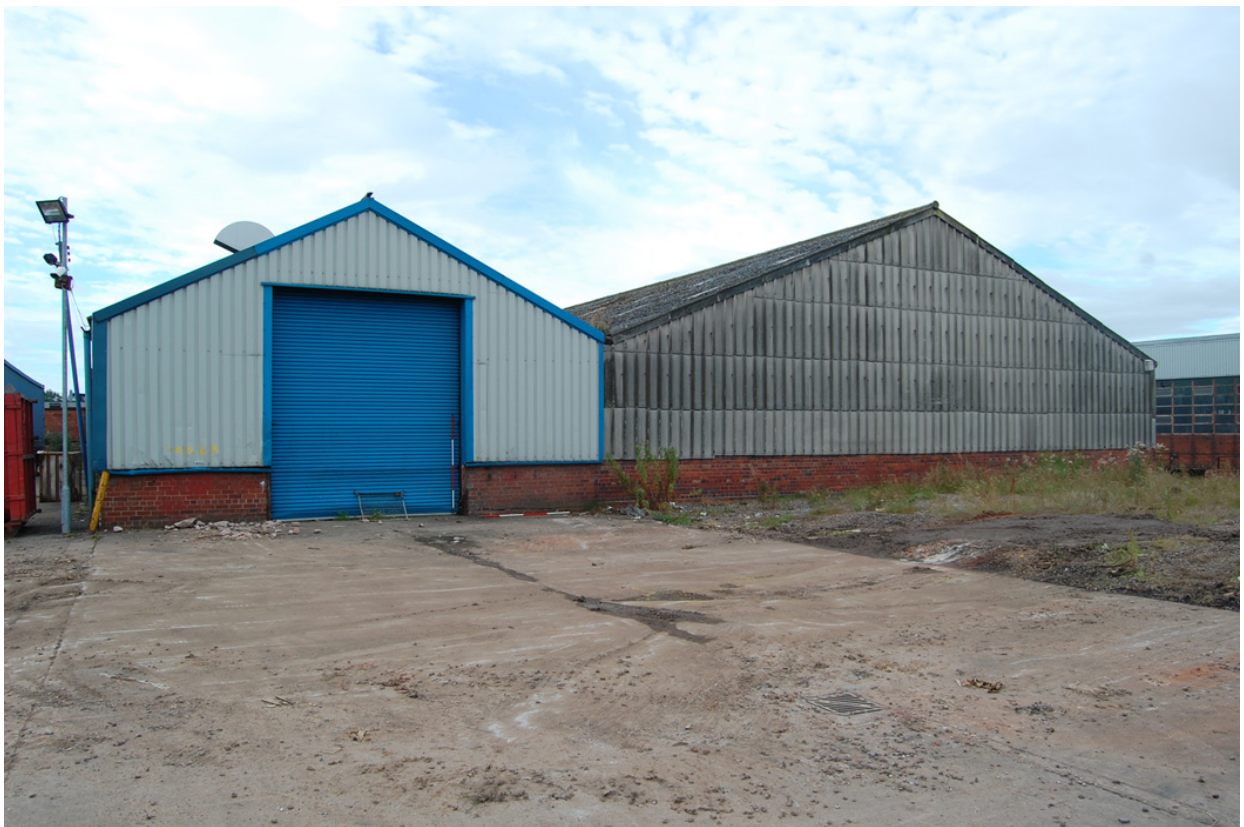
Plate 93: Building 45, north gable elevation.
