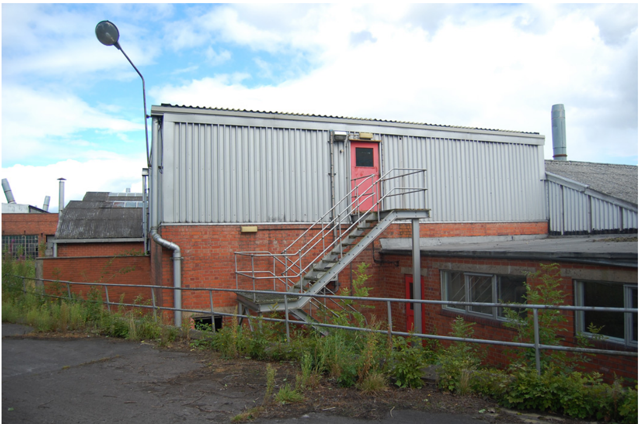
Plate 82: Building 31/75; exterior view, infill buildings at south-west corner.
