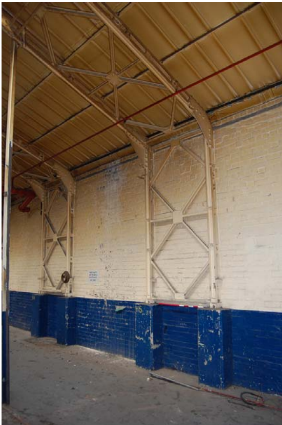
Plate 74: Building 28, detail of 'Bailey' construction.
