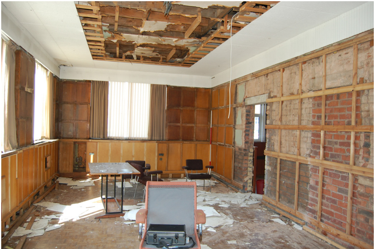
Plate 05: Building 1, interior; front office range (G4).
