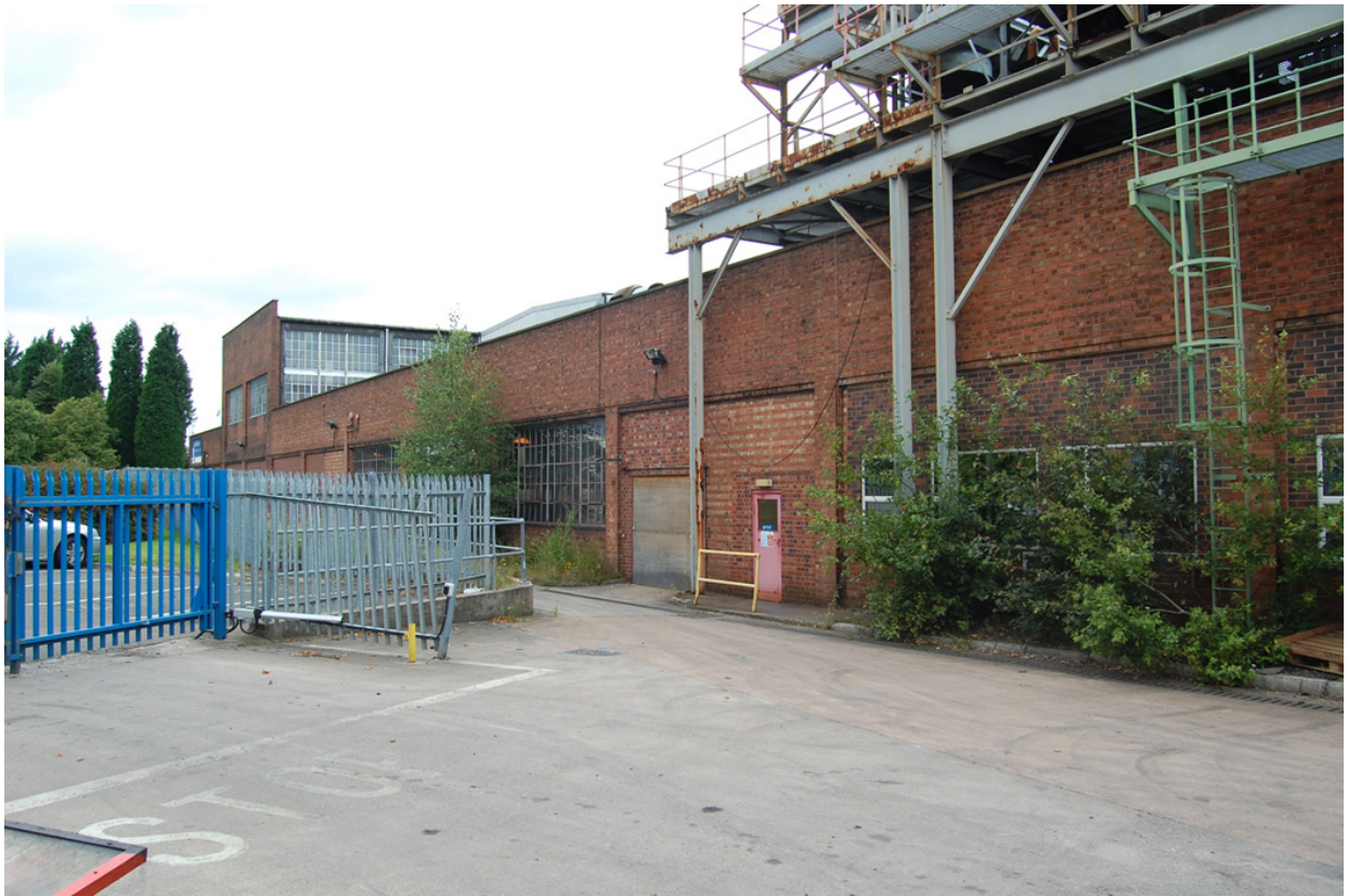
Plate 59: Building 18; south elevation oblique view.
