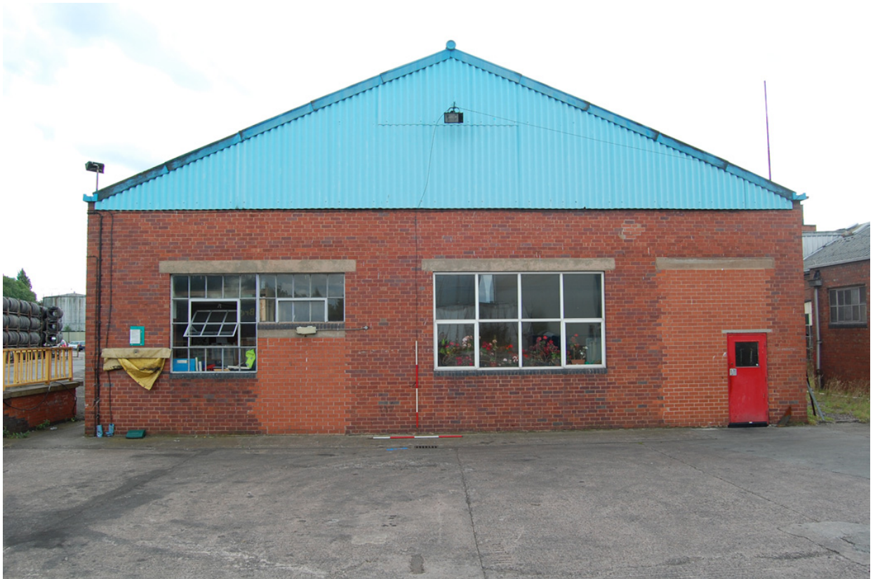
Plate 97: Building 82, north gable elevation.
