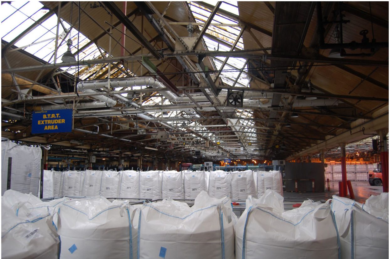
Plate 12: Building 8; west range looking north.
