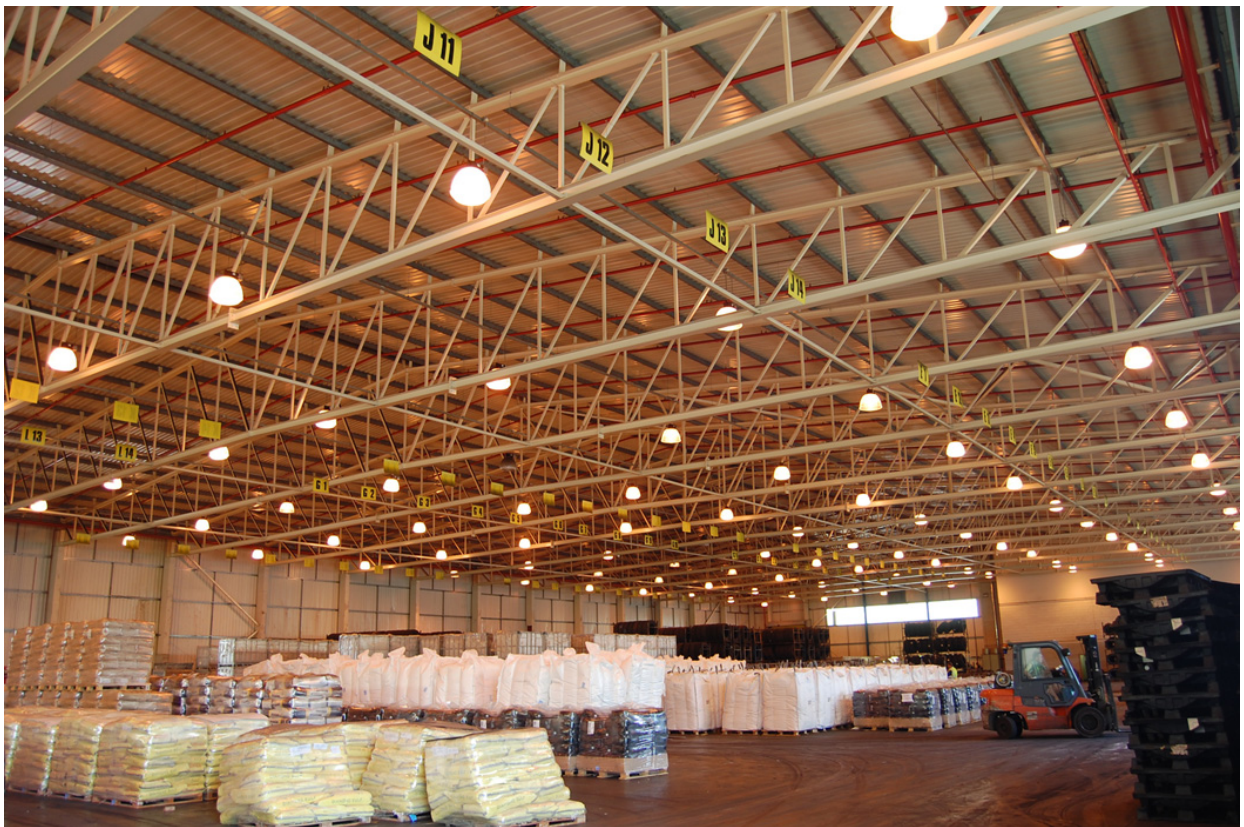
Plate 58: Building 13; interior view looking west.
