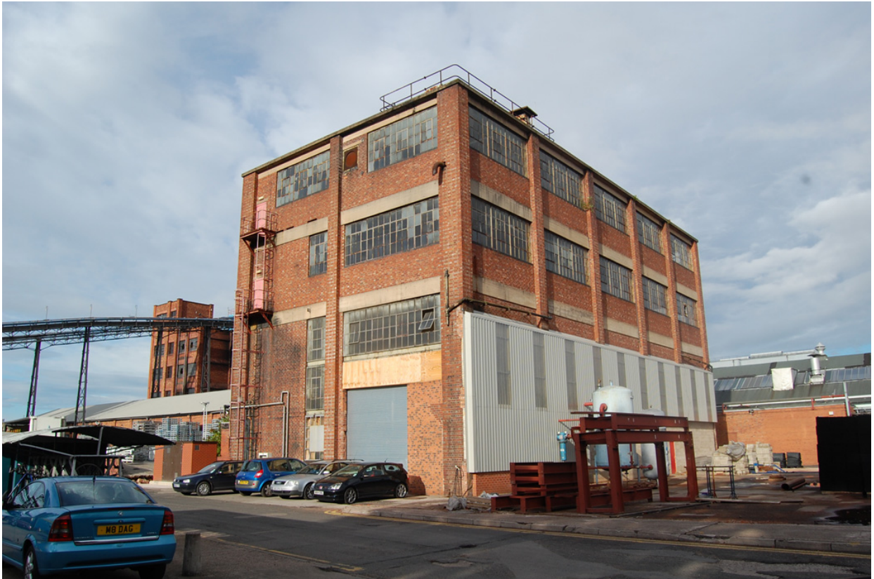
Plate 75: Building 29, exterior view from the north-east.
