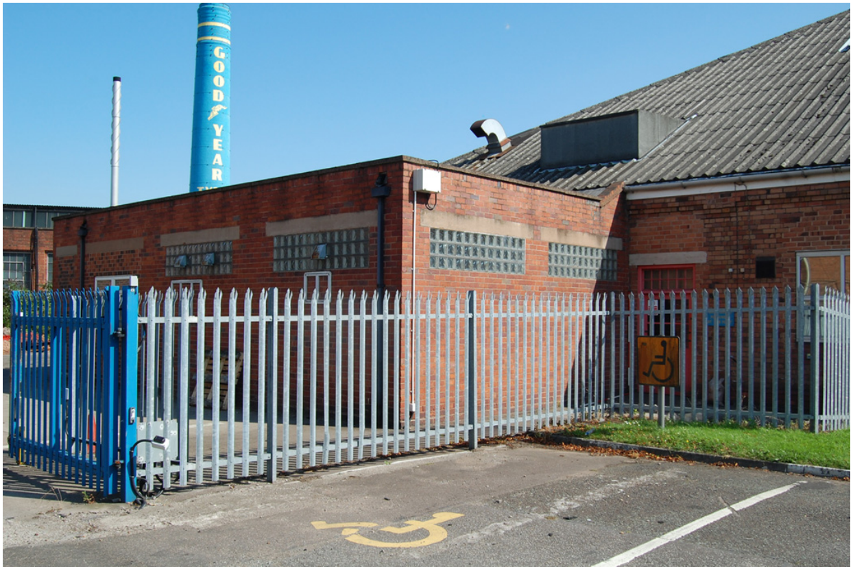
Plate 03: Building 1, north-west extension (boiler house chimney in background).
