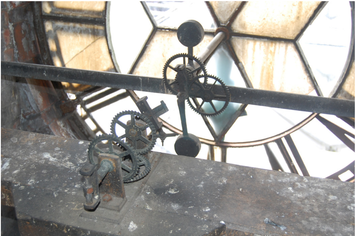
Plate 26: Building 9B; surviving clock mechanism at Level 4.
