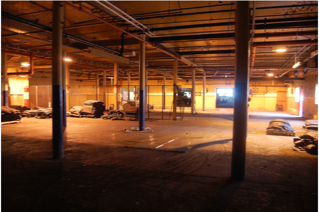
Plate 30: Building 10; interior, ground floor looking north.
