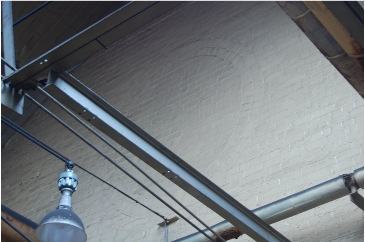
Plate 14: Building 8; east range south elevation gable, blocked circular opening.
