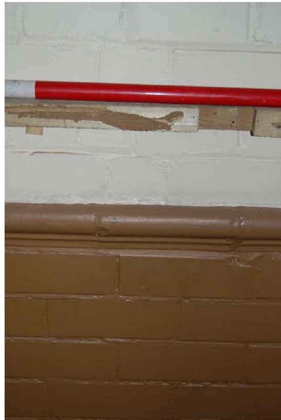
Plate 10: Detail of moulded brick dado.
