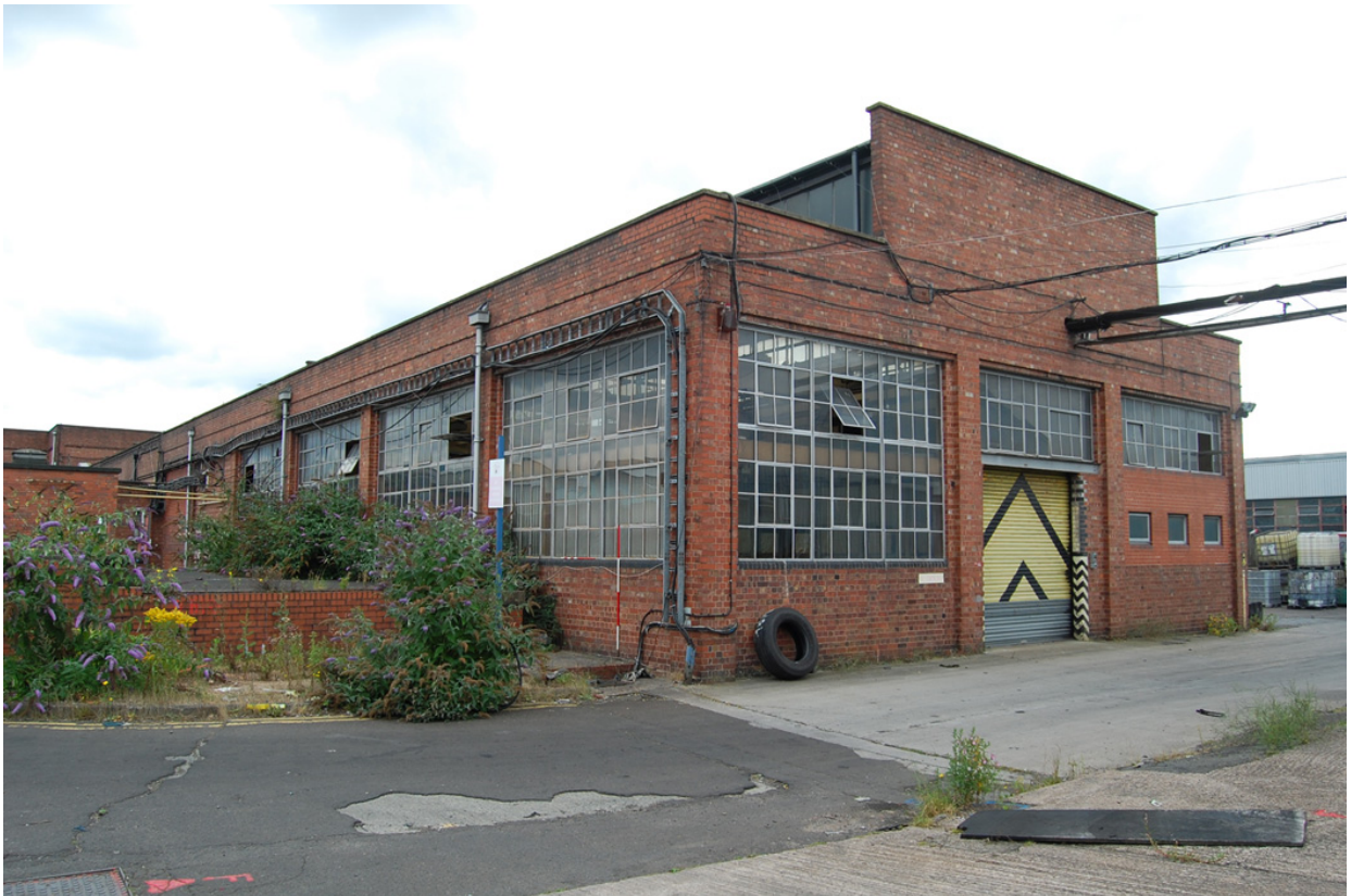
Plate 50: Building 17; exterior view from the north-east.
