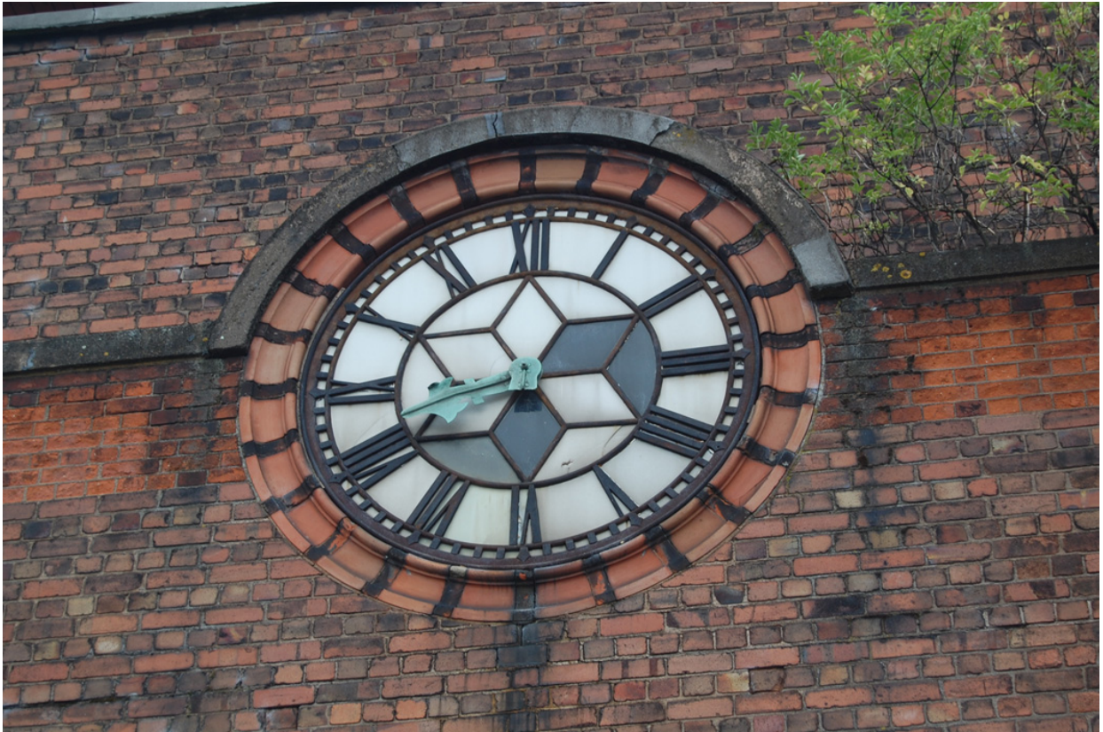
Plate 25: Building 9B; detail of clock (east elevation).
