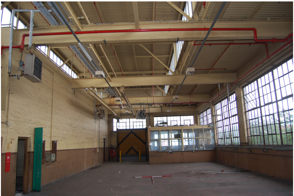
Plate 54: Building 17; interior, north end looking north.
