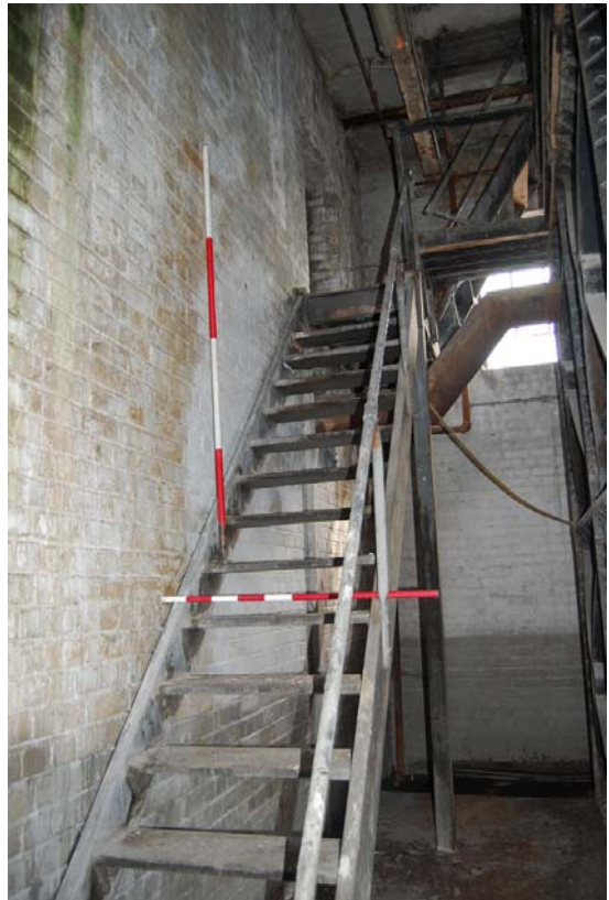
Plate 24: stair access, Levels 3 to 4.
