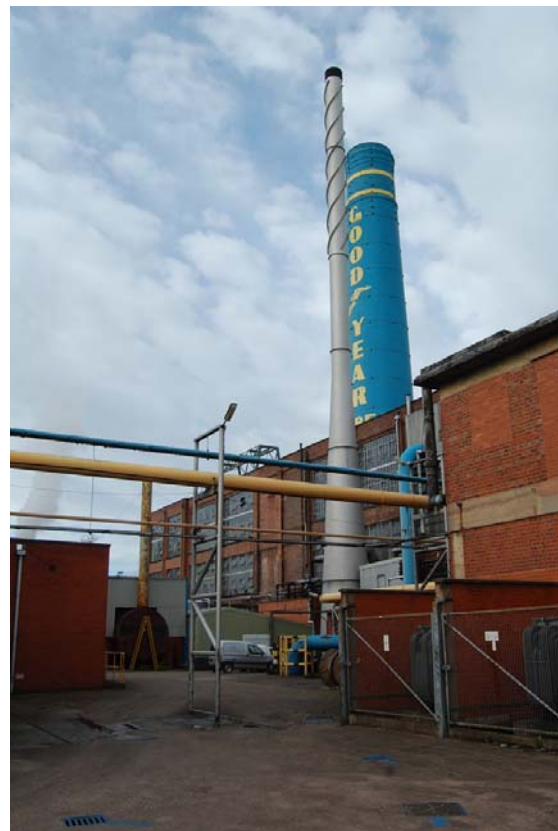
Plate 34: Building 21 from the north-east.
