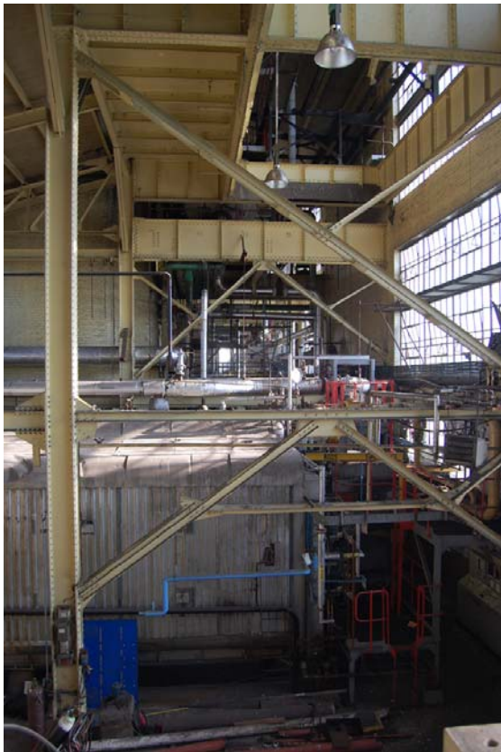
Plate 38: Building 21A; interior looking north.
