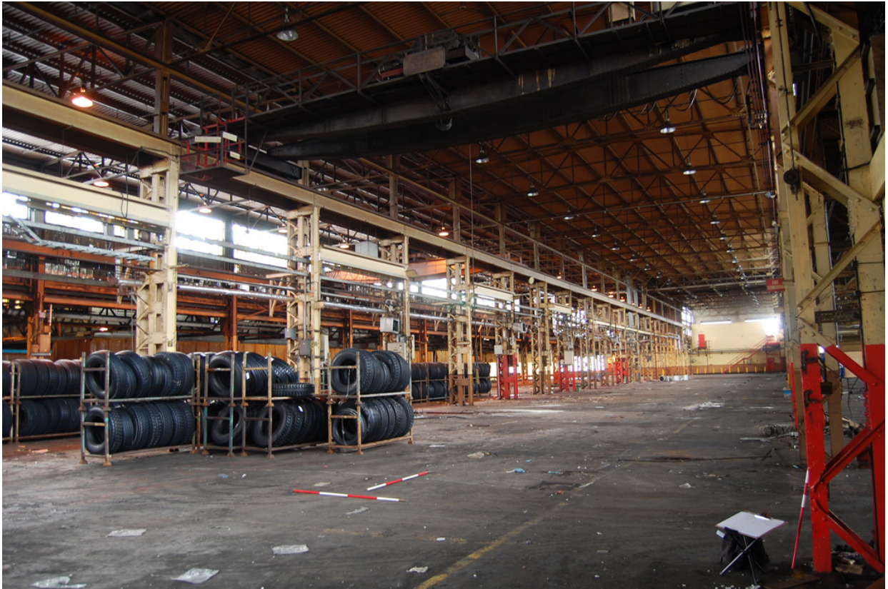
Plate 63: Building 18, Range 10 looking south-east.
