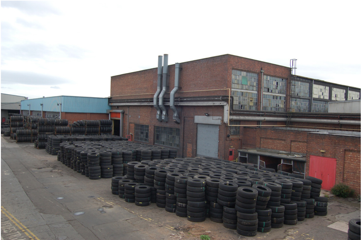
Plate 61: Building 18; north elevation.
