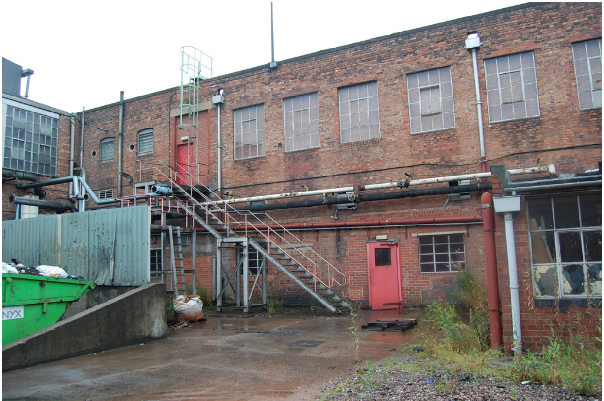
Plate 27: Building 10, east elevation.
