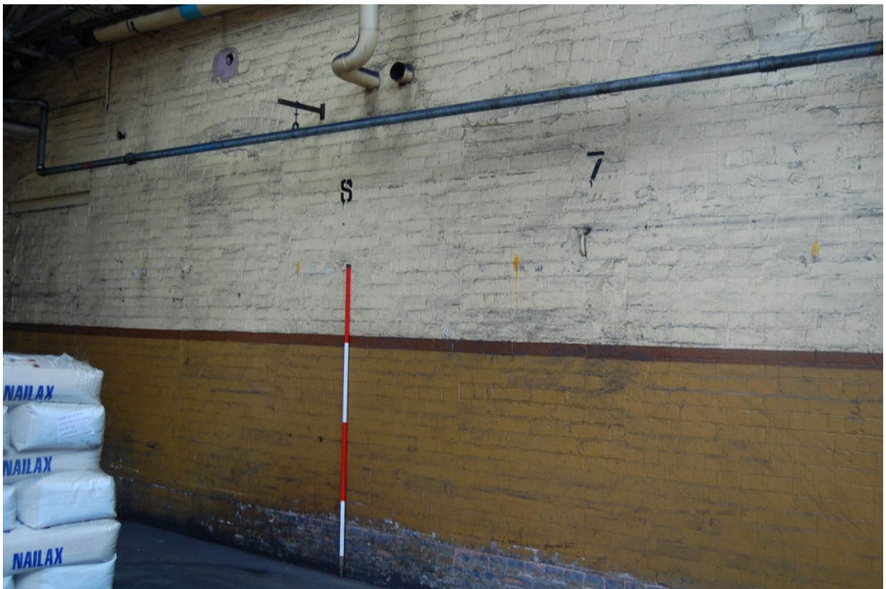
Plate 13: Building 8; east range south elevation, blocked segmental headed windows.
