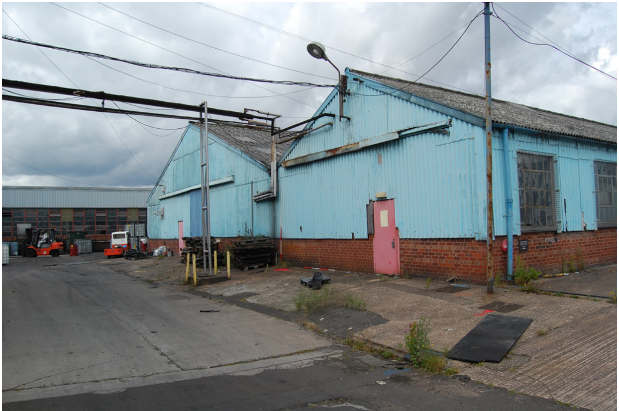
Plate 92: Building 45 south gable elevation.
