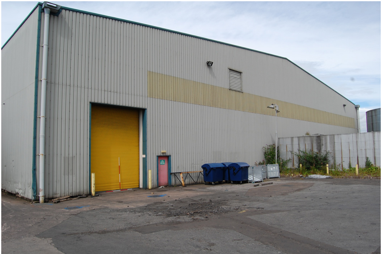
Plate 57: Building 13; eastern gable elevation.
