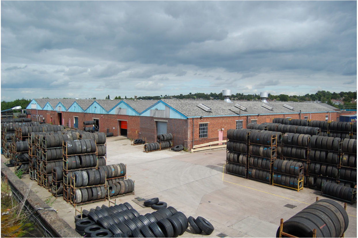
Plate 71: Building 28; exterior view from the south-west (from roof of Building 17).
