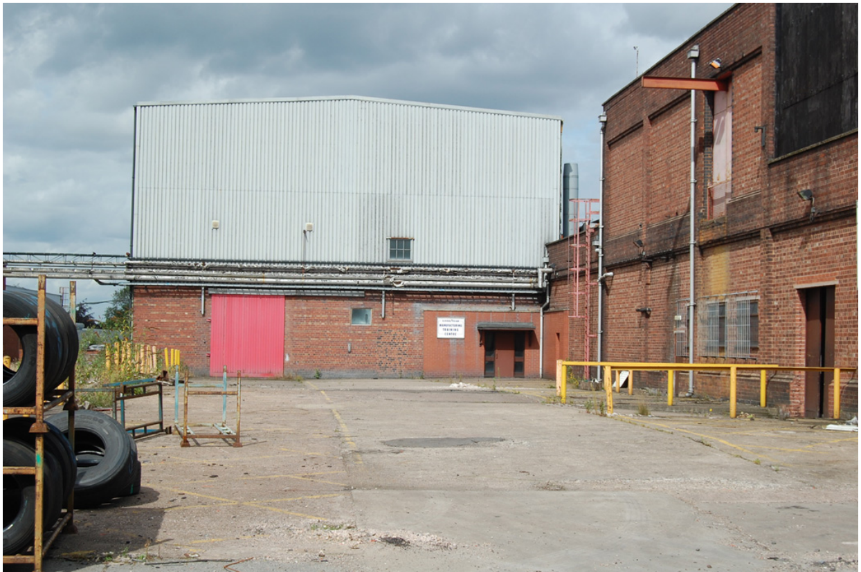
Plate 53: Building 17; 1970's western extension, from the south.
