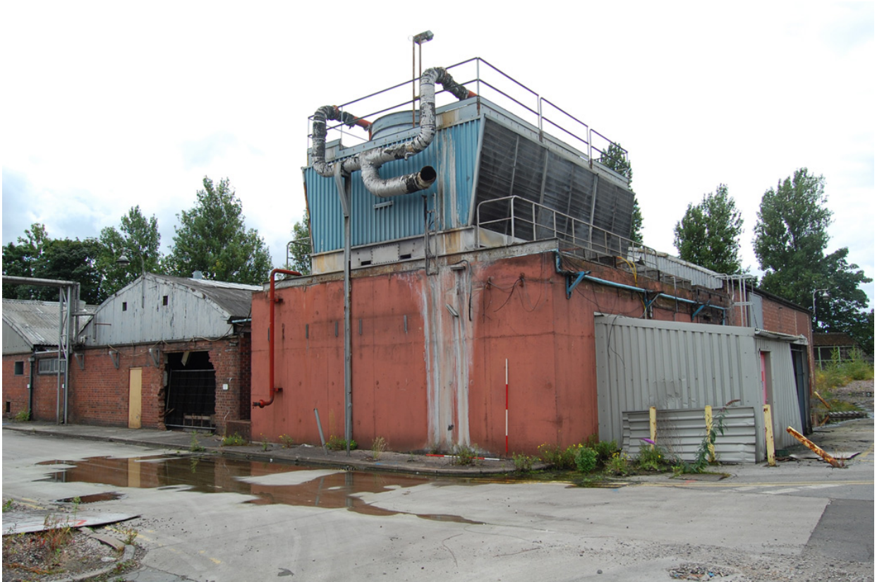
Plate 81: Building 31/75; exterior view from the north-east.
