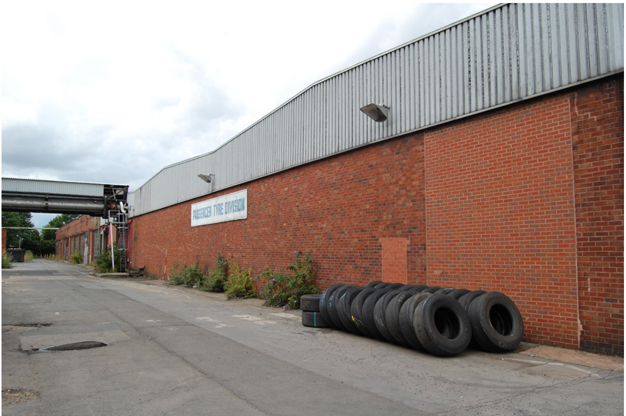
Plate 84: Building 44; south elevation, east (Ranges 1 – 3).
