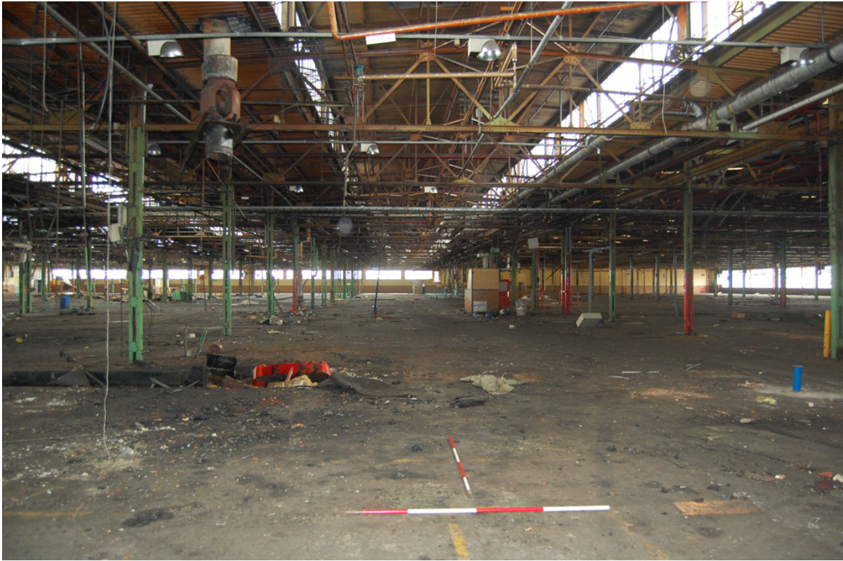
Plate 90: Building 44; south block, level 3 interior looking north.
