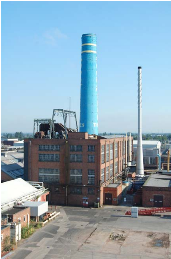
Plate 33: Building 21 from the south.
