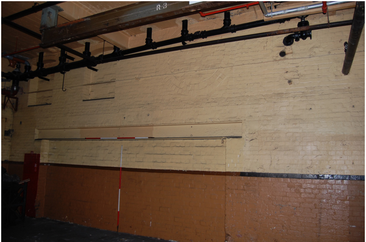
Plate 31: Building 10; south wall, blocked windows and circular vent.
