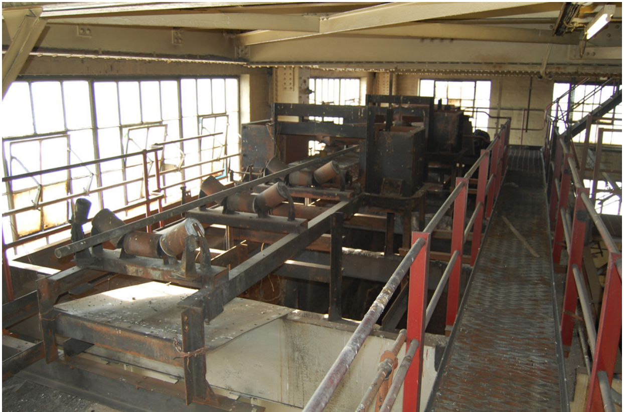
Plate 42: Building 21F; surviving section of conveyor system formerly feeding coal hoppers.
