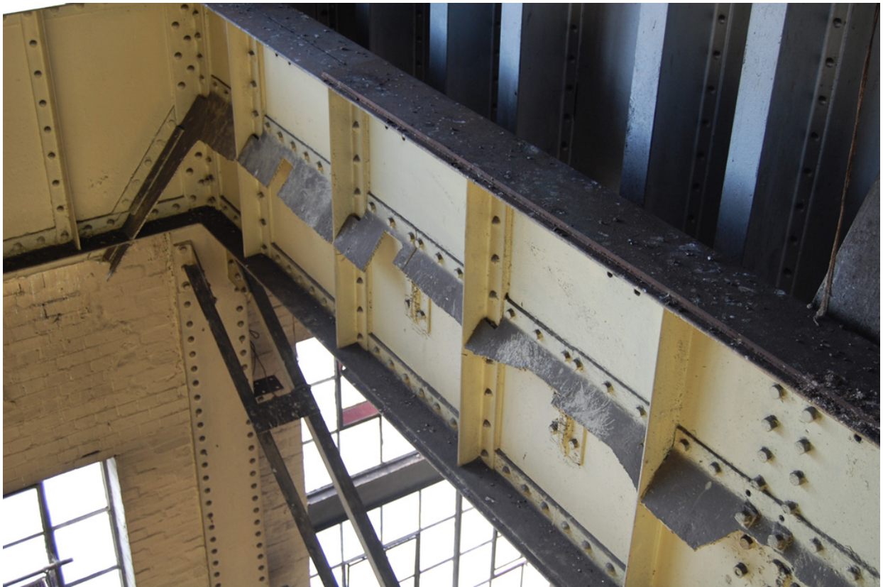
Plate 36: Building 21A: Evidence for former coal hoppers, Bay 2.
