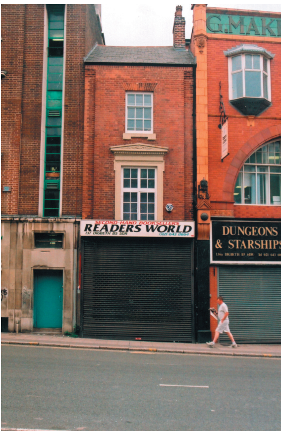
Plate 15. 137 Digbeth from southwest
