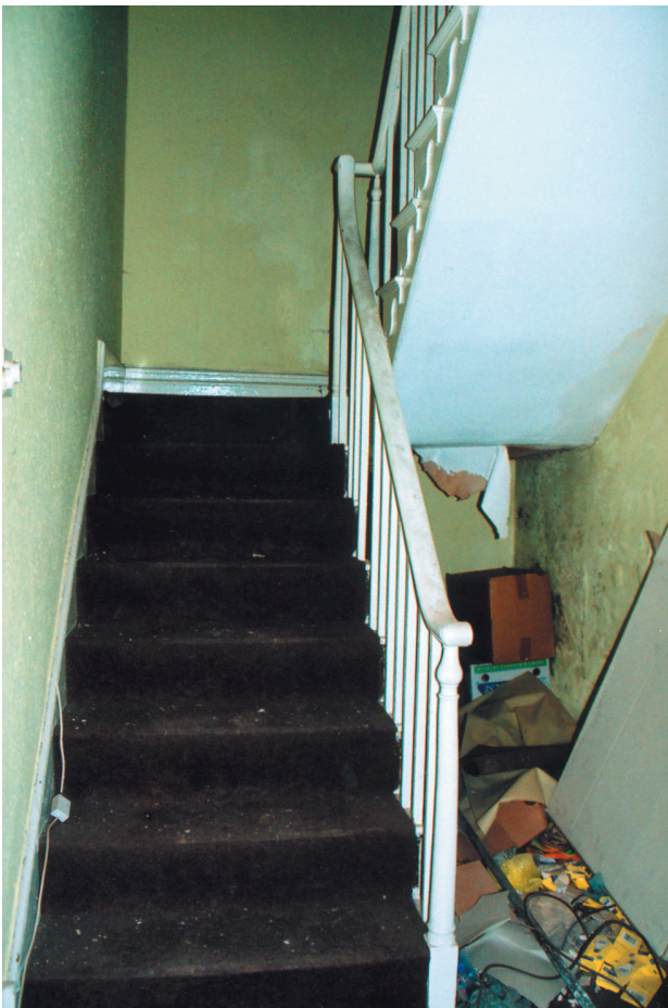
Plate 19. 140 digbeth, staircase from the east
