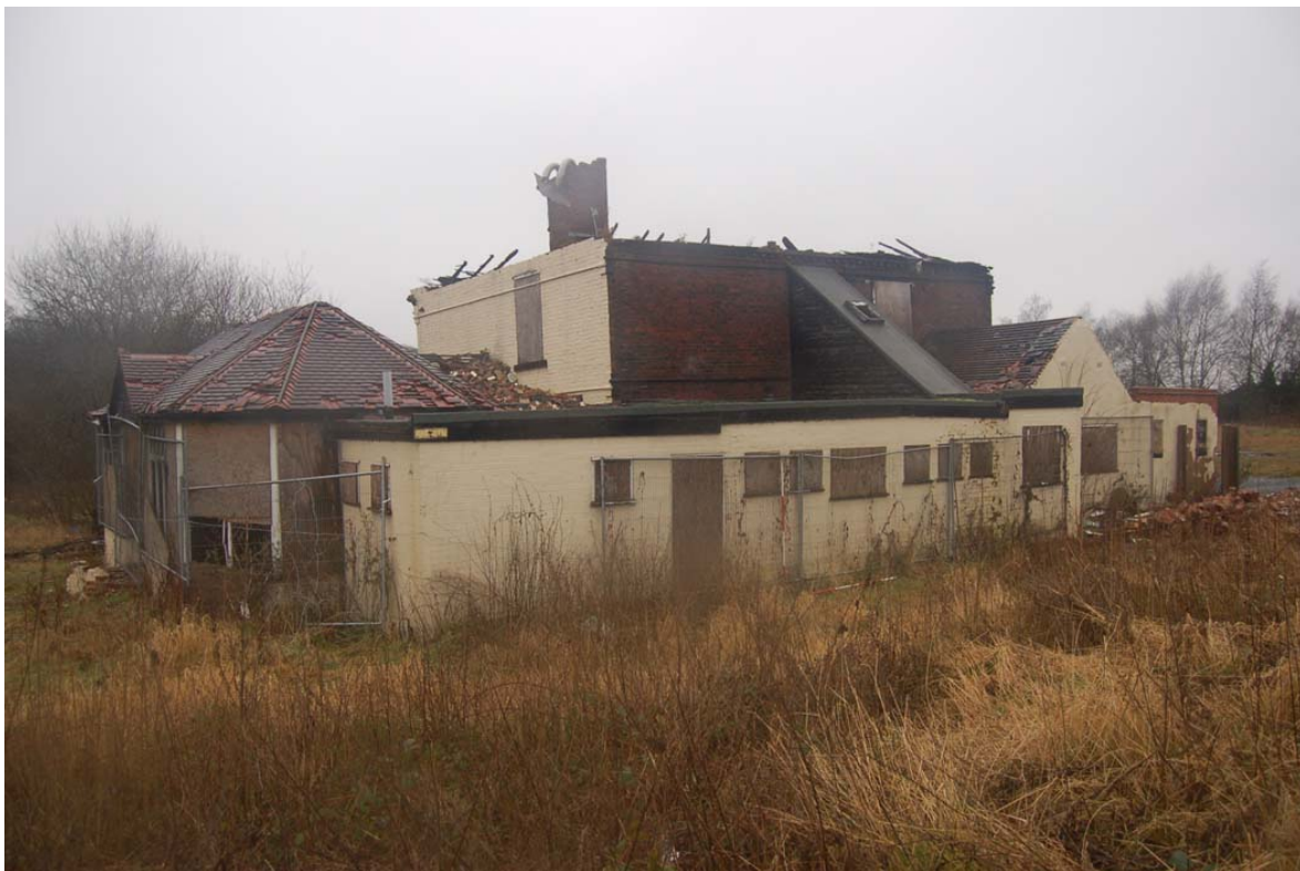
Plate 6: North-east elevation, oblique view.
