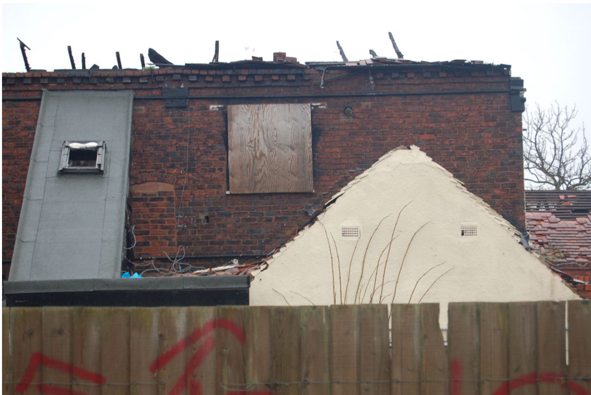
Plate 11: NE elevation, detail. Note blocked window to right of stair.
