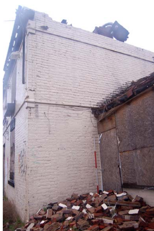
Plate 9: Rebuild of front wall (SE elevation).
