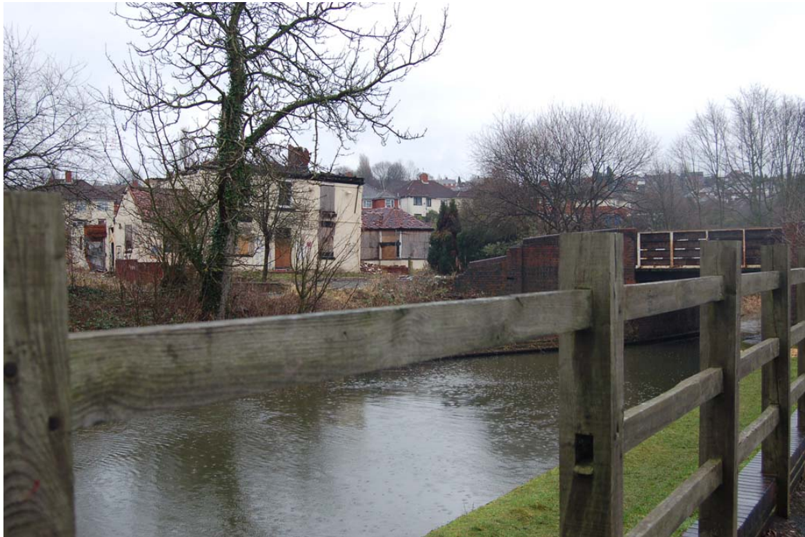
Plate 1: General view from the south-west. Dudley No.2 Canal in foreground.
