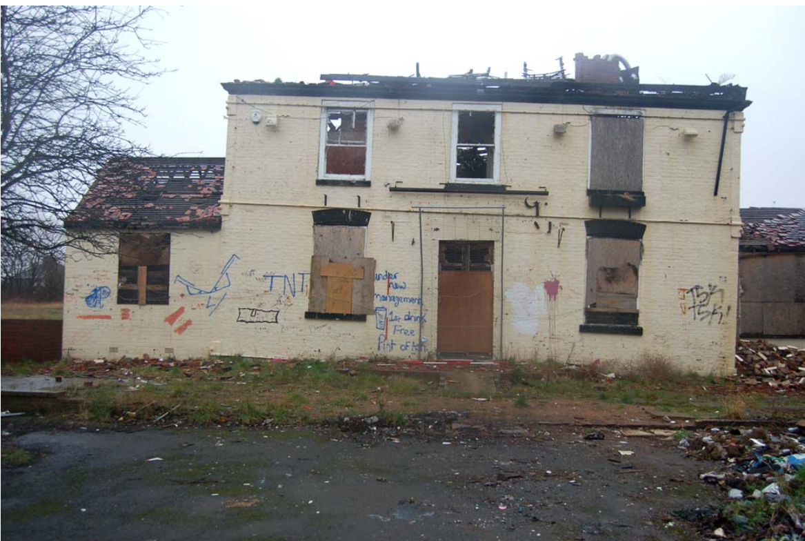
Plate 4: Main block, south-west elevation.
