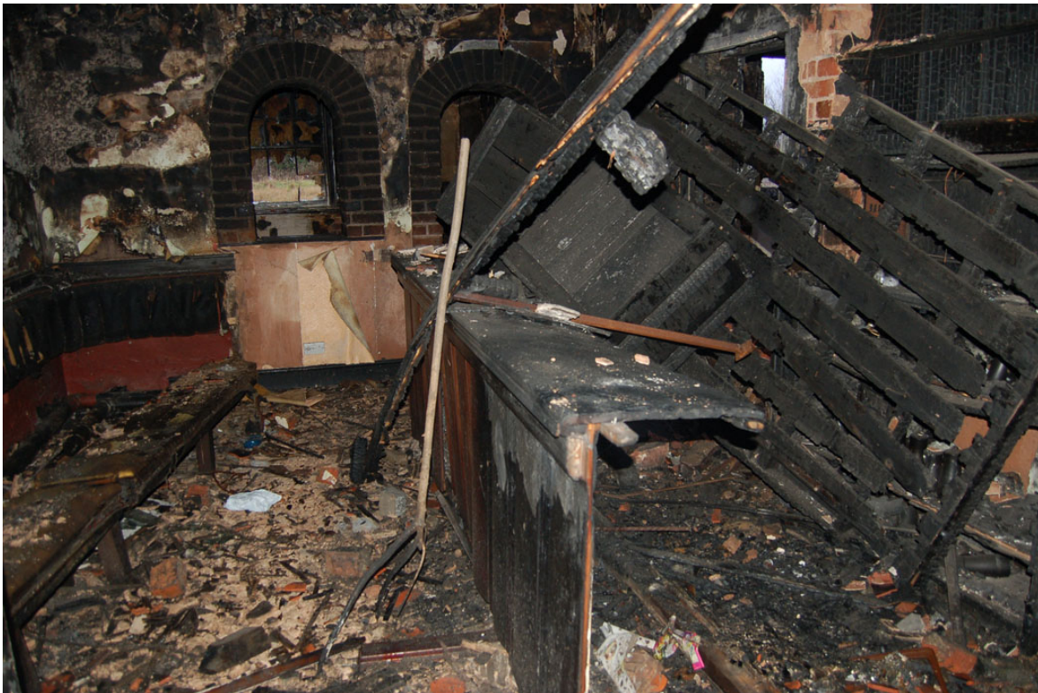
Plate 15: Ground floor interior, Room G2bar area looking north-west.
