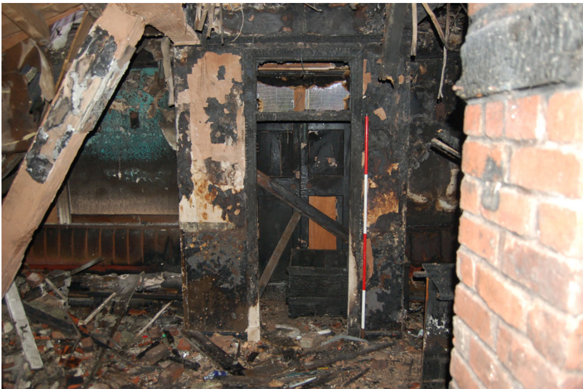
Plate 17: Ground floor interior, Room G2 entrance way.
