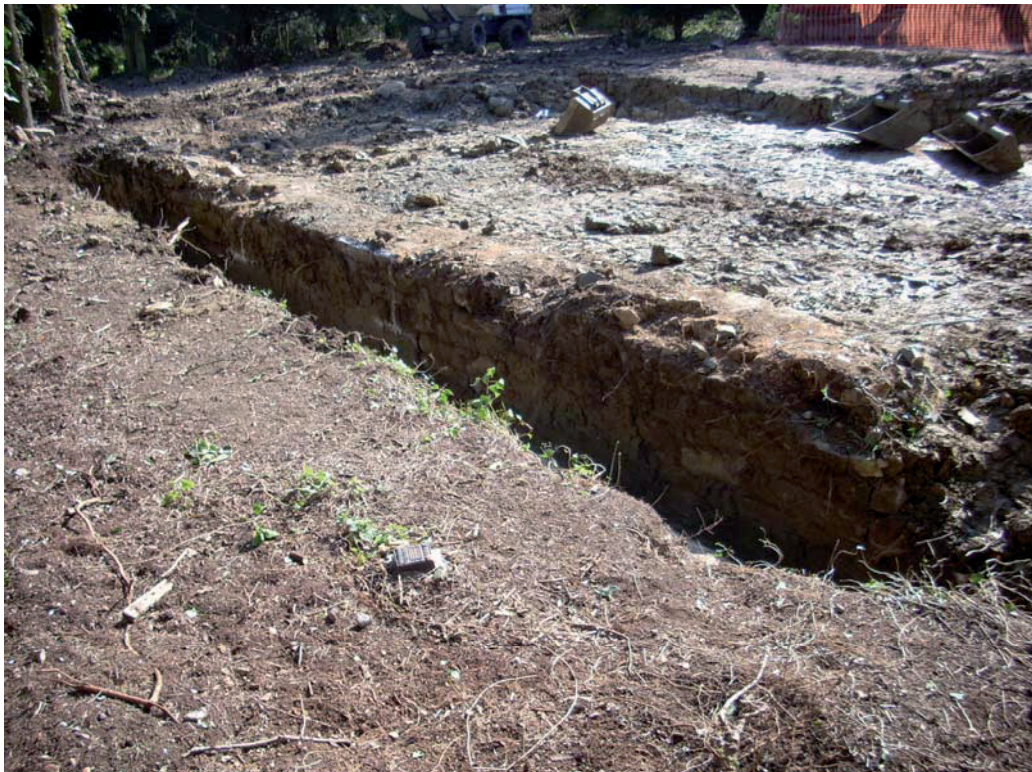
Plate 5: Foundation trench along northwest side of church footprint
