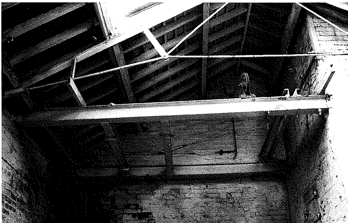
Plate 12. Building D steel framework from the southwest
