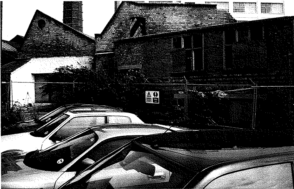
Plate 4. Building B from the southwest
