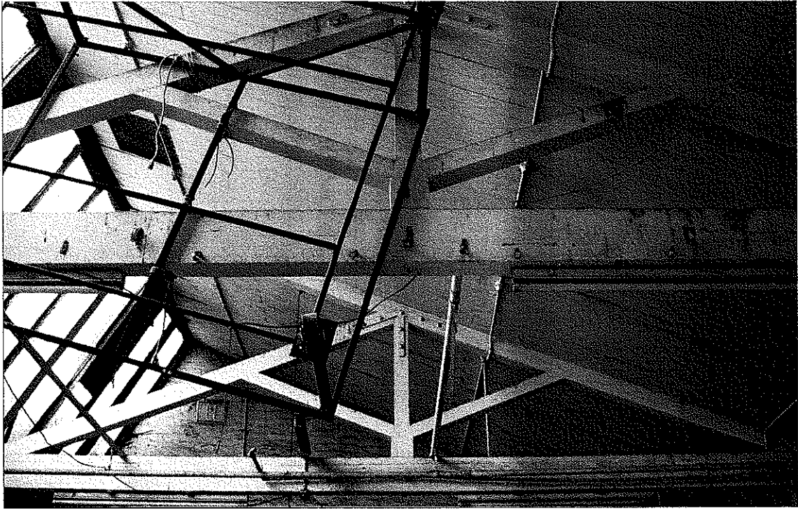
Plate 7. Building C the roof from the southwest
