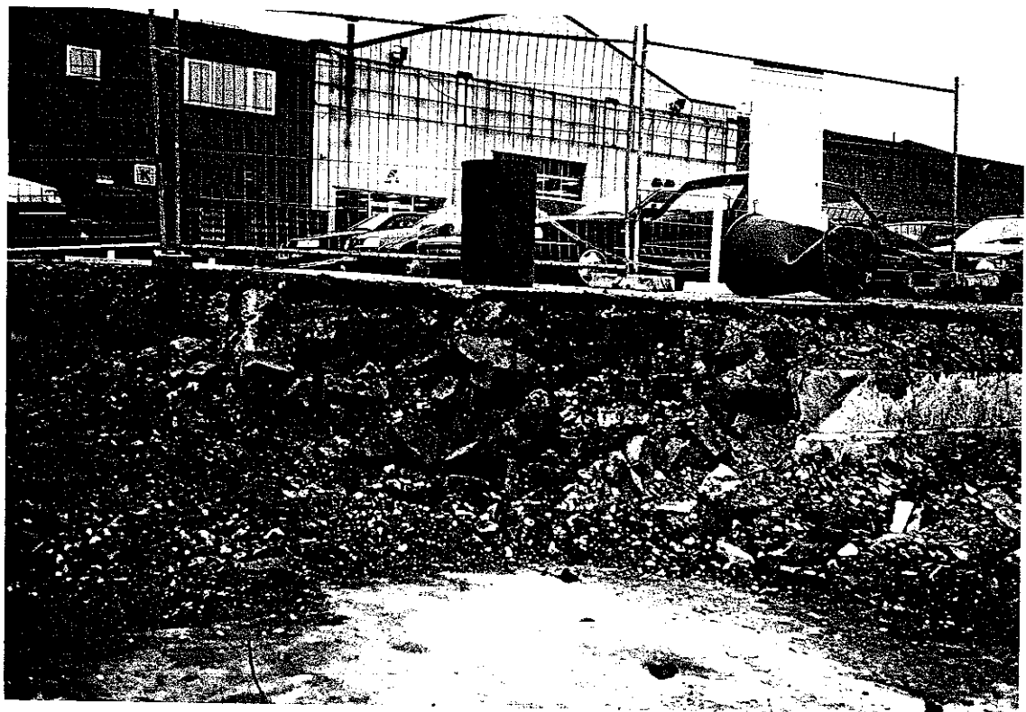
Blocked Cellar Entrance
