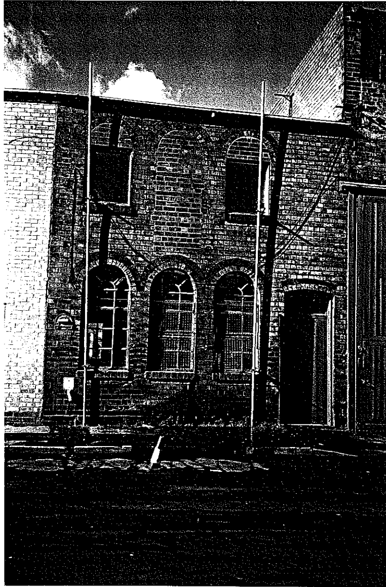
Oxford Street:Demolished Warehouse
