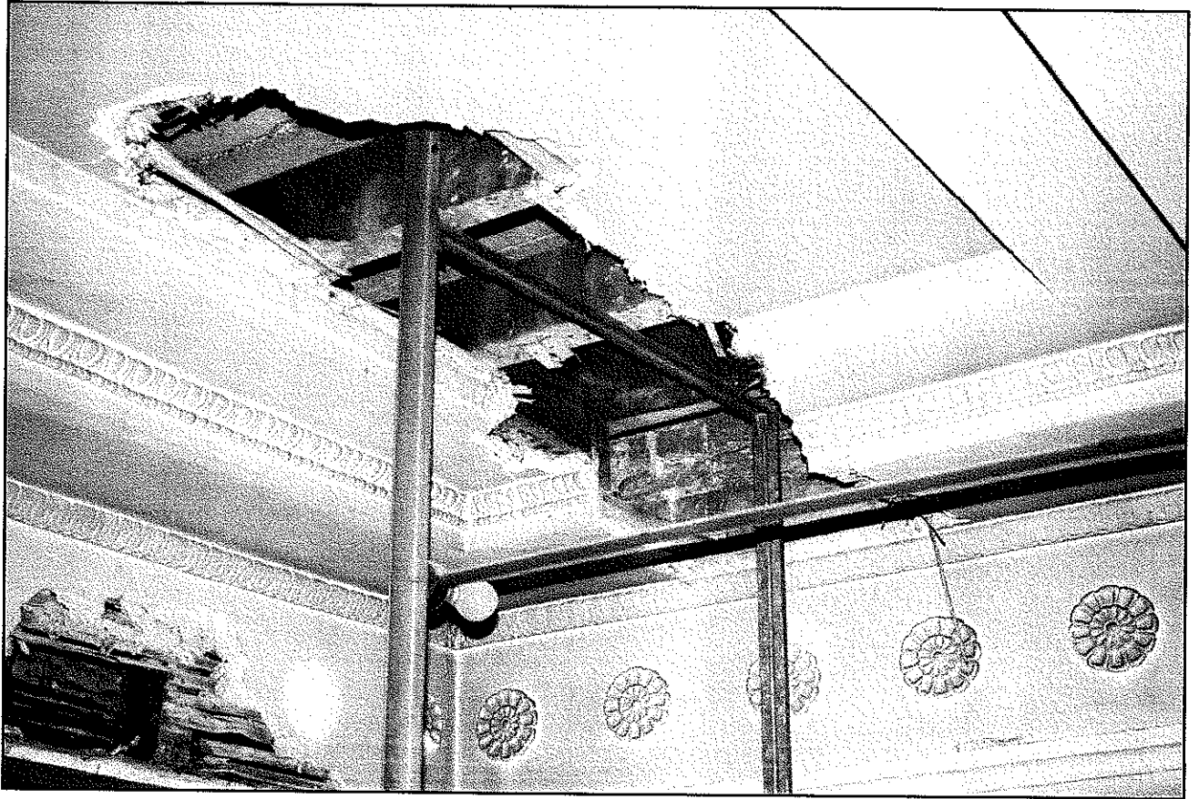
Plate 19: Detail of 1877 plasterwork
