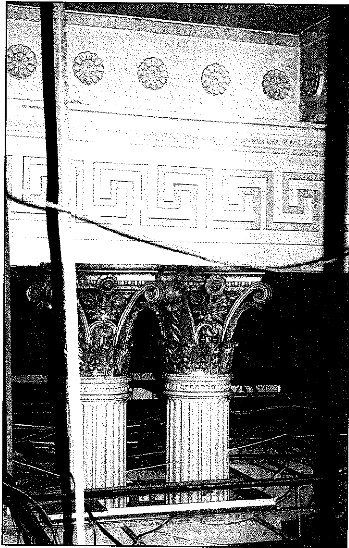
Plate 17: Detail of the 1877 interior
