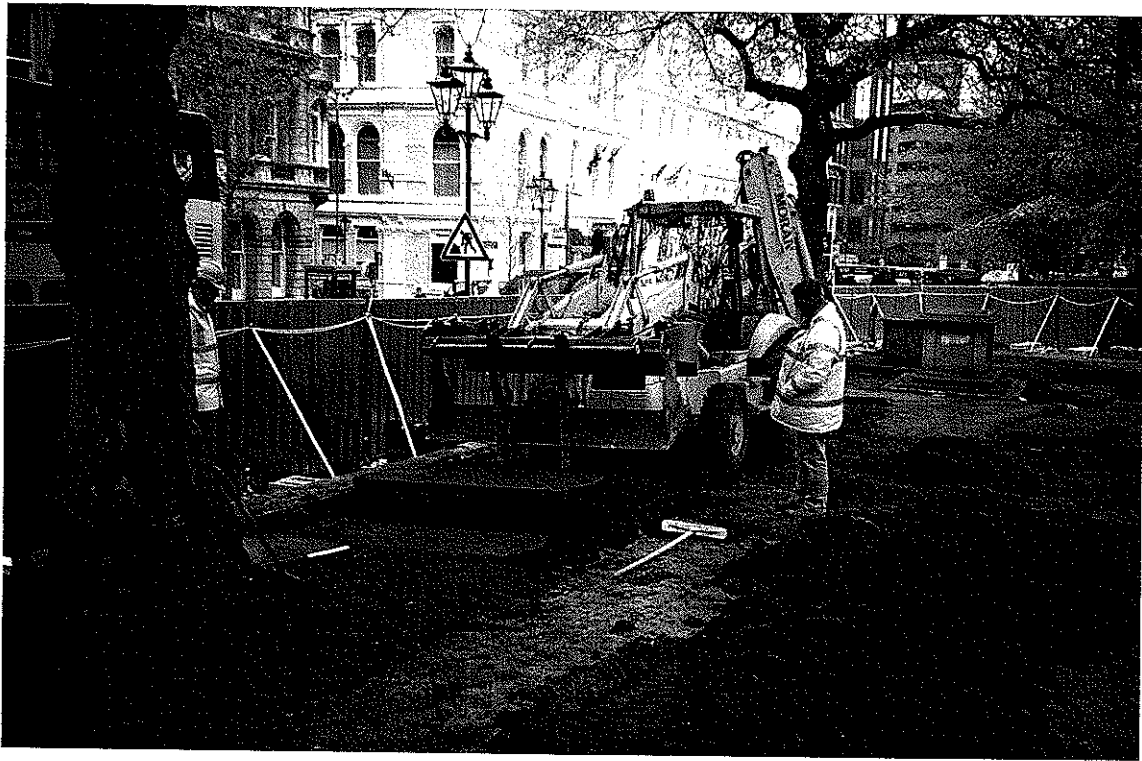
Plate 1 Removal of grave monuments in Area A
