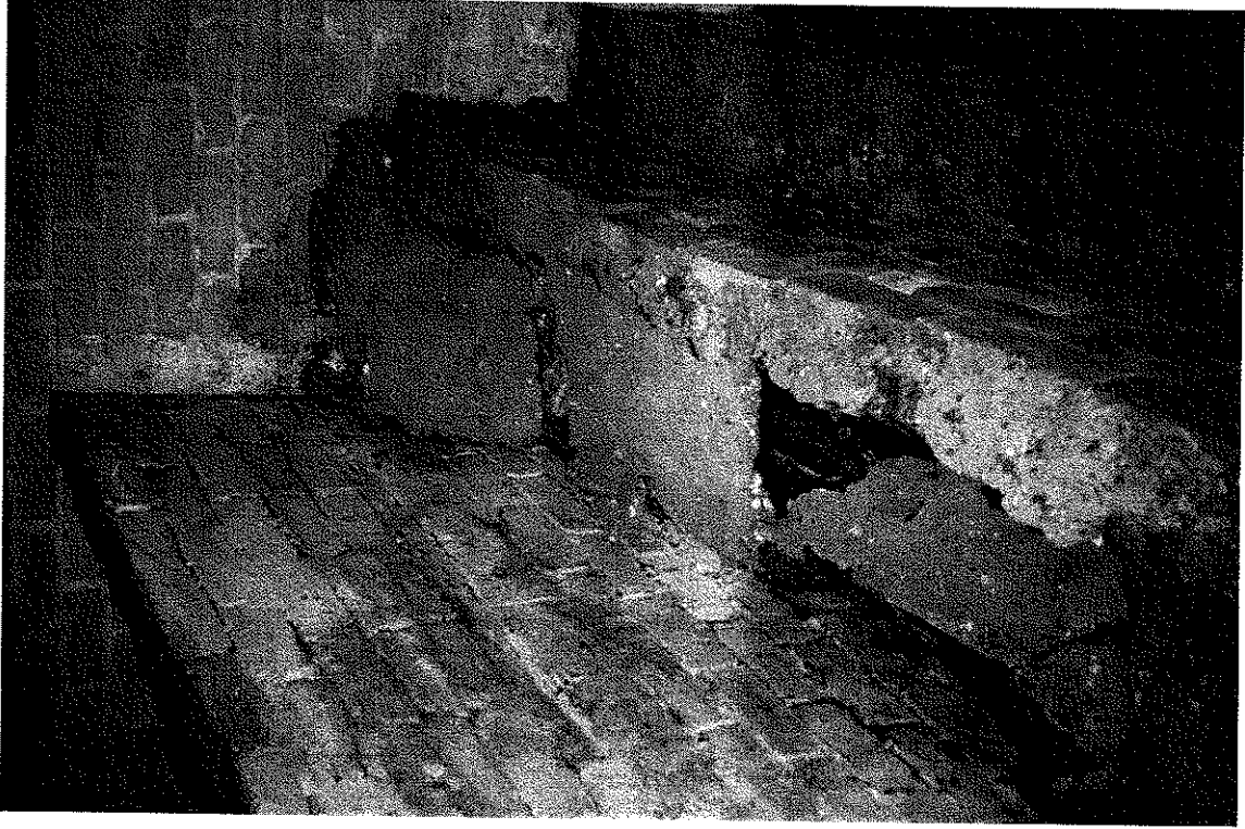
Plate 7 Interior of vault feature 195, Area G1
