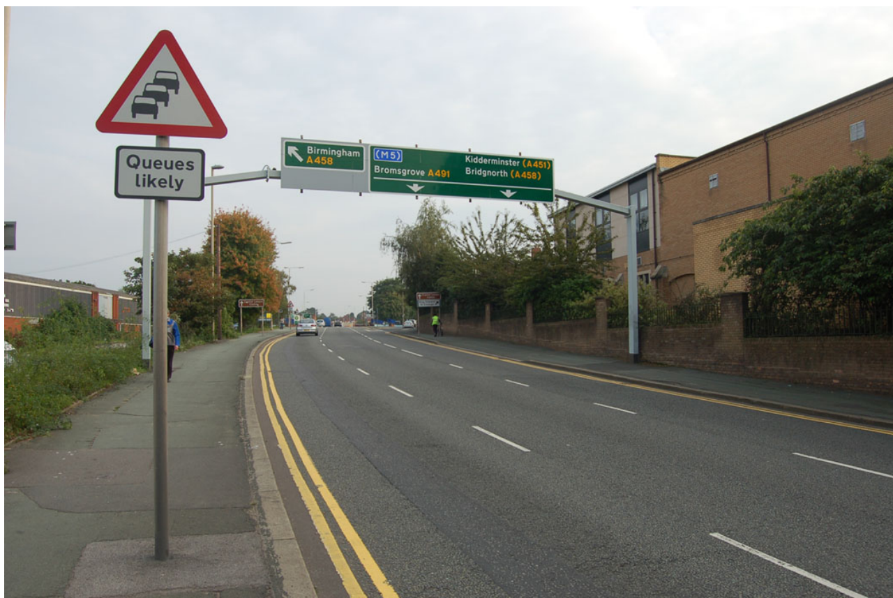
Plate 1: St. John's Road section of ring-road looking south.
