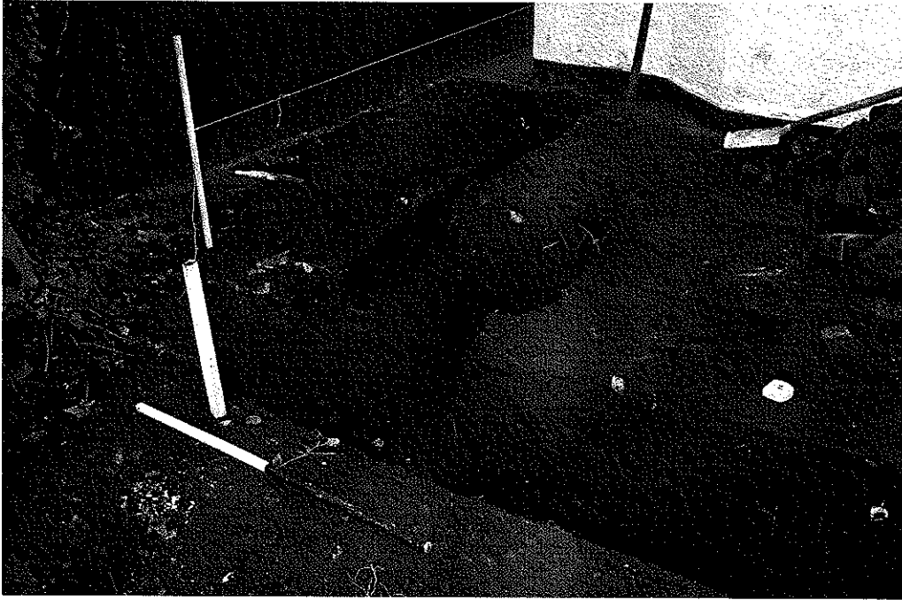
Plate 1 Western Foundation Trench (with Drain)
