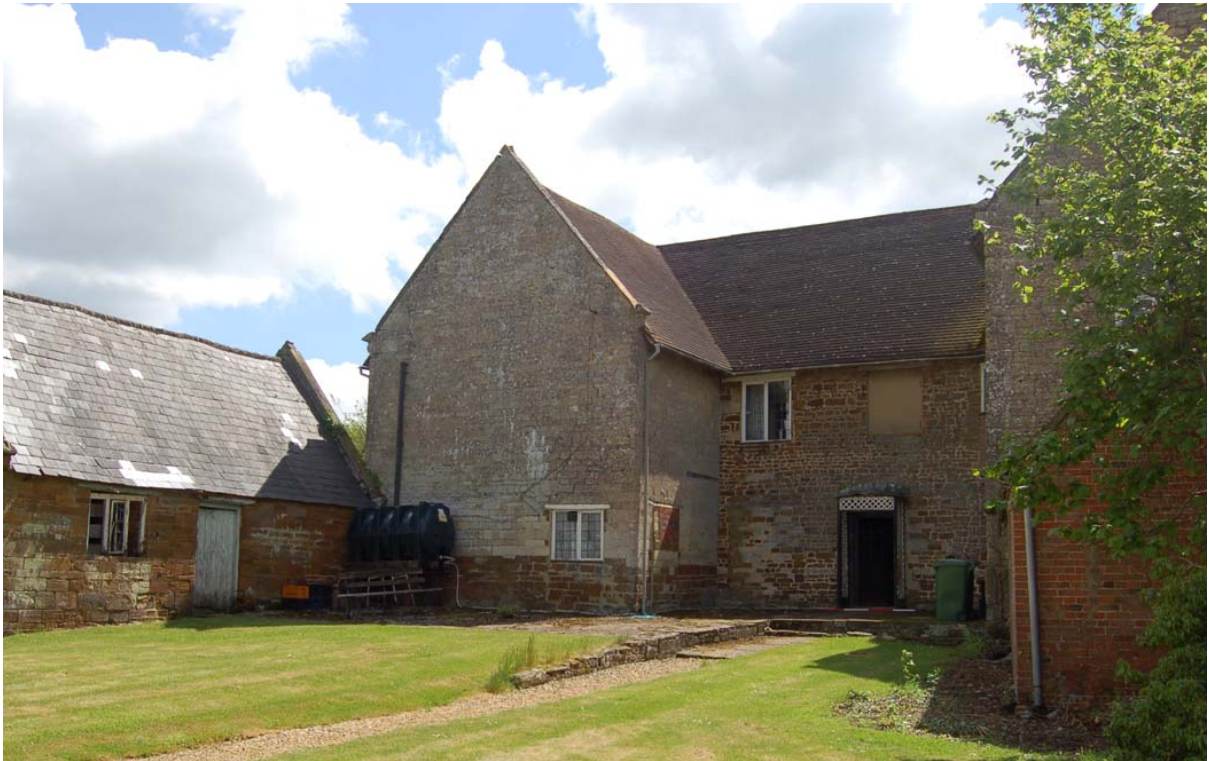
Plate 15: Oblique view of northern extension (windowless pigeon-loft to first floor).
