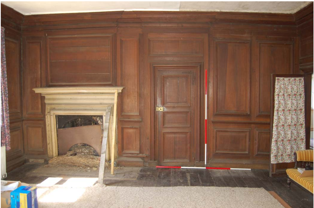
Plate 49: C18th-fielded panelling and bolection fireplace in south wall of Room [1F06].
