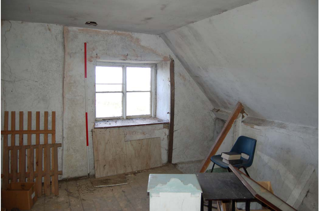
Plate 55: Room [2F01] looking west.
