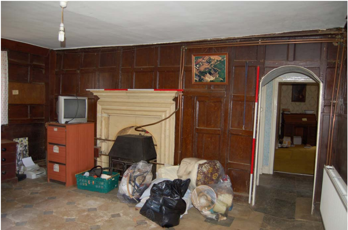
Plate 19: Room [GF06], note bolection fireplace to centre left.
