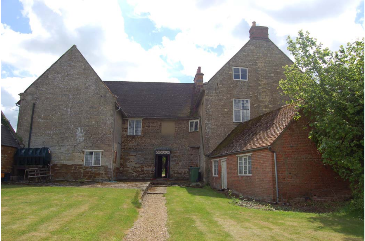
Plate 13: West elevation with late C17th ranges projecting to north and south.
