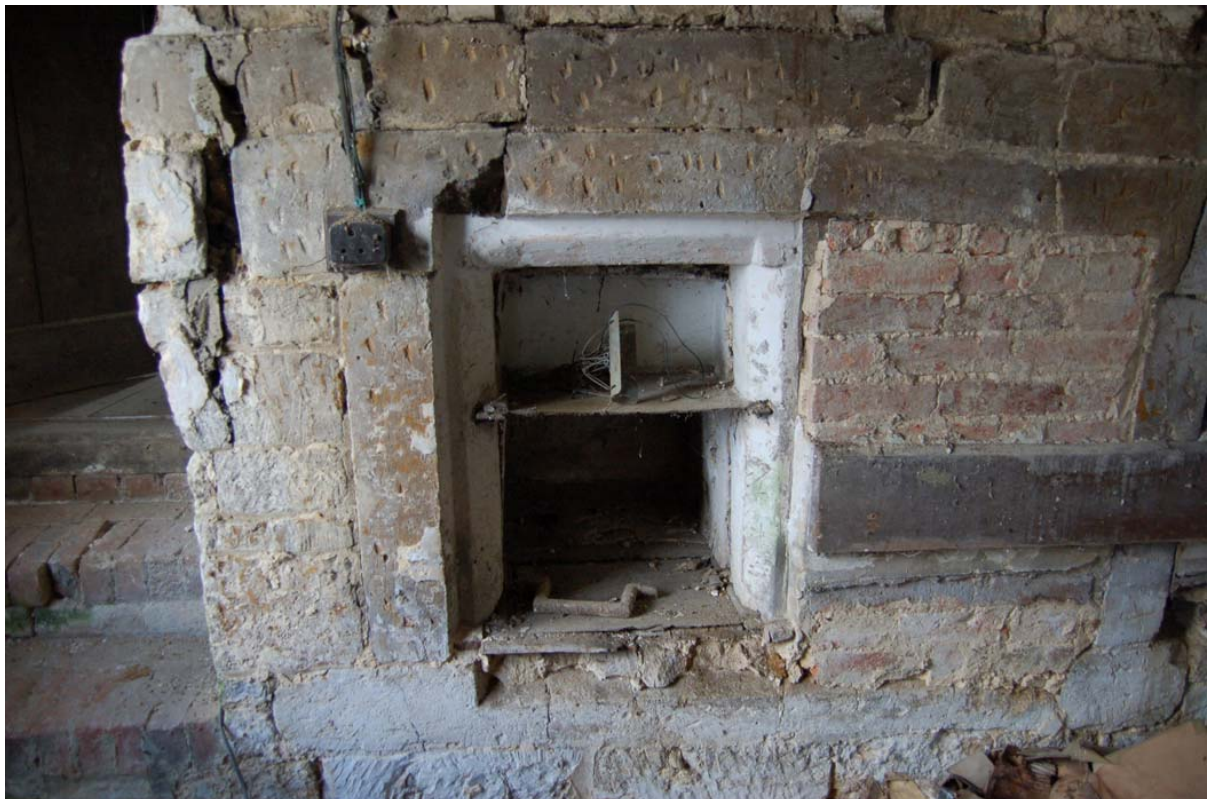
Plate 35: Detail of blocked basement window, reused as cupboard, [GF11].
