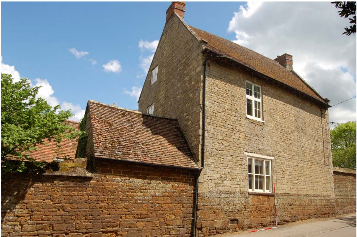
Plate 18: Westhill Farmhouse, south elevation (to High Street).
