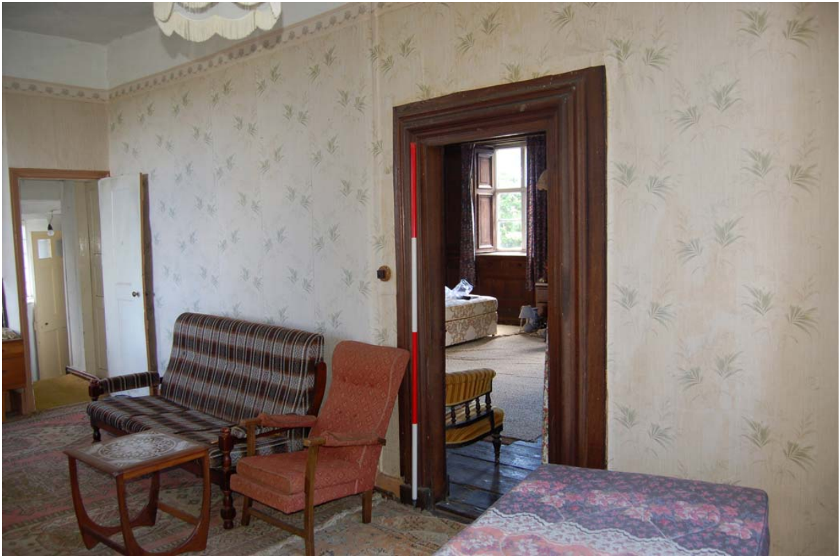
Plate 50: Room [1F07] looking north-east; note bolection doorcase (compare Plate 28).
