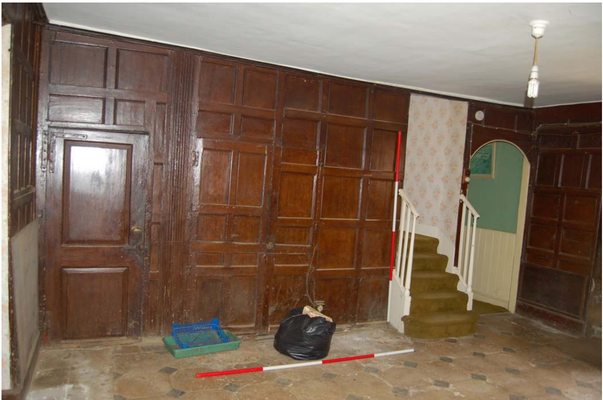
Plate 20: Room [GF06], reset small-square panelling to east wall, note stair to right.
