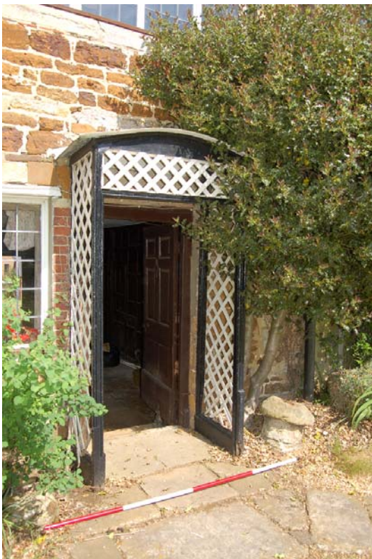
Plate 5: Doorway, east elevation.
