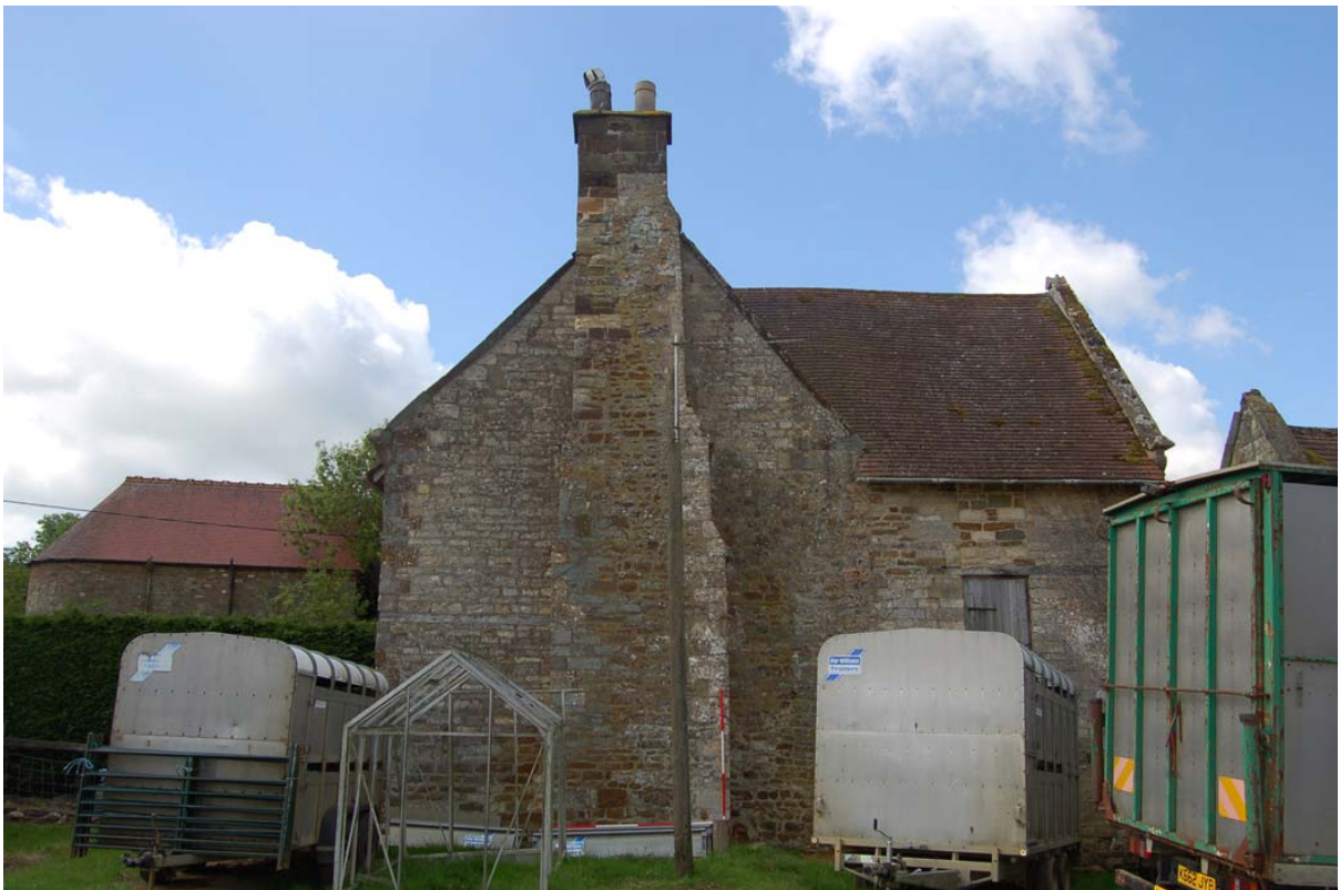
Plate 14: Westhill Farmhouse, north elevation; late C17th extension to right.
