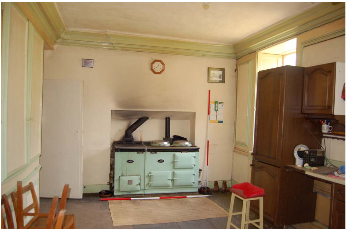
Plate 26: Room [GF07]; general view looking north.
