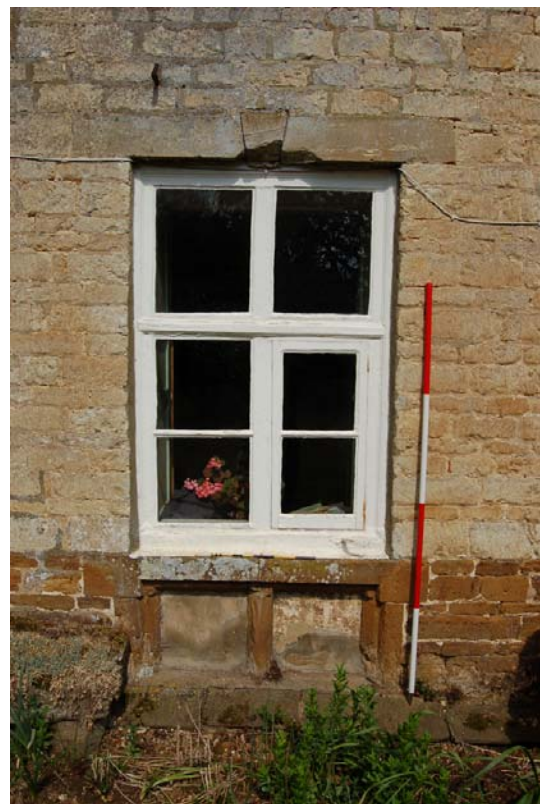
Plate 10: Moulded basement window to late C17th block.
