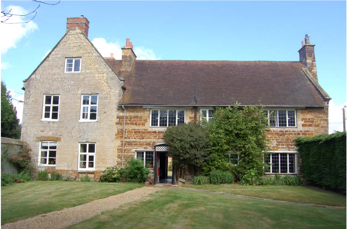
Plate 4: Westhill Farmhouse, east elevation; early C17th block to right, late C17th gable to left.
