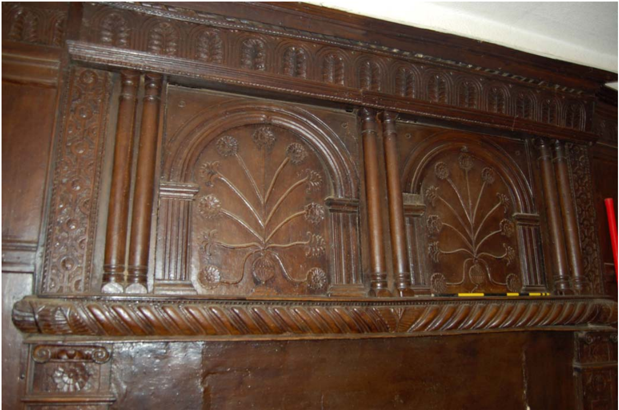
Plate 45: Room [1F05]; detail of Jacobean overmantle.
