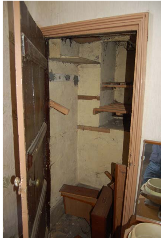
Plate 53: Room [1F07]; stair head.
