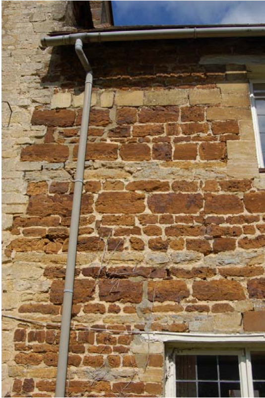
Plate 7: Phase break in east elevation.
