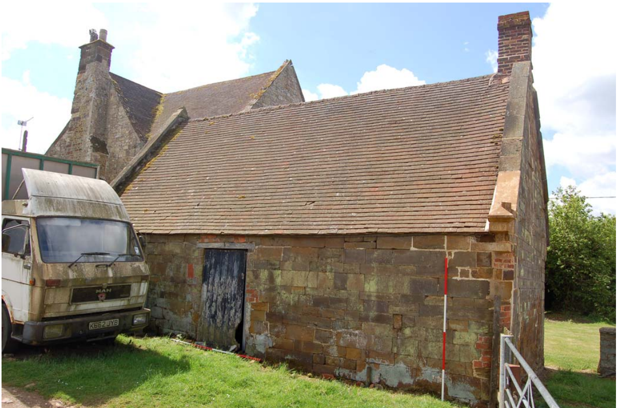
Plate 58: Outbuilding to north-west of farmhouse; looking south-east.
