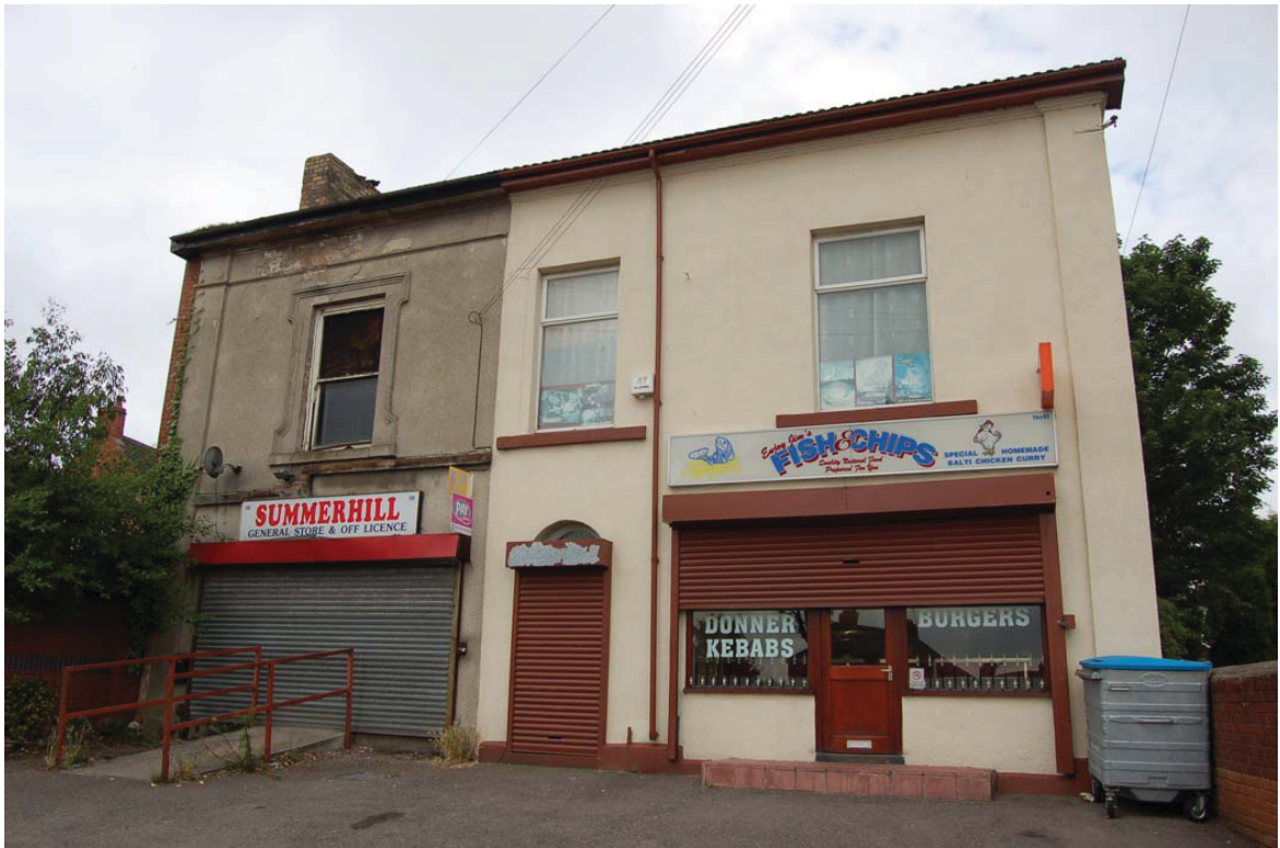
Plate 36: Nos. 39/41 Summerhill Road, street elevation
