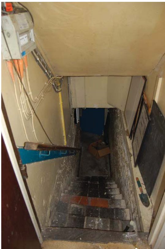
Plate 24: Stair to basement [B3].
