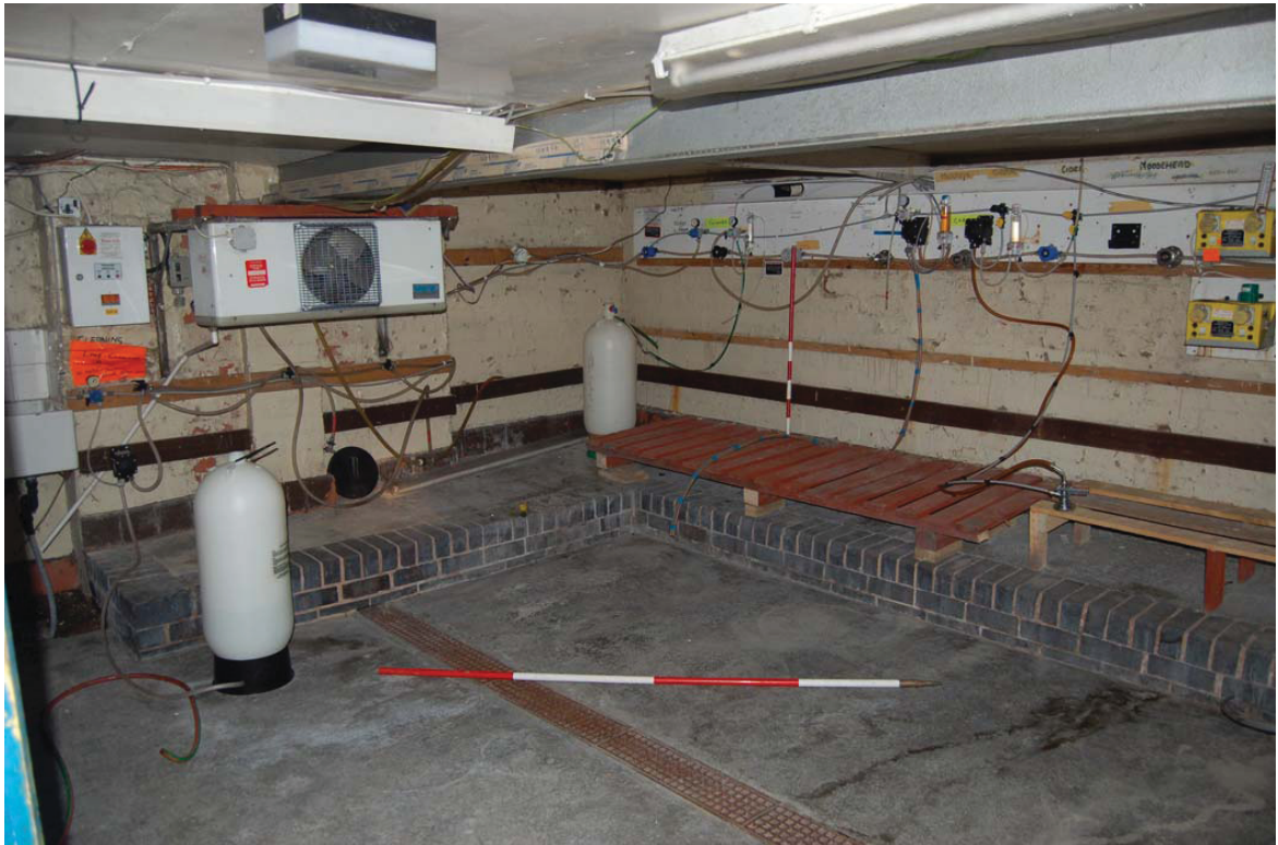
Plate 15: Basement Room [B2] looking north-east.
