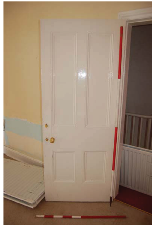
Plate 32: Room [F2]; 4-panel door.
