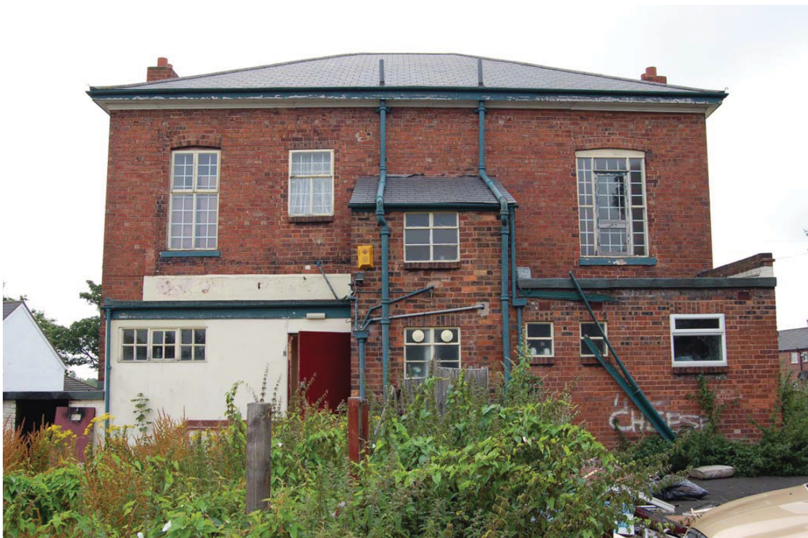
Plate 8: West (rear) elevation, note later extensions to GF level.
