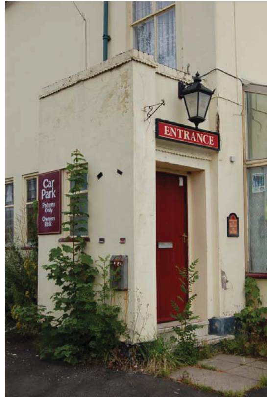
Plate 7: Post-1938 entrance porch (S).
