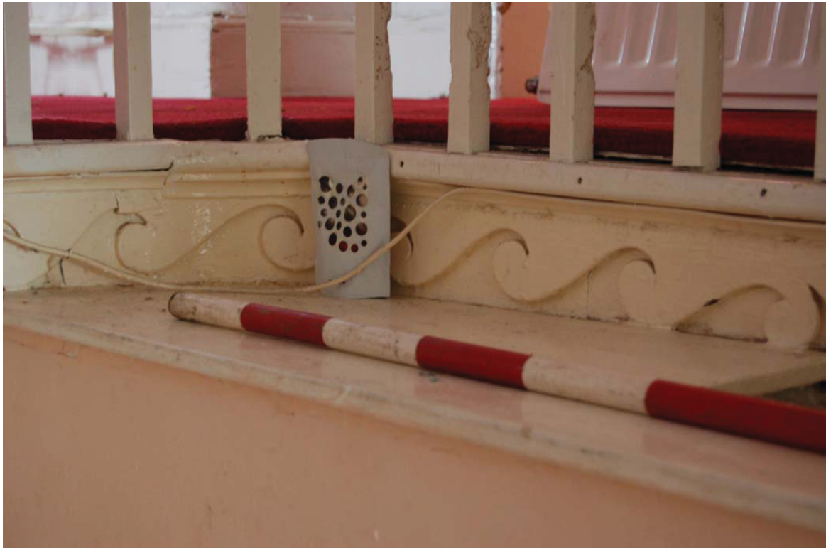
Plate 26: Main stair: detail of running wave decoration to string.
