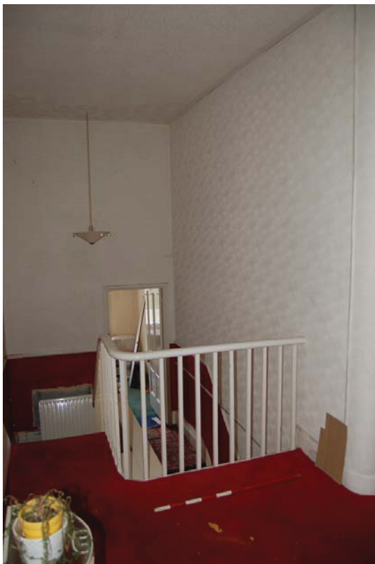
Plate 27: Landing [F1] looking west.
