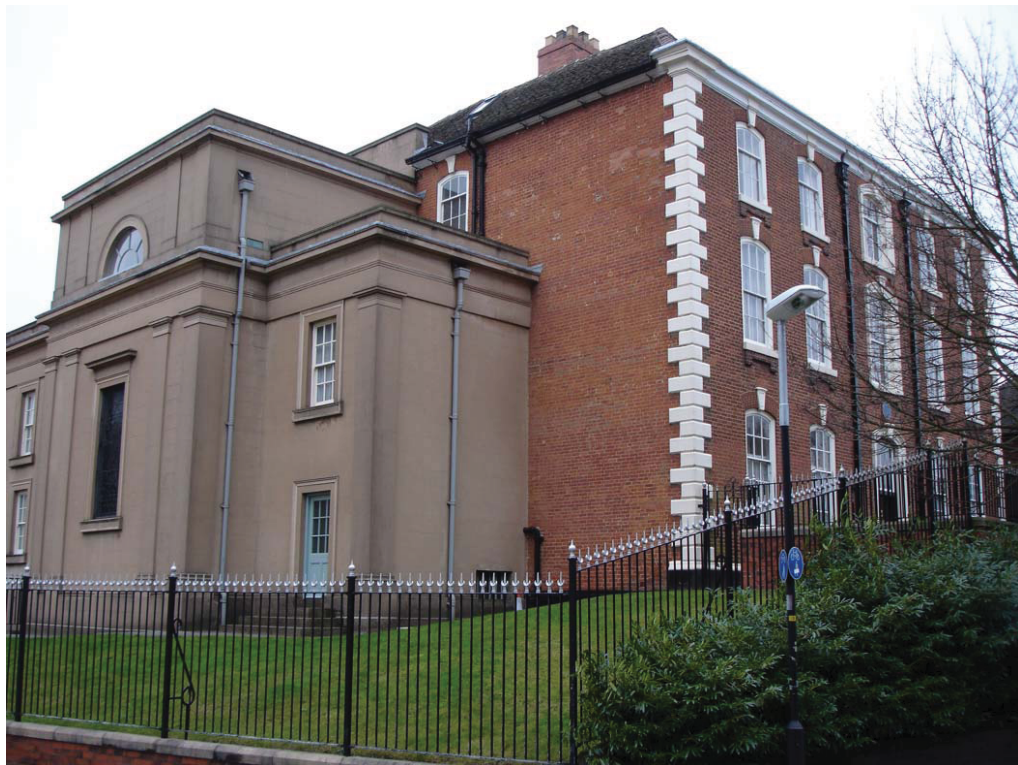
Plate 8: Giffard House (BCSMR 491 , right) with adjoining Catholic Church of St Peter and St Paul (BCSMR 480 , left), both Grade II* Listed buildings.
