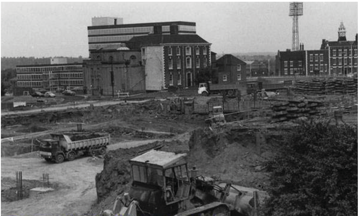
(b) General view looking north during construction of Wolverhampton Civic Centre, 1975 (WALS P/5936); Molineux House to right, Giffard House and Church of St Peter and St Paul to centre.
