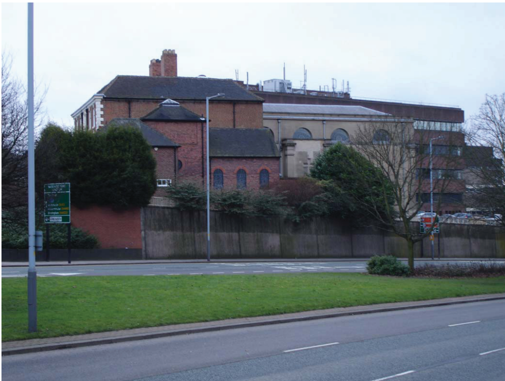
Plate 13: Long view of Giffard House (BCSMR 480) and Catholic Church of St Peter and St Paul (BCSMR 480) from north side of ring road.
