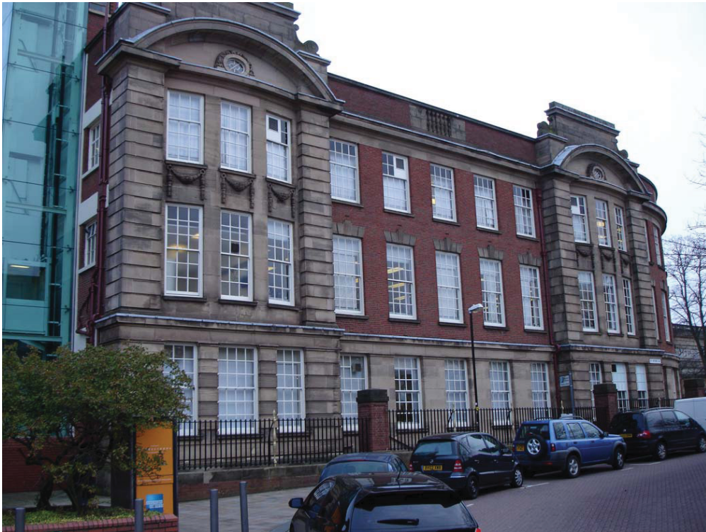
Plate 12: University buildings (formerly W'ton and Staffs. Technical College, BCSMR 13218), 1932.
