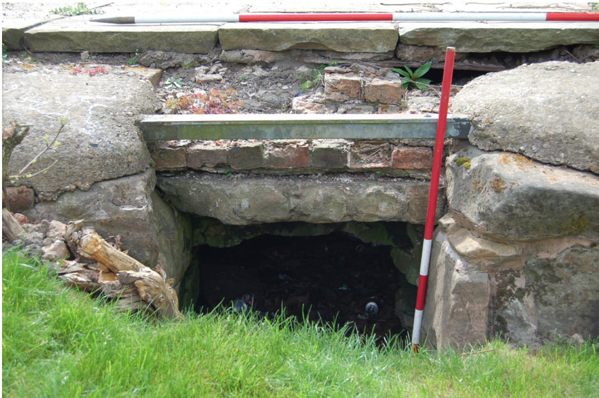
Plate 12: Culvert [C], northern opening.
