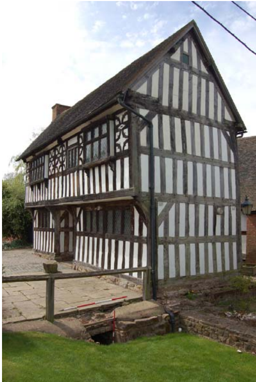
Plate 10: Culvert [C]; context shot looking south-west.
