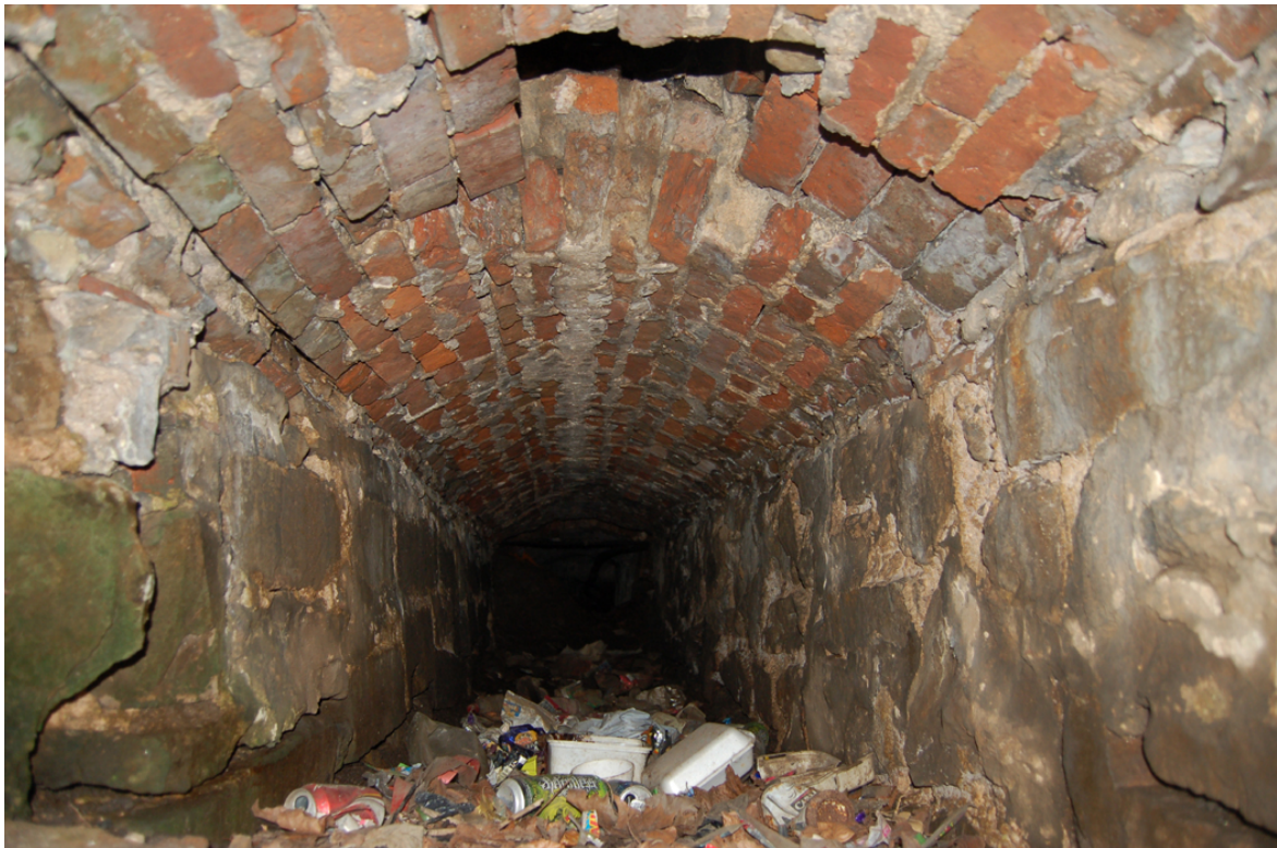
Plate 13: Culvert [C], interior looking south.
