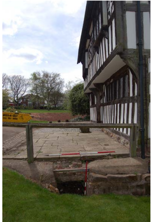
Plate 11: Culvert [C], north end.
