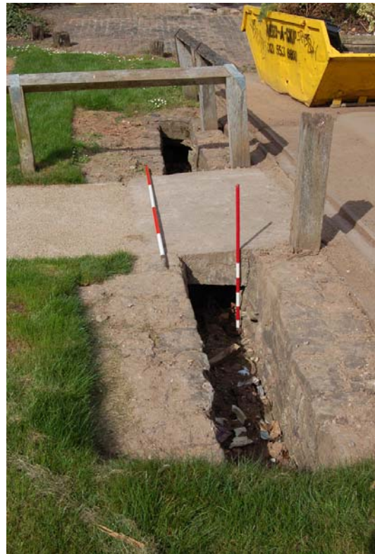
Plate 7: Open section of Culvert [B] looking west.
