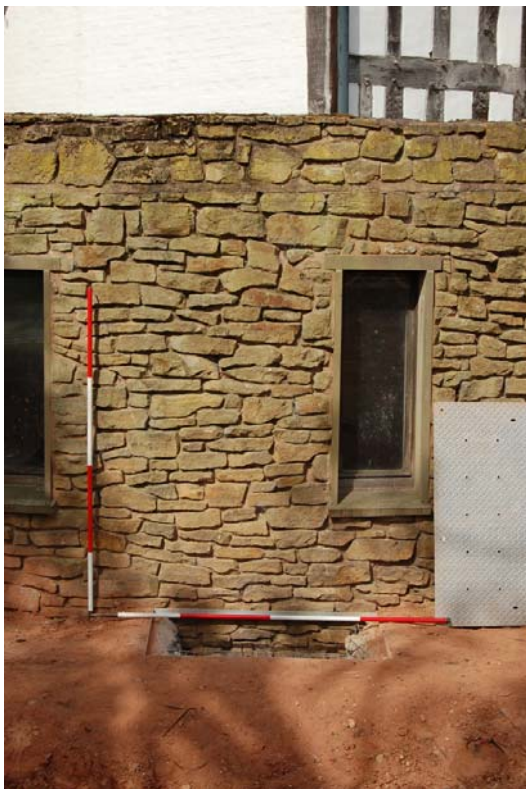
Plate 2: Access to Culvert [A] adjacent to modern extension.
