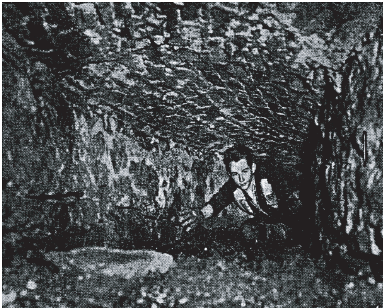
(b) Interior view of Culvert [C] during renovation work (Birmingham Mail 02/05/1957)
