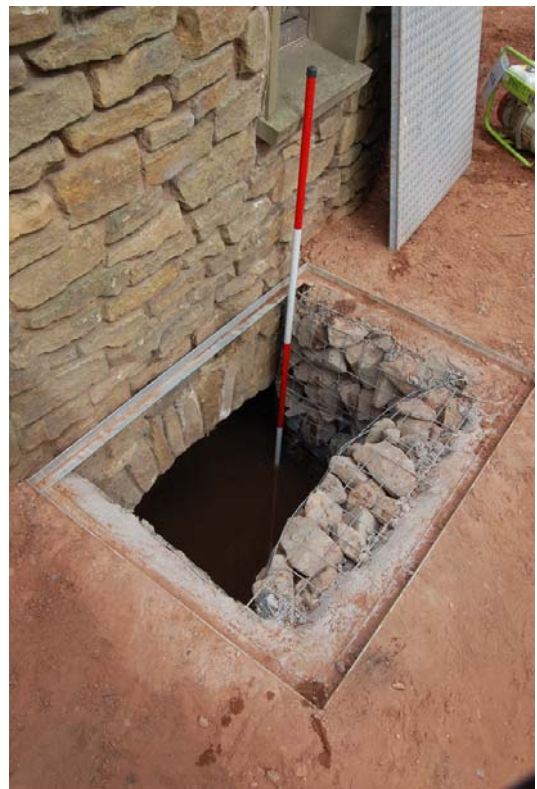
Plate 3: Access hatch to Culvert [A]
