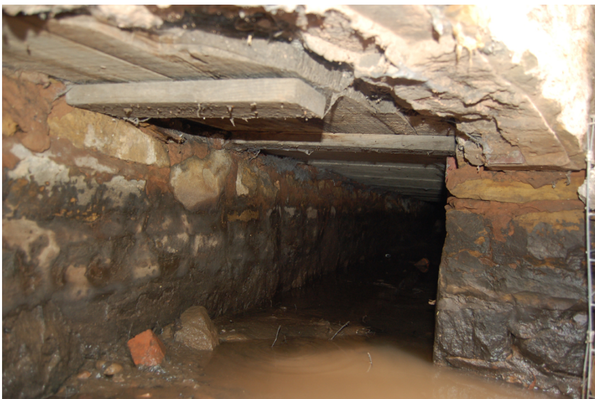
Plate 5: Culvert [A]; interior looking north-east; note high water mark on walls.
