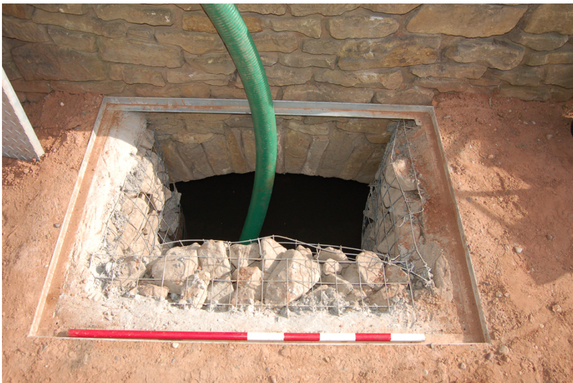
Plate 4: Water-filled terminal to Culvert [A].
