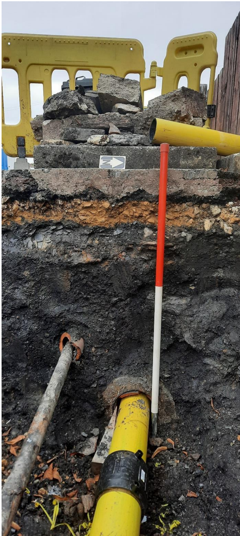
Figure 9: Detail of the east facing section of Trench 14
