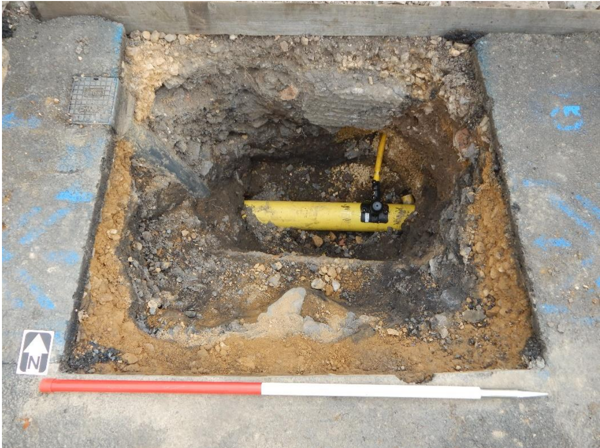
Figure 7: View of Trench 7 at 36 Lanercost Gardens, facing north
