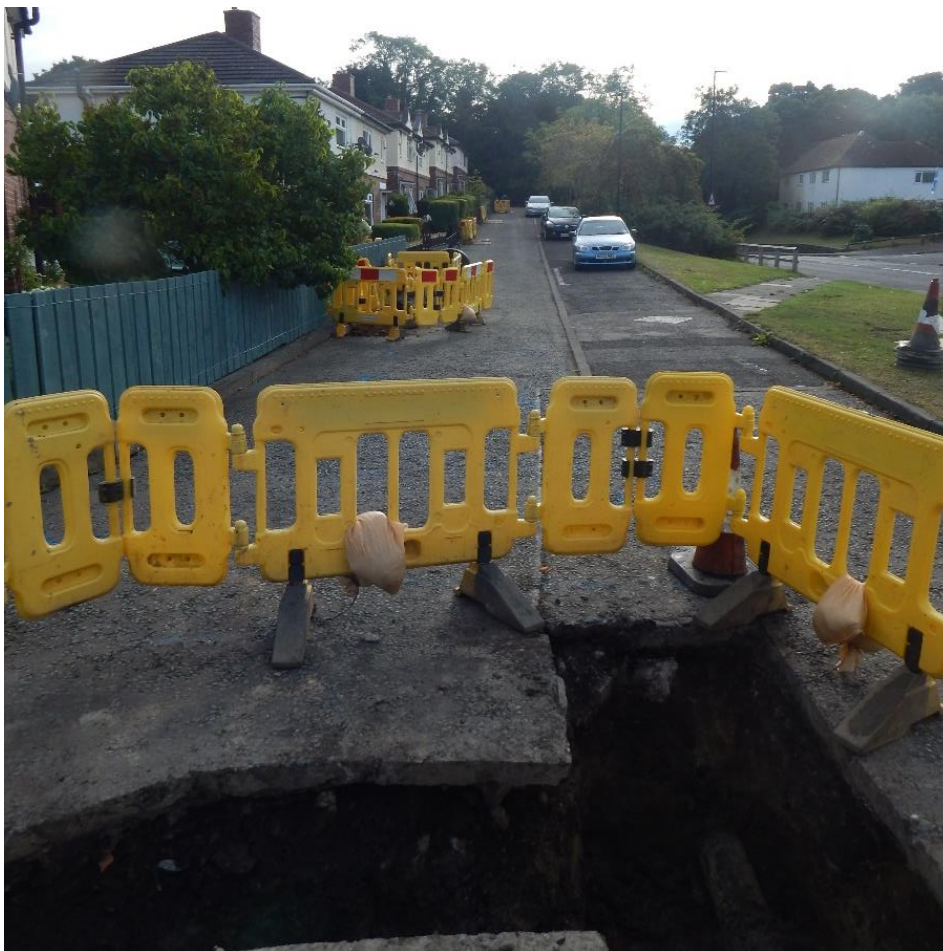
Figure 6: View across Lanercost Gardens, facing east
