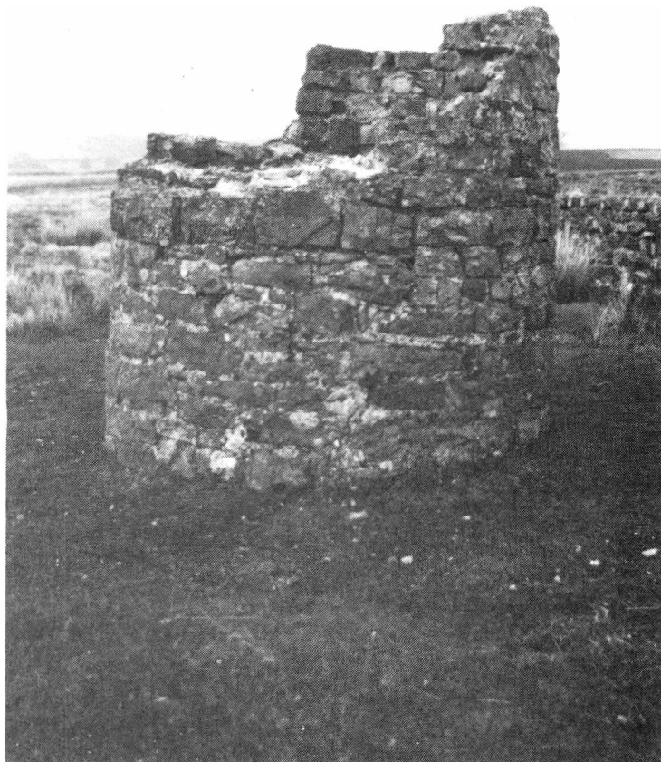
Plate 6. Coal workings (stone chimney for ventilation shaft), Stiddlehill (site K4).
