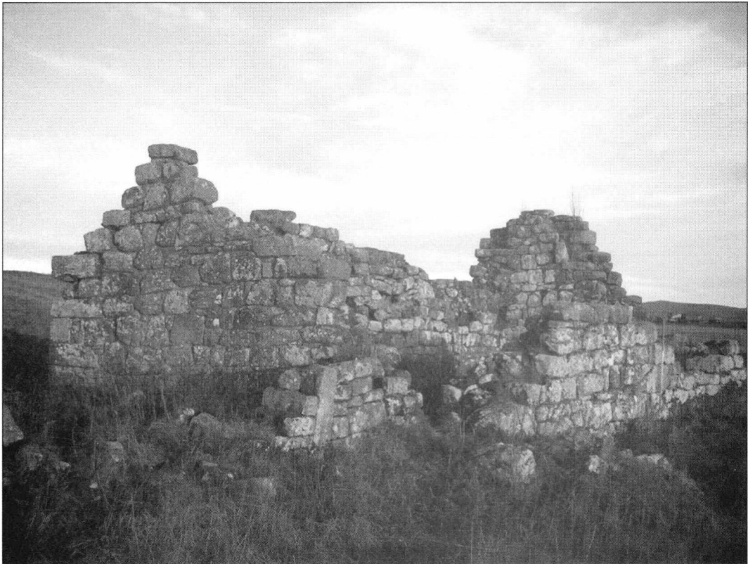
Fig. 6. Ironhouse Bastle, looking north-east
