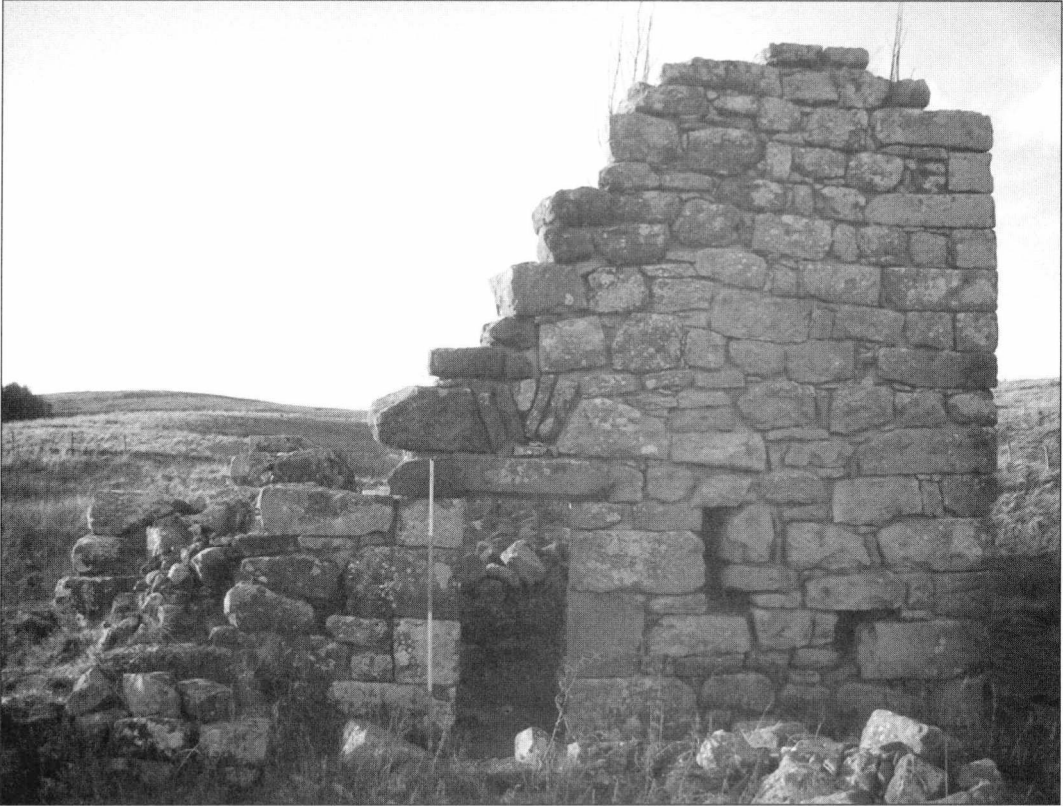
Fig. 5. The eastern gable-end and byre door of Ironhouse Bastle
