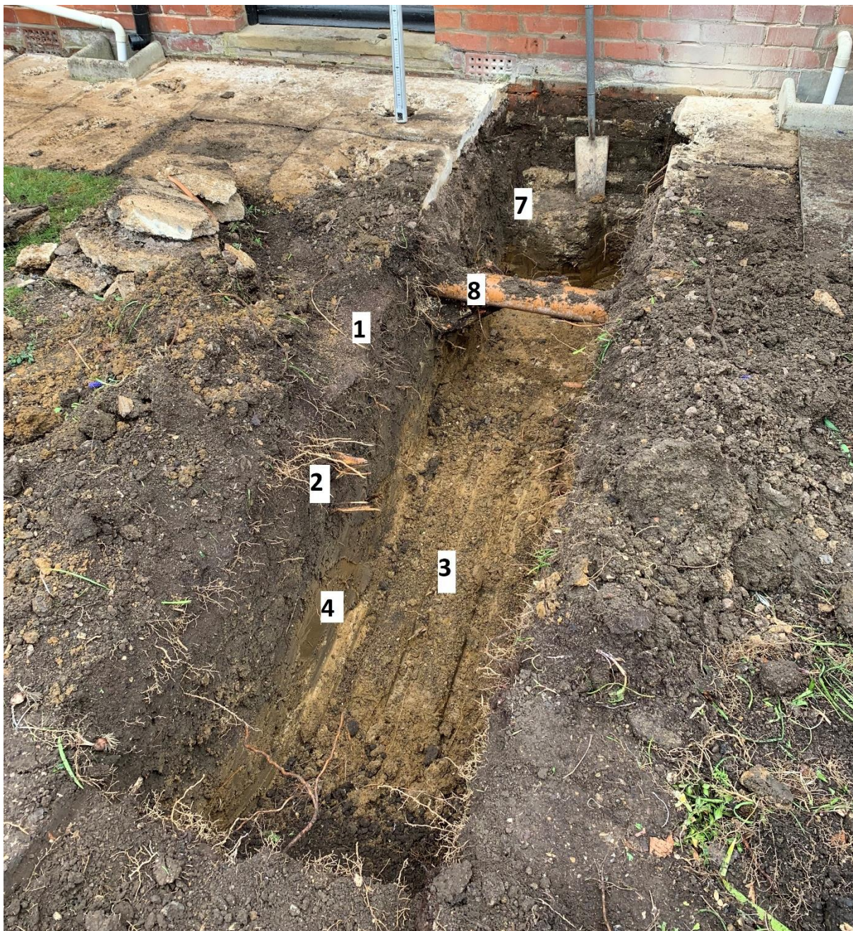
Figure 5: The north foundation trench, also looking west towards the house.
