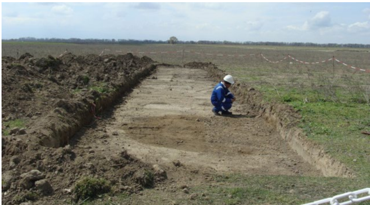
Figure 2. General view of the excavation. View to west.
