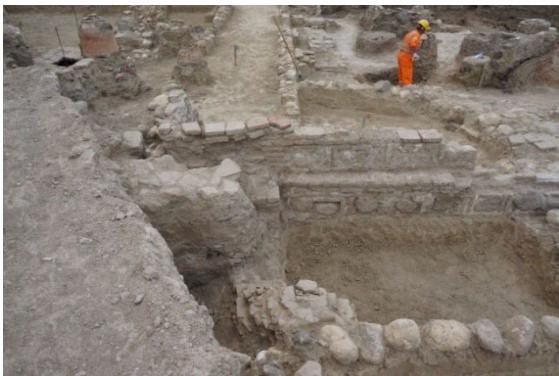
Figure 11: North entrance tower, 2017 excavation, looking west. Brick and stone decorated wall on the west of the entrance, ephemeral remains of east wall. North wall is in the distance.
