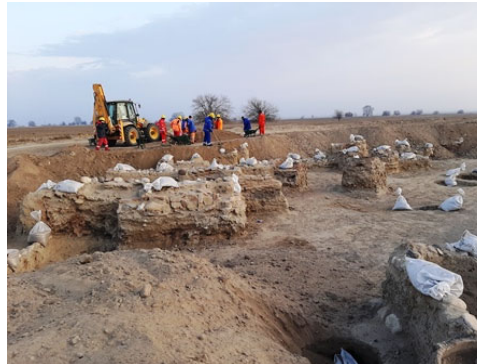
Photo 229h. Conservation activities in west
