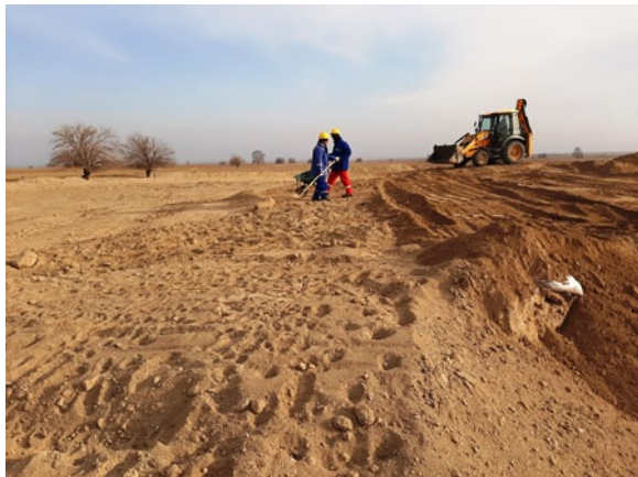
Photo 229k. Levelling upper soil layer
