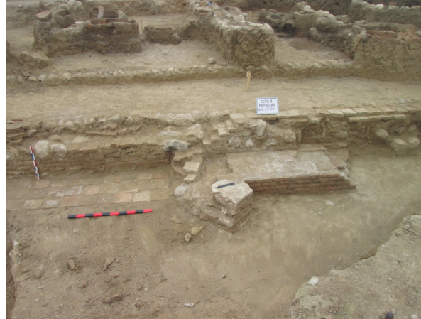
Photo 115. U38. Castle wall showing two phases of external brickwork and foundation line of stones to rear of rampart. Small outer projection (possible turret). View to east.
