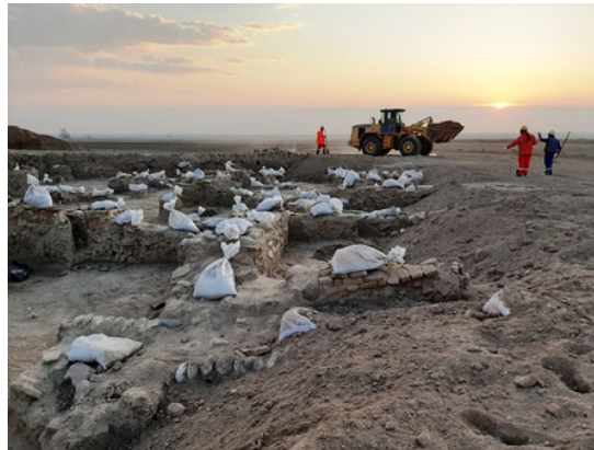
Photo 229 ii. Conservation work in southwest
