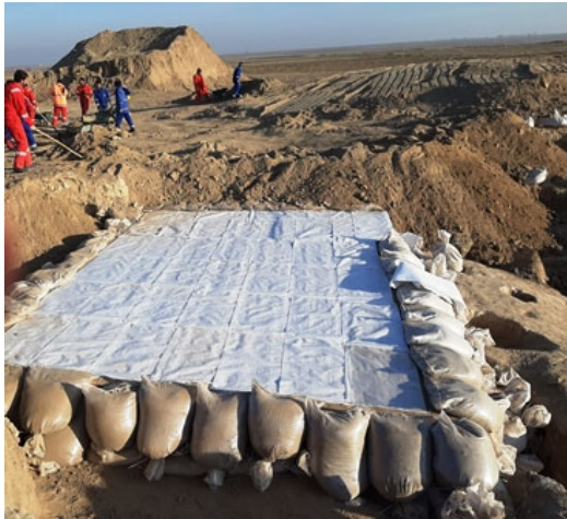
Photo 229 ee. Final completion of kiln conservation
