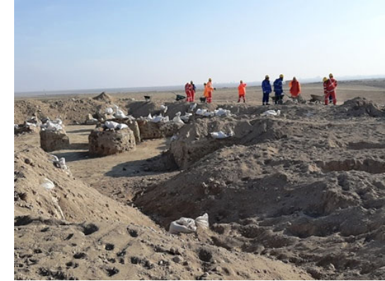
Photo 229c. Conservation work in southeast
