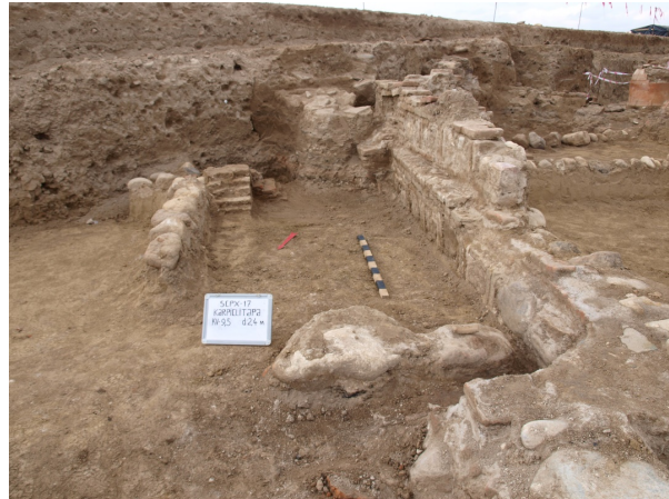
Photo 112. U9. Tower 2, entrance to interior of castle through centre of tower. View to south
