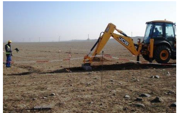
Photo 6. Trial pit excavation by machine.
