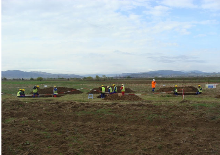
Photo 8. Excavation site. View to south.
