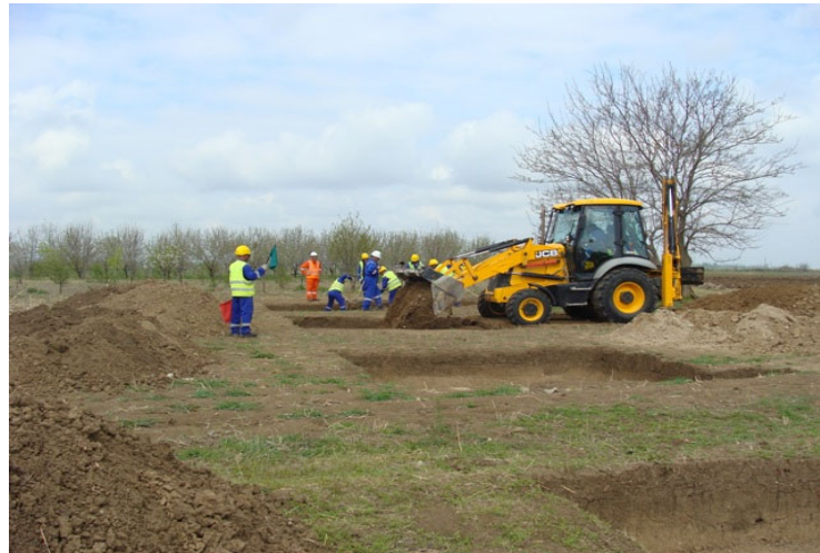
Photo 7. Backfilling excavation.
