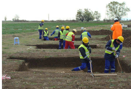
Photo 11. Excavation in process
